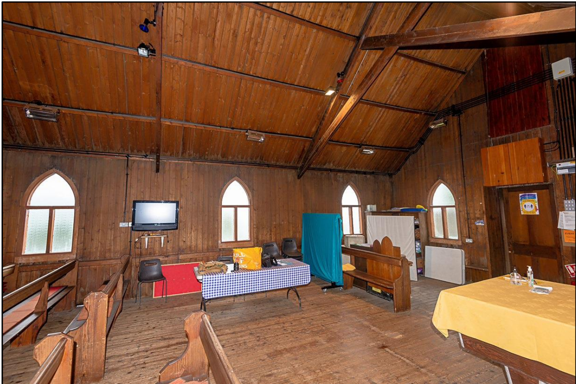
Nave looking Southwest
