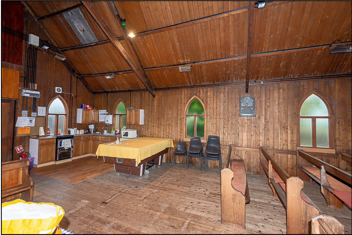
Nave looking Northwest
