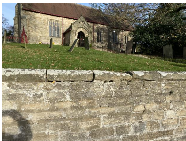
Image E & F: Lifting coping stones to Southern boundary wall
