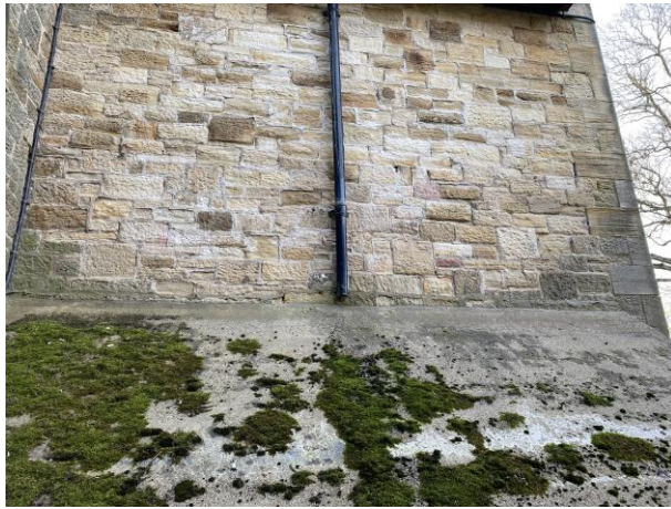
Image A: In situ concrete roof to Boiler house.
