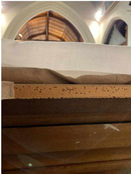
Image H, I & J: Evidence of woodworm
