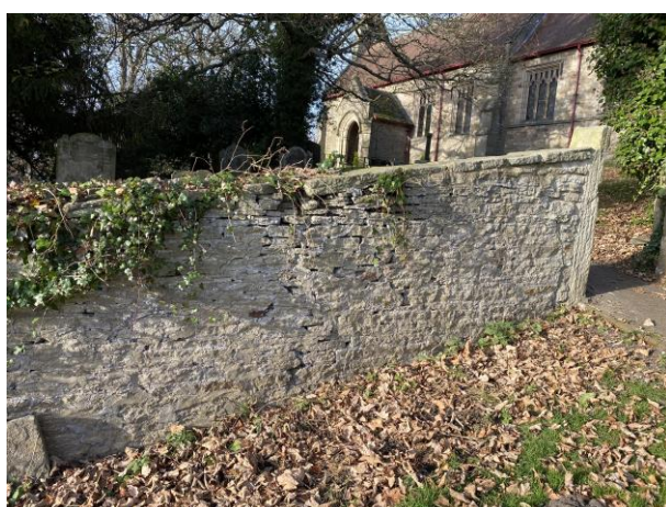
Image C & D: Boundary walls requiring attention
