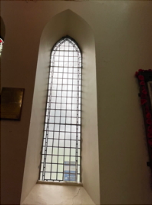
Window 1 Leaded, plain glass, good condition
