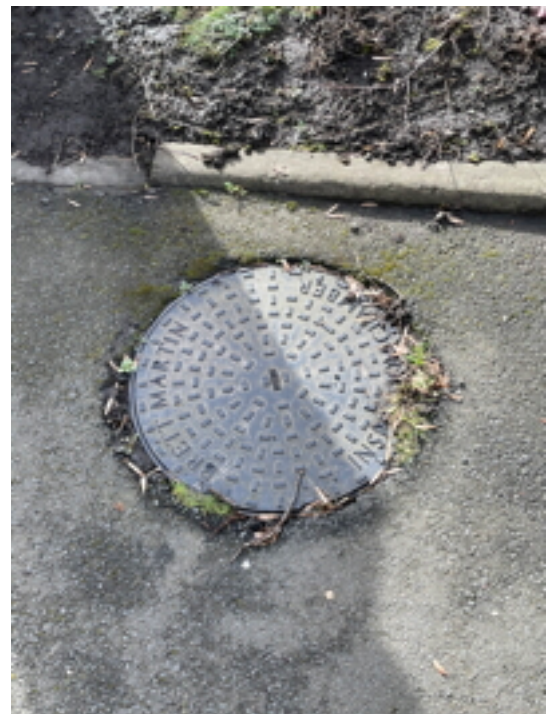
Modern Inspection Chamber
