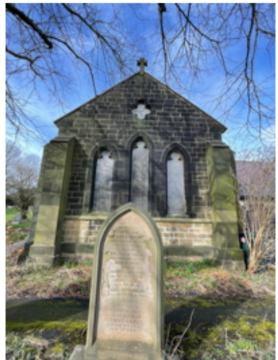
Chancel East Wall
