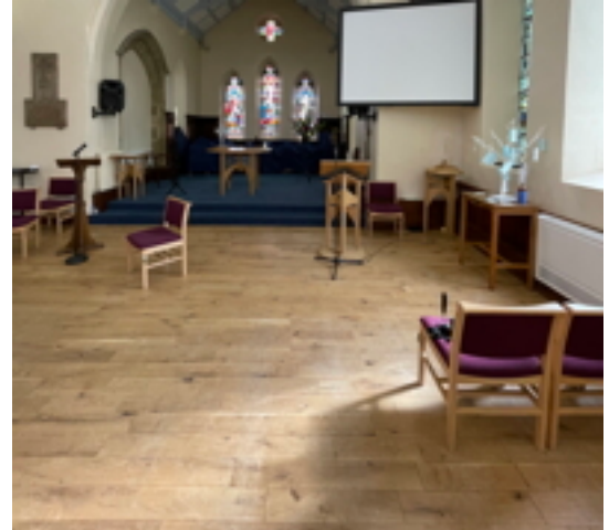
Oak Flooring to Nave
