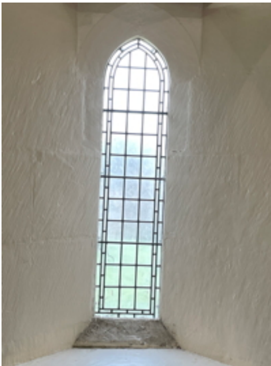
Window 17 North Aisle, single lancet, plain.
