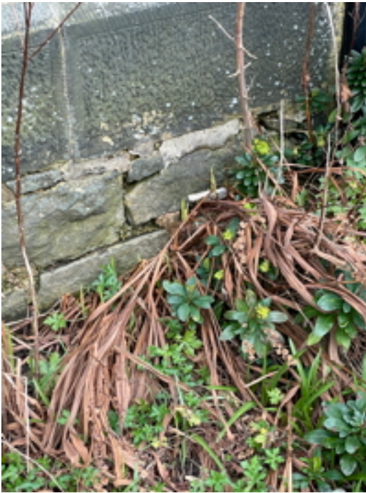
Nave South Wall High Ground Level
