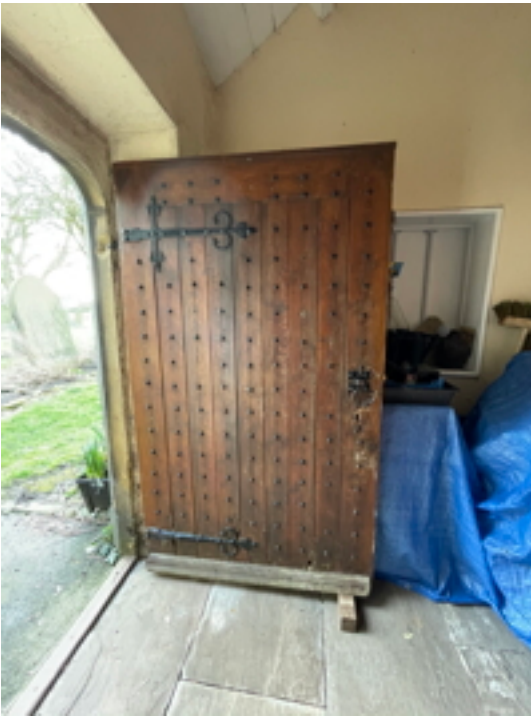
Porch Door, heavy boarded door with iron fittings and studs
