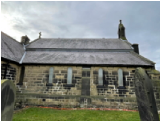
North Aisle Roof
