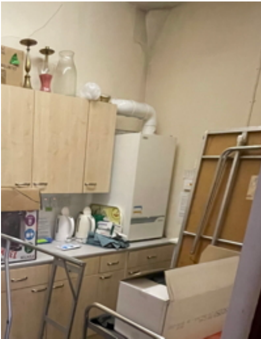
Boiler in Kitchen
