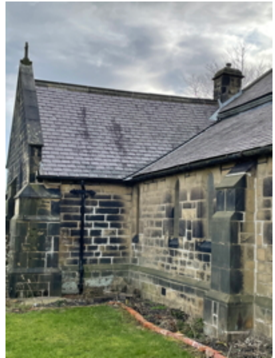
North Transept West Roof
