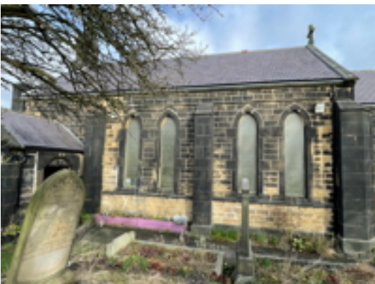
Nave South Wall
