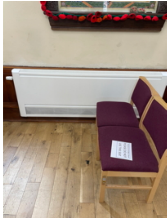
Low Surface Temperature Radiator in Nave
