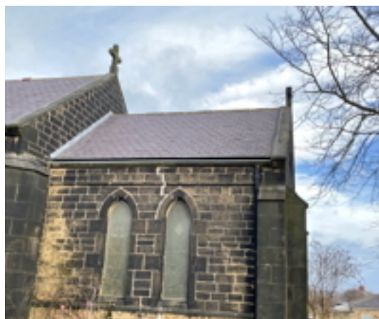
Chancel South Roof
