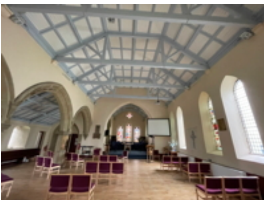
Nave Ceiling Facing East
