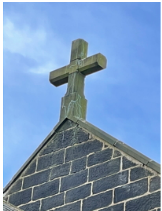
Nave East End Finial
