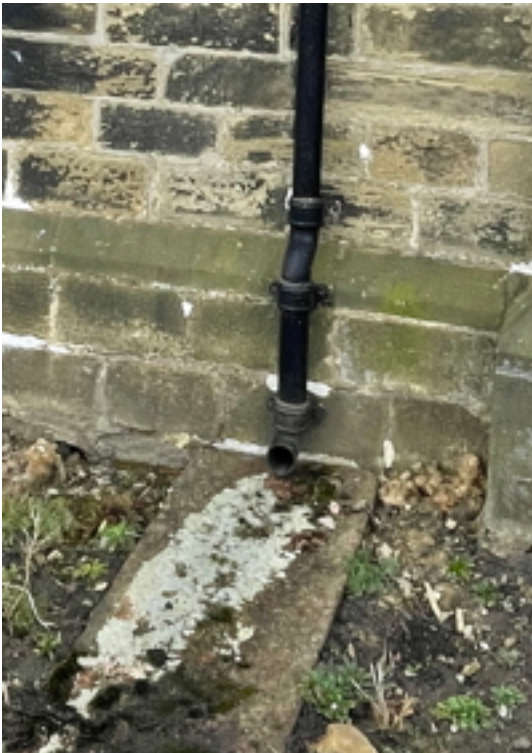
Typical run off on concrete slab
