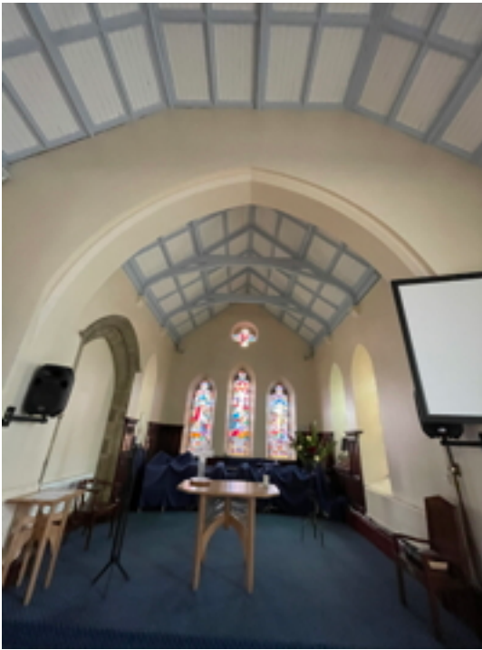
Chancel Ceiling Facing East
