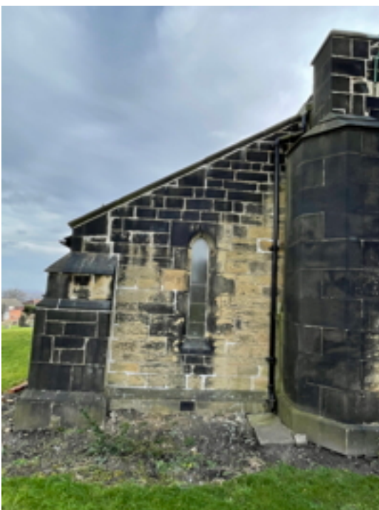
West Wall North Aisle
