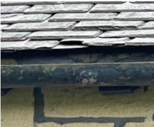
Typical Cast Iron Gutter
