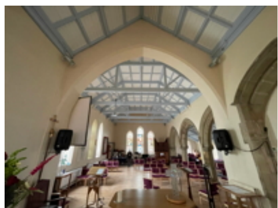
Nave Ceiling Facing West
