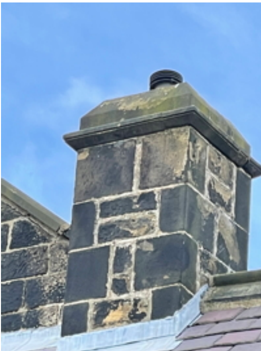
Chimney over North Transept Finial
