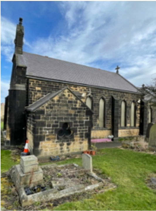
South Nave Roof
