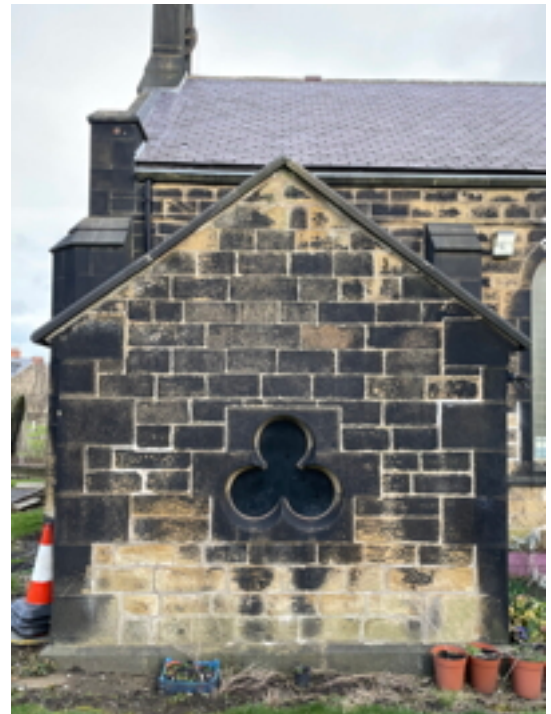
Window 24 South Porch, trefoil window infilled with plywood
