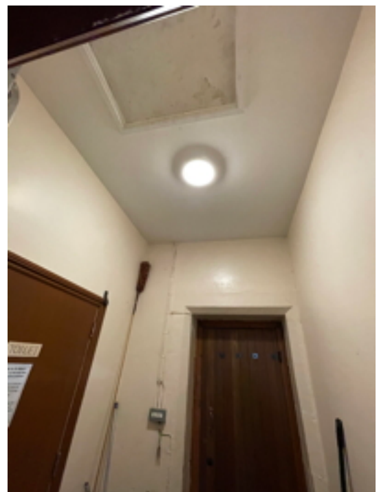
Typical Fluorescent Lighting
