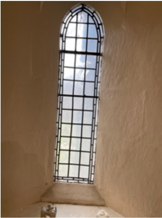
Window 15 North Aisle, temporary polycarbonate-glazed with applied lead tape.
