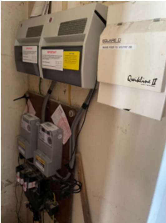
Porch DB Boards
