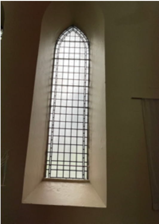
Window 3 Leaded, plain glass, good condition
