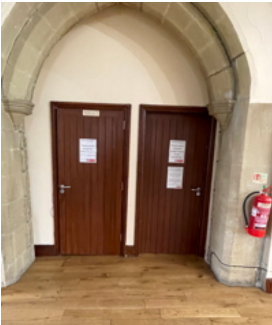
Exit Door Signed as WC
