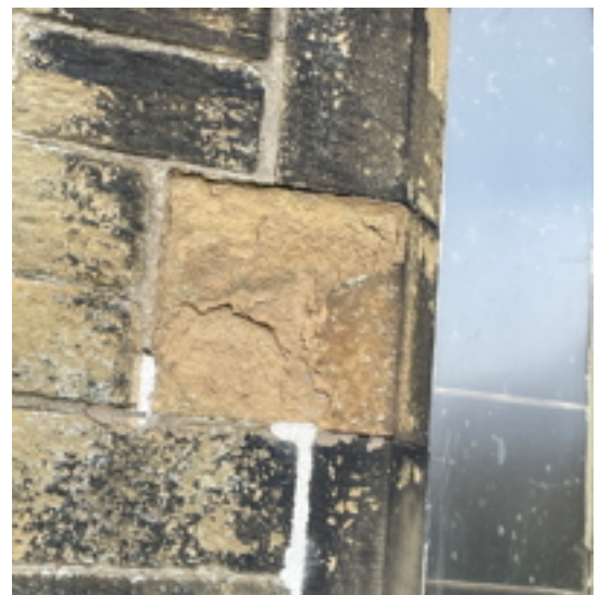
Eroding Stone to West Wall North Aisle
