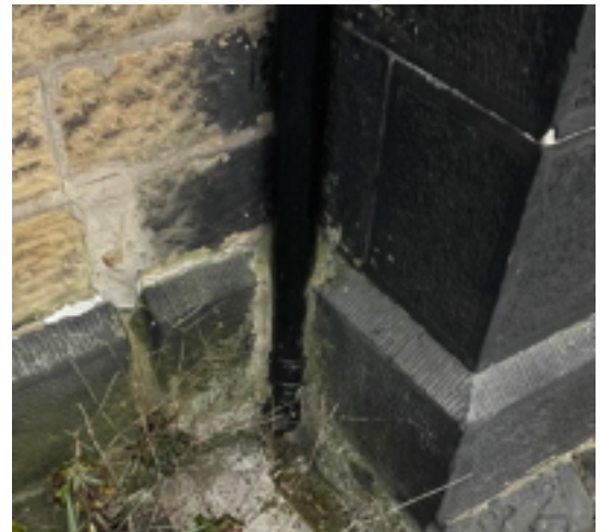
Rainwater Pipe Cemented In
