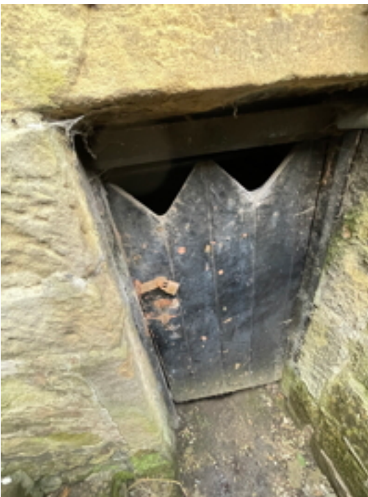
Boiler Room Door
