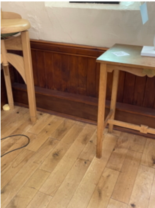
Nave South Side
