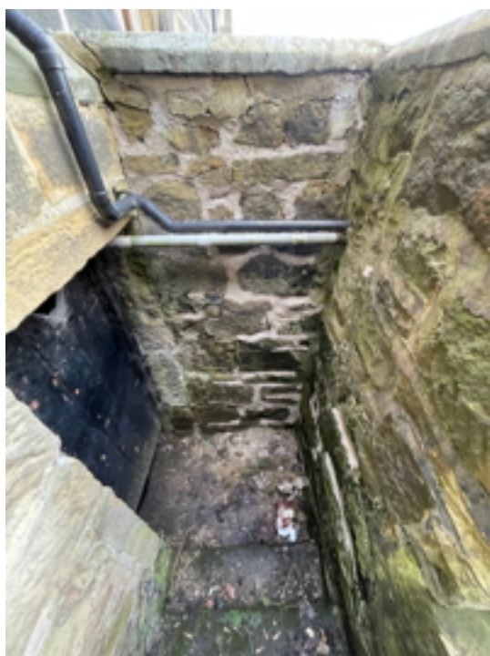
Boiler Room Steps
