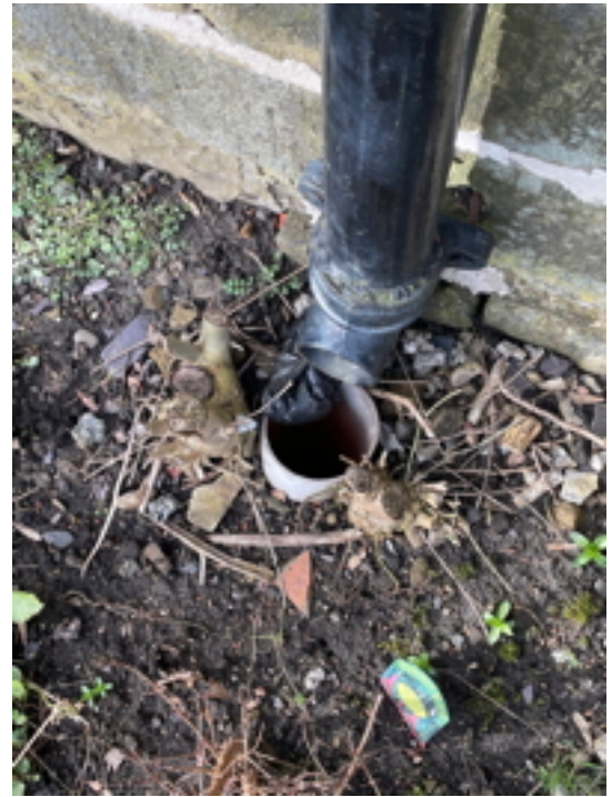
Gully Missing to Drain
