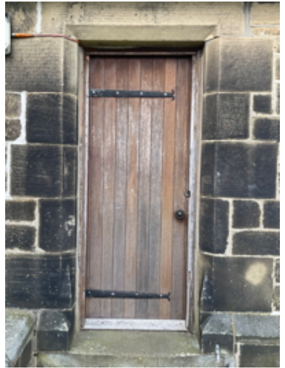
East Lobby Door, Boarded door with iron strap hinges
