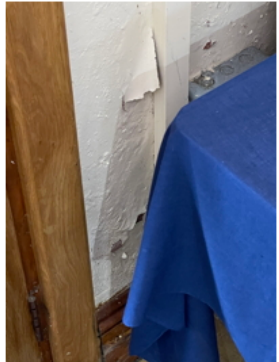
Peeling Paint to RHS of Door to Entrance Lobby
