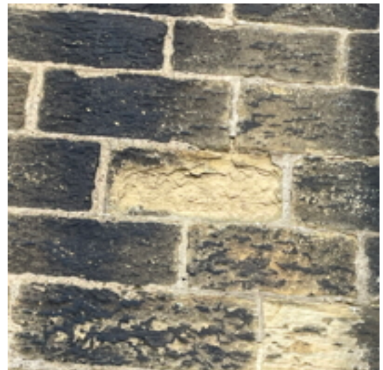
Eroding Stone to West Wall
