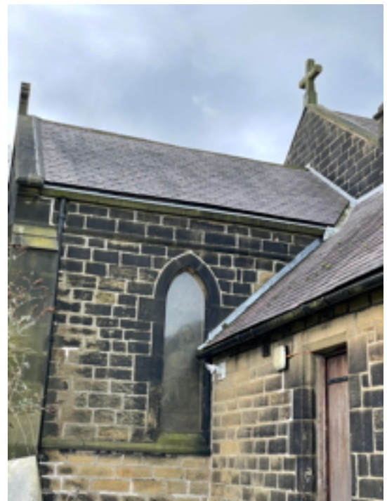
Chancel North Roof
