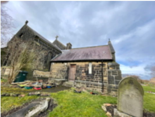
North Transept East Roof
