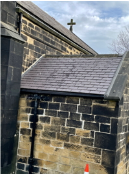
Porch West Roof
