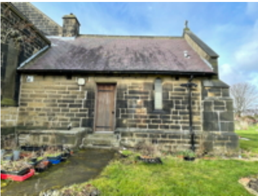
North Transept East Wall
