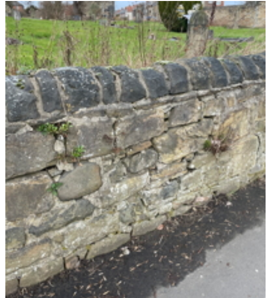
Typical Stone Walling
