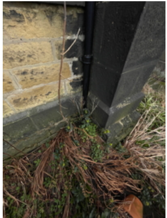
Bottom of pipe blocked by vegetation
