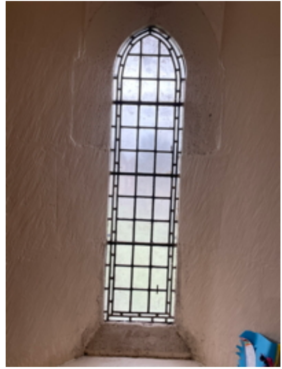
Window 18 North Aisle, single lancet, plain.
