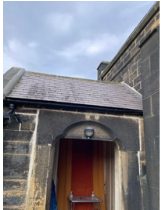
Porch East Roof
