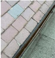
Figure 10 – Pooling in gutter above south aisle
