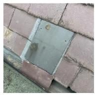
Figure 8- Poor tile replacement
