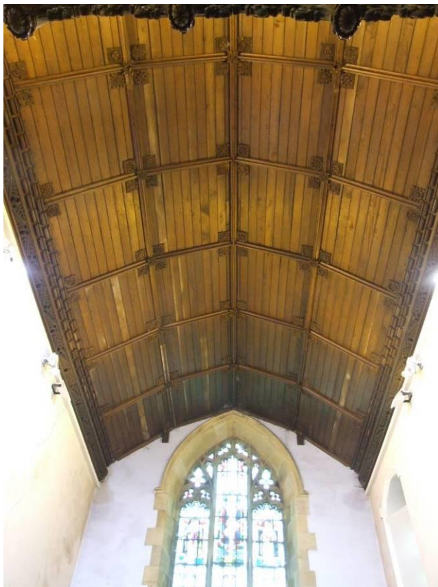
P27 (8728): Chancel ceiling; some water staining
