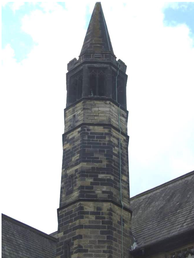
P45 (8760): Weathered stone below bell tower tracery
