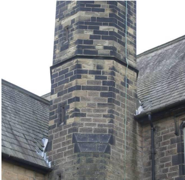
P44 (8759): Valleys to tower; displaced slates
