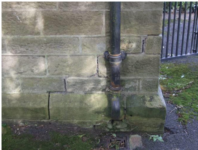
P33 (8737): Porch, southwest corner; joints opening from settlement
