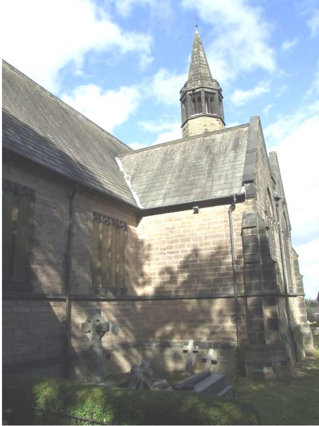
P30 (8732): South transept, west end: damaged monuments, plastic guttering, displaced valley slates, small areas of high level pointing missing
