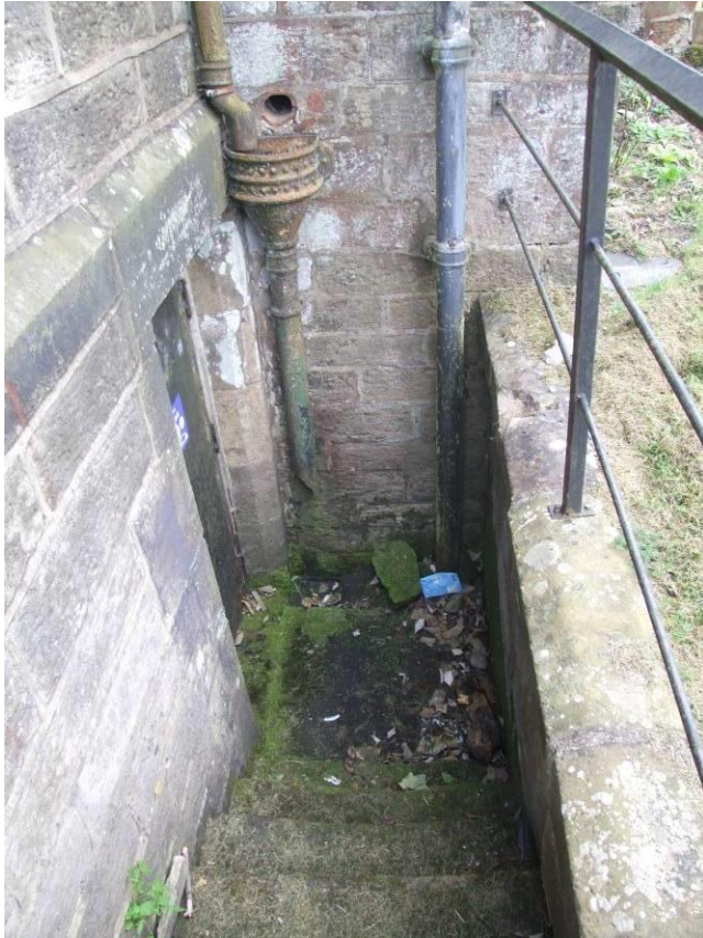
P41 (8753): Boiler house steps
