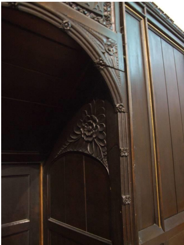
P17 (8702): Vestry door, cracked carving to right hand side
