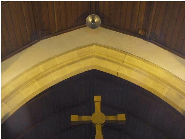
P24 (8719): Minor cracking to chancel arch
