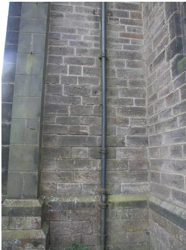
P47 (8765): South transept, east wall; missing pointing
