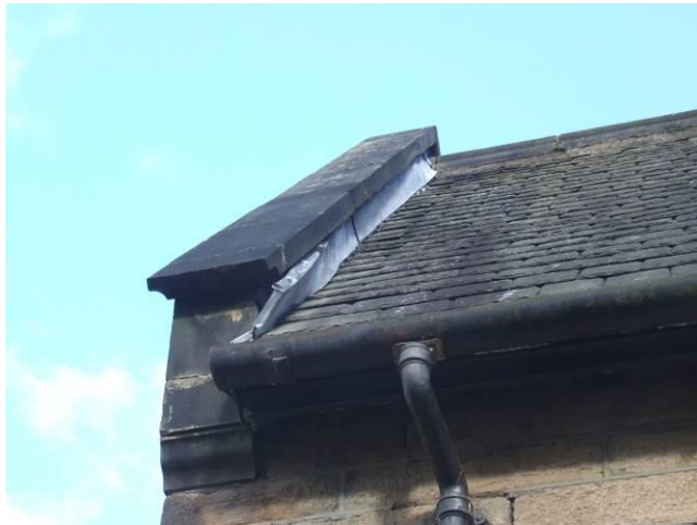
P38 (8744): North transept, west side; displaced lead flashing
