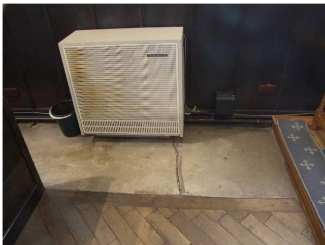
P6 (8675): Concrete slab movement in Lady Chapel
