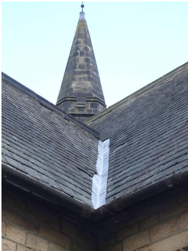
P39 (8746): North transept, west side; displaced slate in valley
