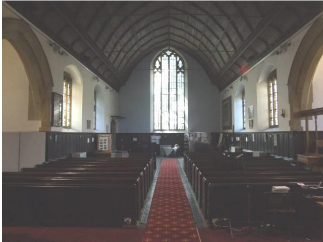
P23 (8716): Nave from east
