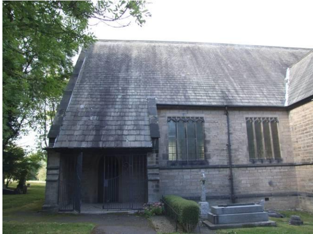
P32 (8734): West porch, displaced slates
