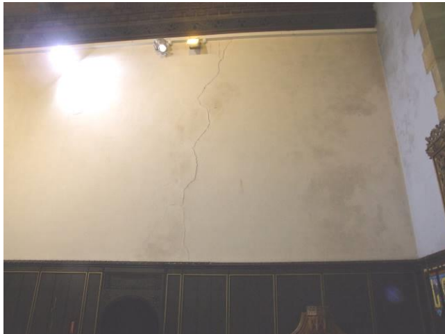
P14 (8689): Cracking to north chancel wall
