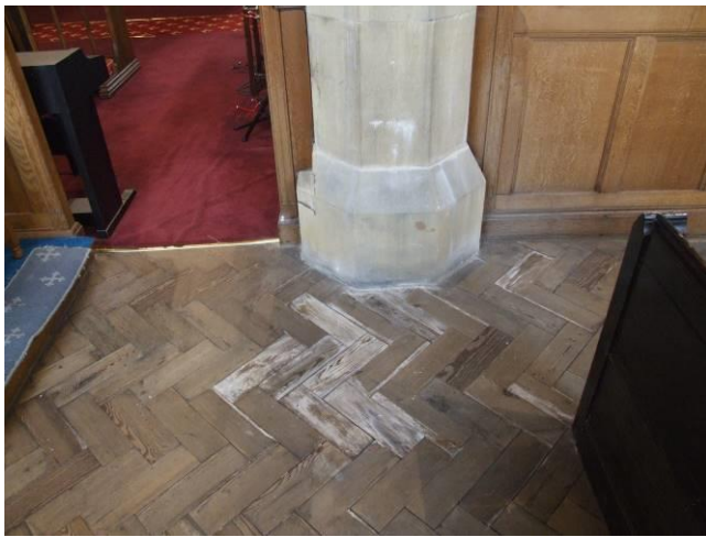
P7 (8677): Evidence of water ingress to Lady Chapel
