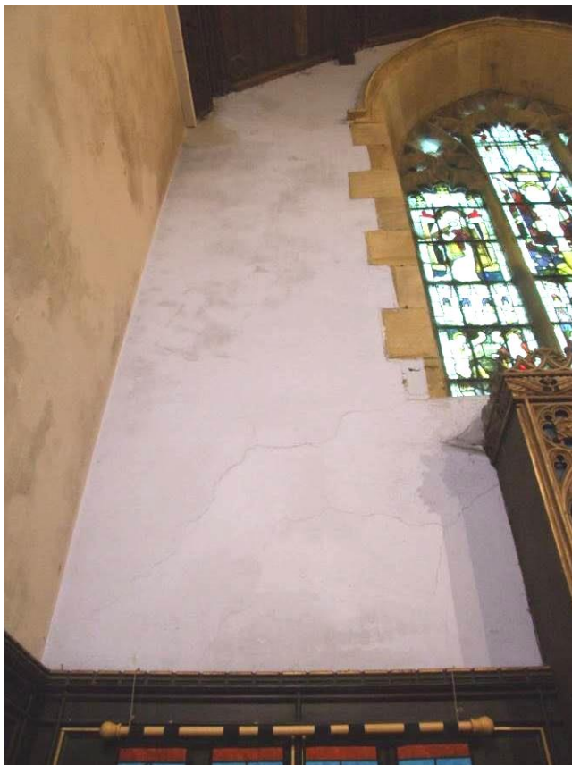
P12 (8686): Efflorescence to wall to eastern/ northern chancel walls
