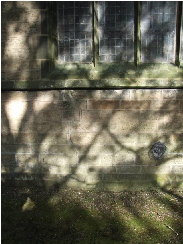
P35 (8740): West end; low level joint opening from settlement
