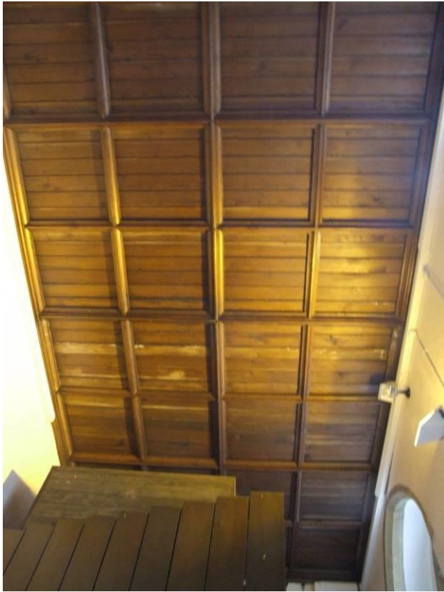
P18 (8704): South transept roof; evidence of water ingress
