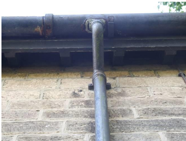
P36 (8741): Failing gutter/downpipe connection
