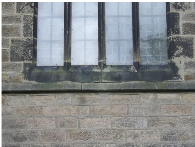
P37 (8743): Open joints, north side window/ drip course
