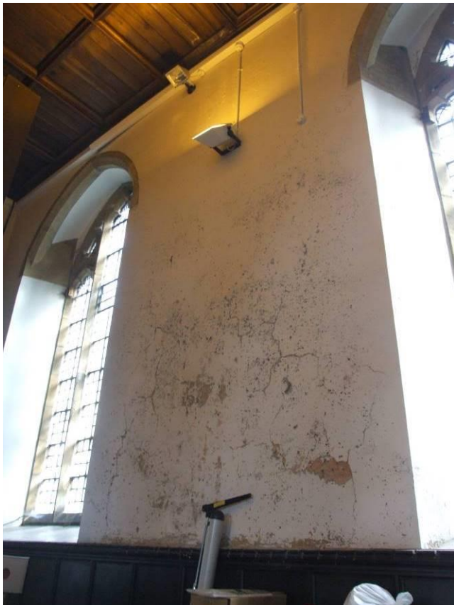
P19 (8705): South transept wall; historic water penetration
