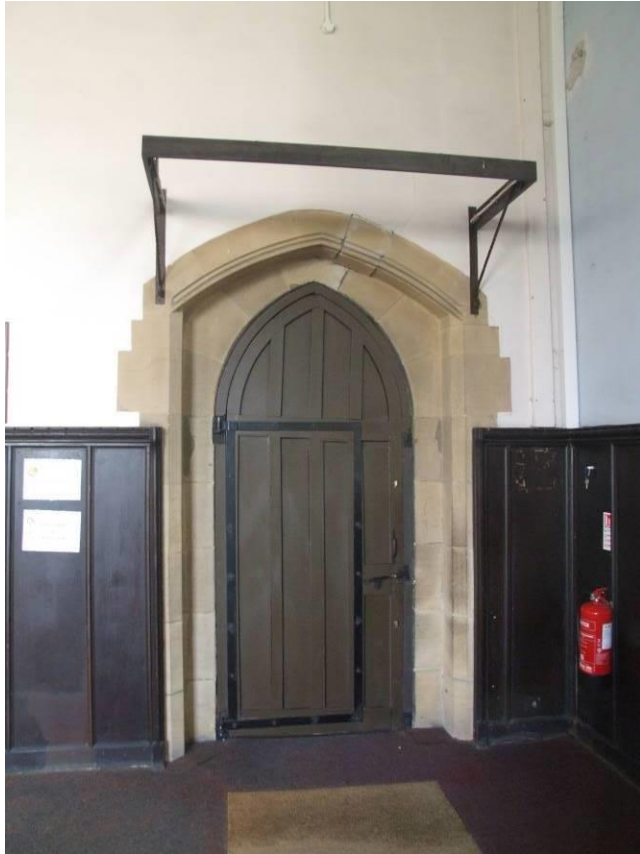
P28 (8729): South entrance door; displaced stone arch
