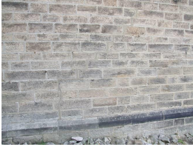
P46 (8764): South chancel wall; minor settlement cracking
