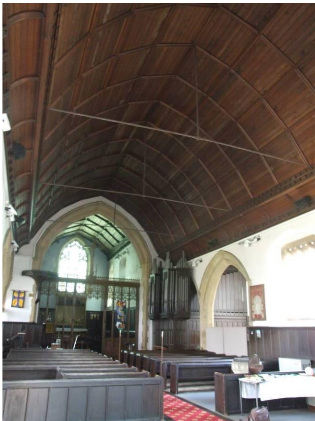
P29 (8730): Nave roof, general view
