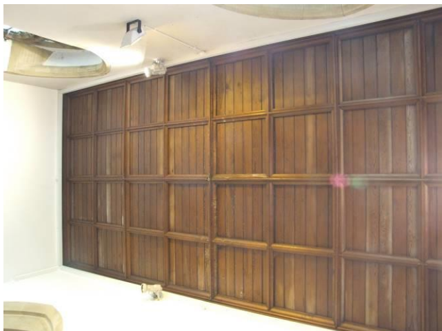
P3 (8672): Chancel roof; signs of water penetration salts
