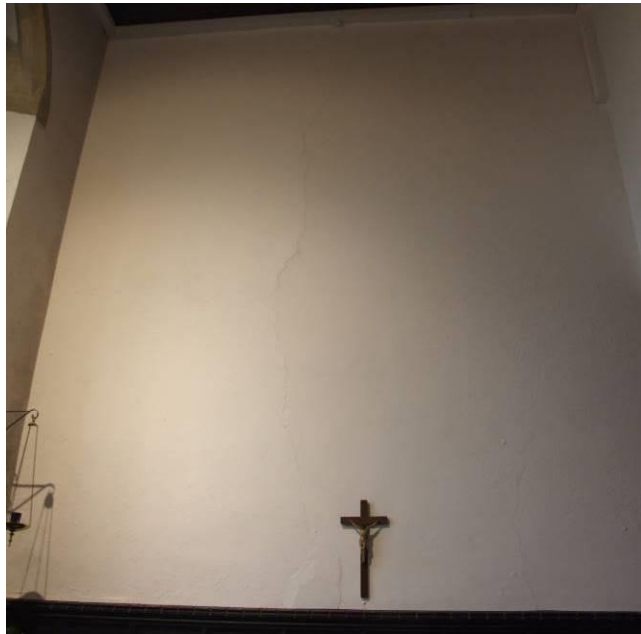
P8 (8679): Vertical cracking to Lady Chapel, east wall
