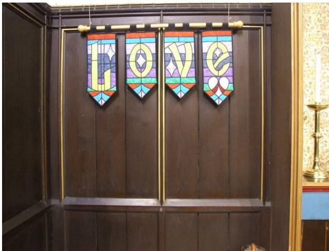
P11 (8685): Shrinkage to wainscoting to eastern chancel wall
