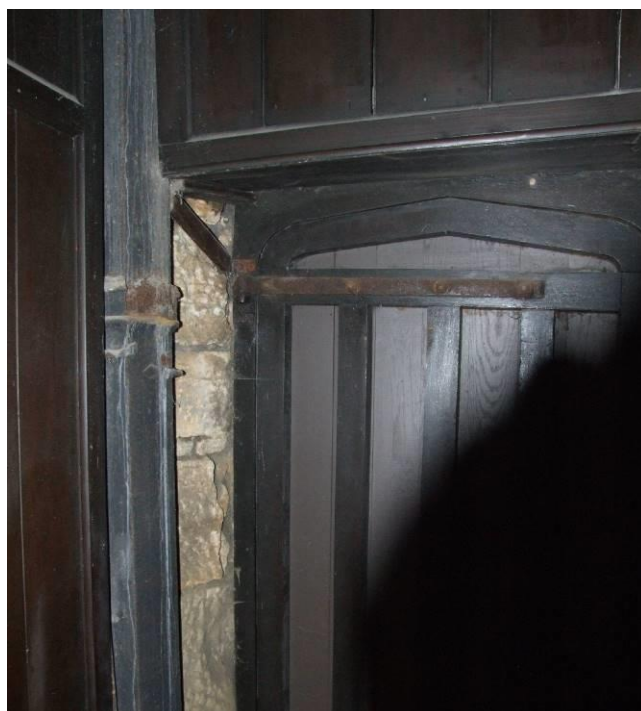
P15 (8690): Internal downpipe adjacent to vestry door
