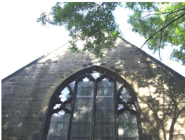
P34 (8738): West end; high level pointing missing, open joints to water tabling
