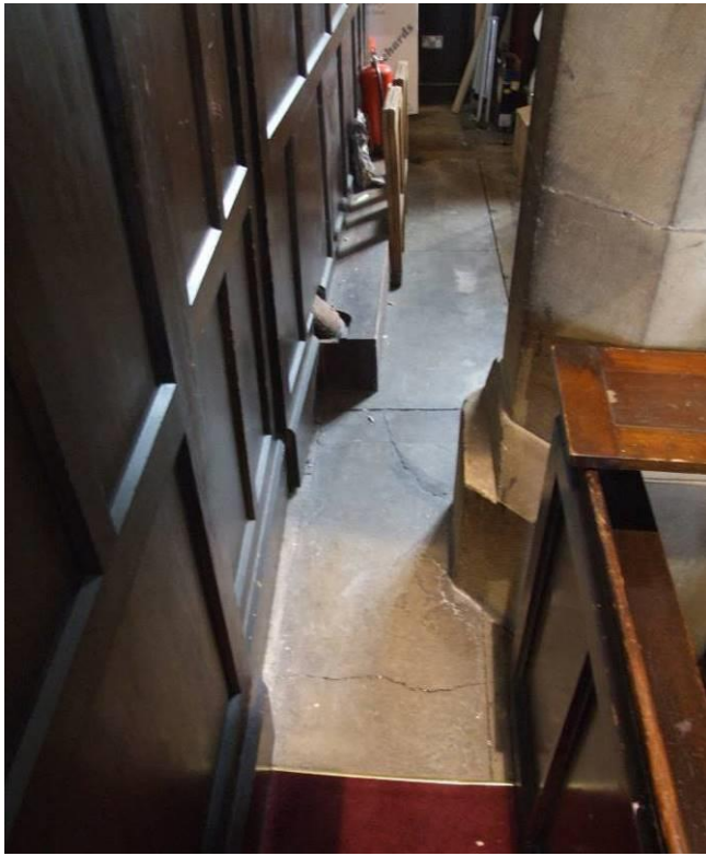
P20 (8709): Concrete slab movement in south transept
