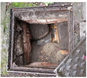
Loose brickwork and soil blocking kitchen branch at NW manhole
