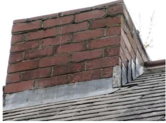
Lead cover flashing missing from NW of chimney
