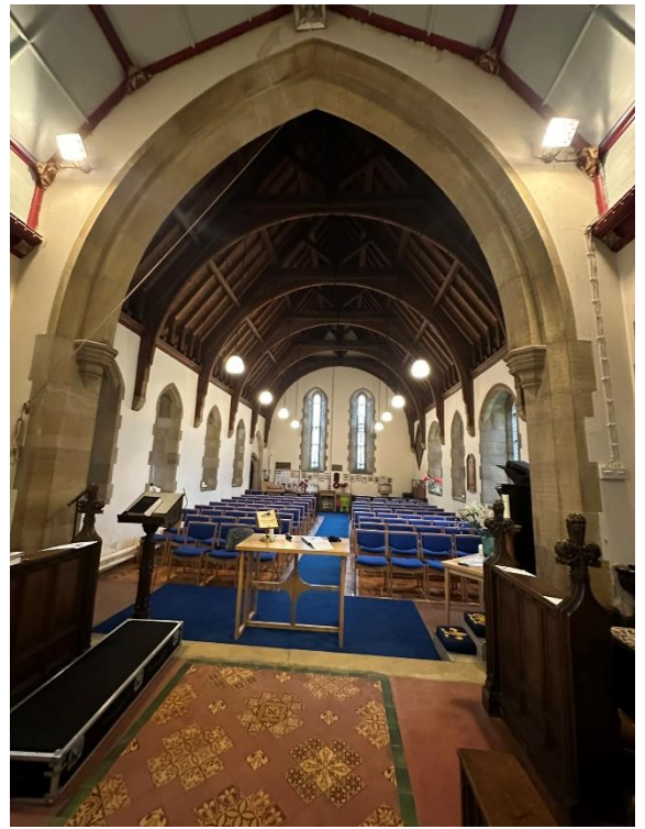
Internal view to Nave
