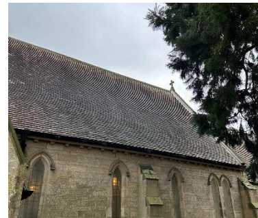
Figure 2- South Nave roof
