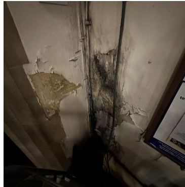
Figure 22- SW Corner Nave
