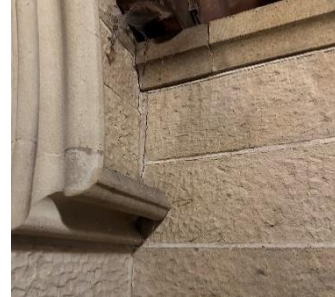
Figure 19 – Porch to Nave abutment
