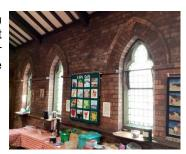
3.52 Hopper vents may require an overhaul. There are some areas of missing or damaged metalwork and damaged glazing. In addition, the hopper vent does not appear to be functional as the strings are missing. They should be overhauled so that they are in good working order.
