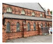
4.22 Particularly at low level there is some open jointing around the buttresses. A programme of raking out and repointing up, perhaps one elevation at a time picking up on open joints, would be beneficial.
