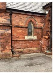
4.59 There is some open jointing and soft brickwork. This would benefit from being repointed.
