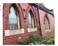
4.28 There is a little bit of evidence of the movement that has taken place over in the heads of the two westernmost windows and through the cill of the central lancet window. They should be repointed so that they can be monitored.
