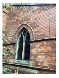
4.45 At high level there is some vegetation within the parapet and spalling stone and missing pointing lower down. It seems likely that water is entering the wall top here and this has caused the spalling of the bricks and the loss of mortar. Vegetation needs removing and open joints need to be repointed.
