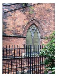
4.34 At high level there is a fracture running through the parapet that appears to have been caused by the vegetation that has taken hold within the brickwork. The vegetation needs removing as soon as possible and the fracture pointing back up.
