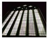
3.65 The tracery windows were somewhat difficult to view from below. However, from what could be seen, they appear to be in reasonable condition. The glazing is apparently straight, and from what could be seen, all elements such as saddle bars and copper ties seem to be intact, however, none of the hopper vents are operational which is a shame and it would be a desirable improvement to bring these back into use.
