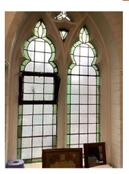
3.32 Damaged or missing lead cames should be repaired.
