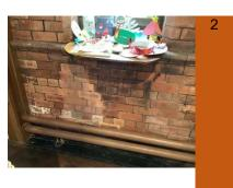
3.50 At high level in the south-eastern corner there is a significant amount of salting. This is from a failed high level downpipe. As this has now been resolved the salting will eventually wear away. However, brushing it and repointing the joints would be helpful.
