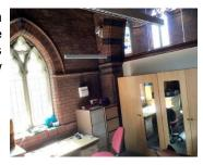
3.2 There is a lean-to ceiling, with purlins and a principal rafter with boarding between. In the south-western corner there is a significant amount of staining. This is understood to be historic from a now repaired roof leak. There are a couple of other areas of staining on the roof, particularly towards the lower reaches and they should be kept under observation.
