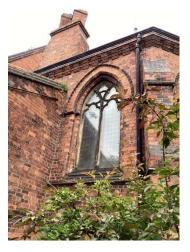
4.38 There is some open jointing to some of the brickwork to the upper reaches of the chimney stack and there is some vegetation slightly lower. This should be removed.
