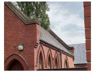
4.9 Pointing to the eastern flashing and the western flashing couldn't be seen from the ground, and so this should be inspected by a roofer. The missing pointing to the flashing should be repointed.
