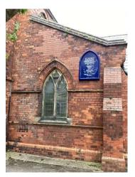
4.53 Both the buttress and parapet have quite a bit of vegetation growing out of them, these require raking out and repointing.
