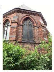
4.42 There are open joints to the tracery of the easternmost window. They should be repointed.
