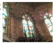
3.14 The plain glazed window seems in reasonable condition, but there is a little bit of openness through the tracery, particularly on the southern side. It would be useful to fill these with mortar. There is a fracture that continues through the cill of the southern window, and it seems likely that this openness to the tracery is related to that. Filling both with mortar would allow for monitoring.
