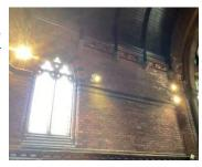
3.12 At either side of the chancel, although most pressing on the south side, there is a significant amount of salting. It seems likely, given the level of this, that this is due to either a flashing or a guttering issue. Once this issue has been resolved the brick should be carefully brushed off and the areas repointed, and the walling should very slowly dry out.
