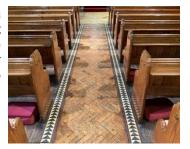
3.63 The PCC should, however, just keep an eye on some areas of the parquet where there does appear to have been suitably fresh damage. It might be that this is just from wear and tear, but it's also possible that it has come from a little bit of dampness within the timber. This should be kept under observation, and if there is a worsening of these areas, the architect should be informed so that a programme of treatment can be carried out in the future.
