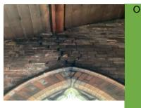
3.6 There was a little bit of salting in the north-eastern corner, particularly on the eastern wall. It seems likely this is related to water ingressing into the wall above. The wall requires repointing very carefully in a soft lime mortar.
