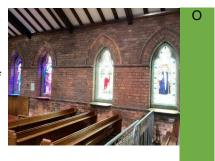
3.71 There is a fracture through the cill of the easternmost window and this should be repointed.
