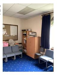
3.24 The grid system ceiling also houses the light fittings. There is a little bit of staining within the corners. However, this is understood to have been historic water ingress and has now been resolved. Ceiling is functional, if a little tired.
