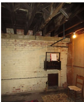
water marked Belfry floor (open to Ringing Chamber)
