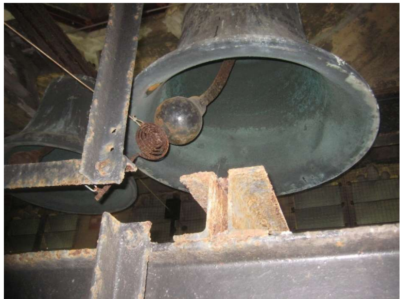
Rusting steels in Belfry
