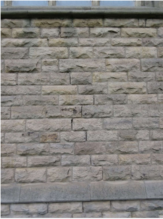
cracked joints at Nave W gable – para 32
