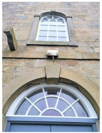
Lose masonry to reveal over fanlight. Crack through jamb to window above
