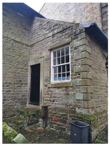
Heavy moss, damp plinth, cementitious pointing - may have caused timber rot to floor internally
