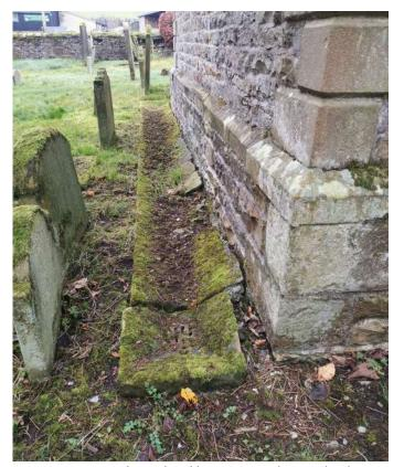
Remove concrete channel and leave exposed to earth. Clear gullies.
