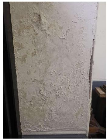
Internal walls of tower worsened - non-breathable paint making issues worse
