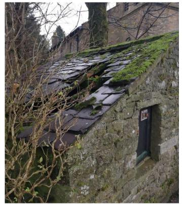
Garden shed roof collapsed - dangerous. Northern wall of shed/boundary wall also collapsed at eastern corner
