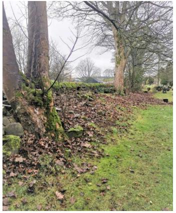
Garden waste against wall will be adding pressure to wall and maintaining a damp wall that could lead to mortar washout and de-stabilisation
