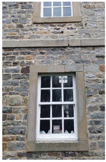
Splits down vertical window jambs. Cracks through head lintel and stringcourse above.
