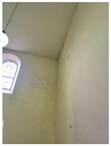
New crack in plaster to west of western window, damp damaged finishes. Tell-tale to western wall
