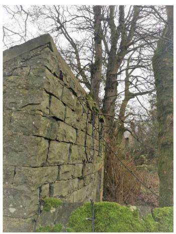
Front of garden shed leaning out and masonry unstable - dangerous - the area in front should be fenced off
