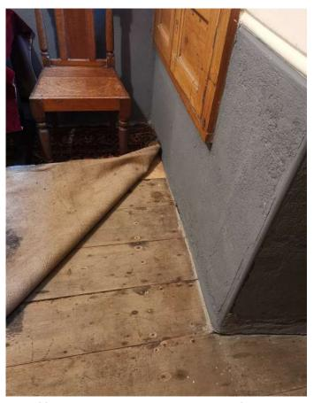
Area of floor to east vestry wall is spongey underfoot indicating lack of support, possibly rotten joists
