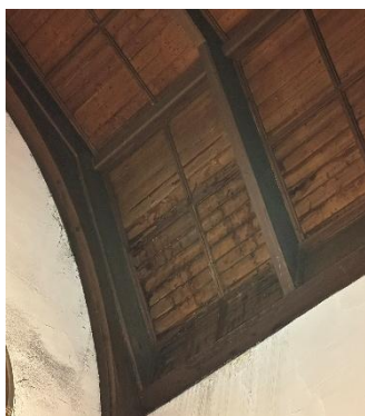
Figure 37 – Chancel South roof
