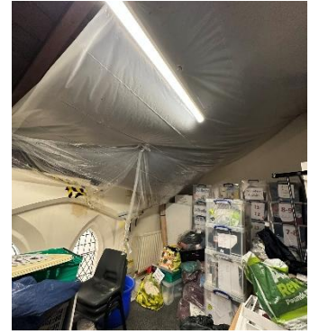
Figure 58 – ceiling S aisle W end
