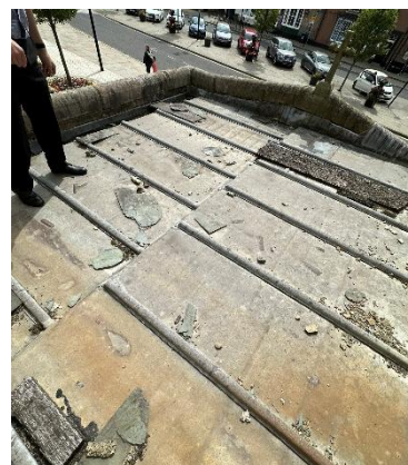
Figure 8 – SE lead roof (over WCs)
