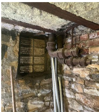
Figure 31 – ceiling and former window
