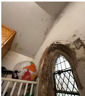
Figure 62 – Vestry ceiling and E
