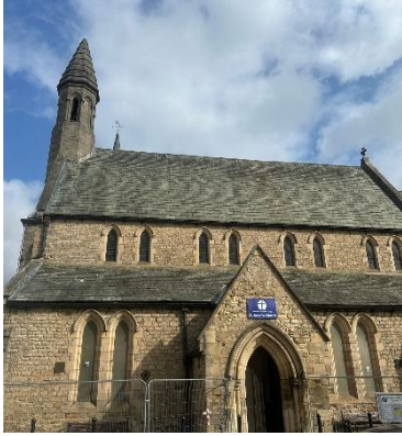
Figure 4- South Nave and Aisle
