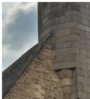
Figure 2 – Coping to NW Nave
