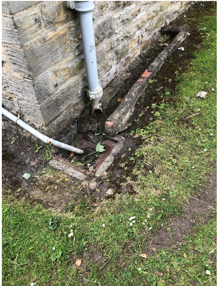
P10 (IMG 7698): Damaged surrounds to gully, to be repointed
