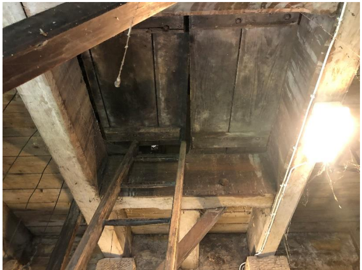
P12 (IMG 7612): Damaged/unsafe spire access ladder
