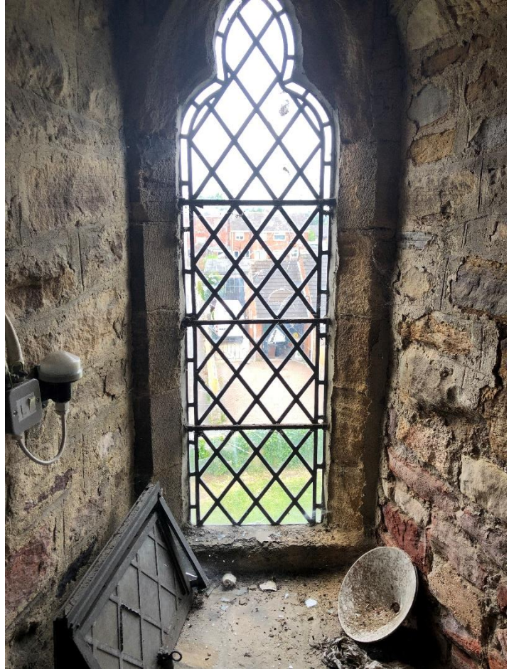
P11 (IMG 7607): Tower clock room, west elevation, showing 3 no. broken panes
