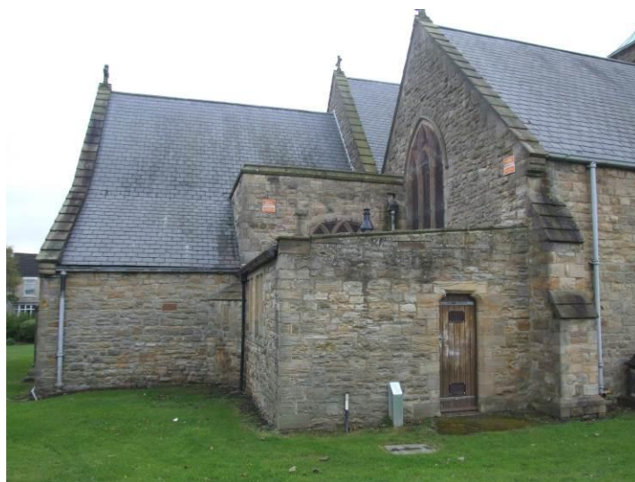
P6 (IMG 476): Chancel, north elevation
