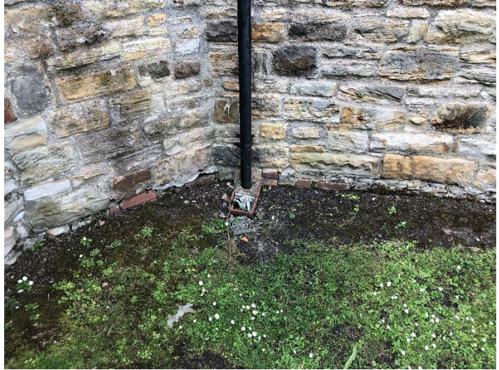
P9 (IMG 7696): Ground gully choked with vegetation
