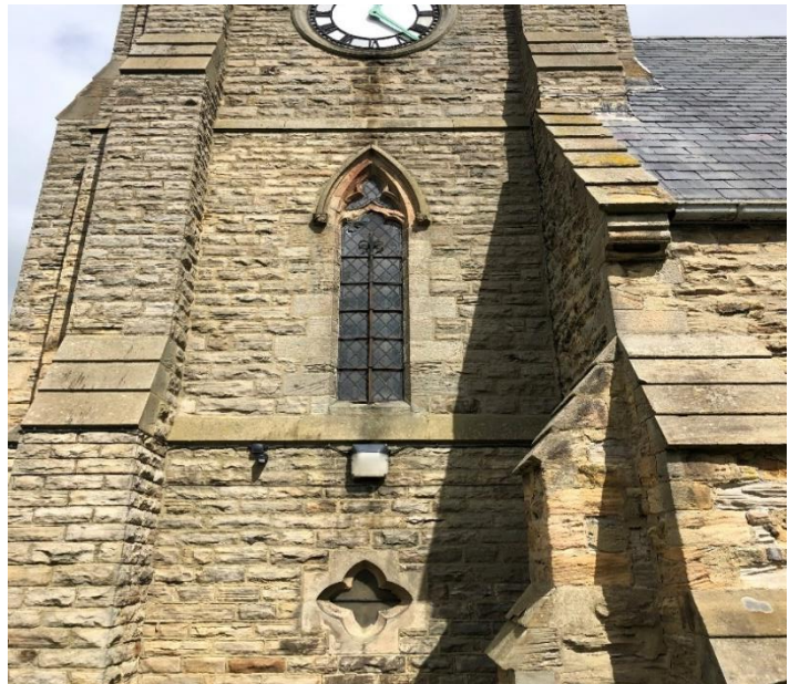
P2 (IMG 7699): Cracked tracery head, lower Tower lancet window
