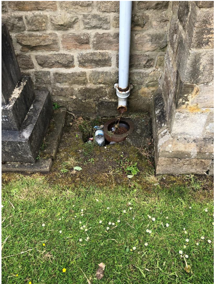
P7 (IMG 7684): Ground gully choked with vegetation/litter
