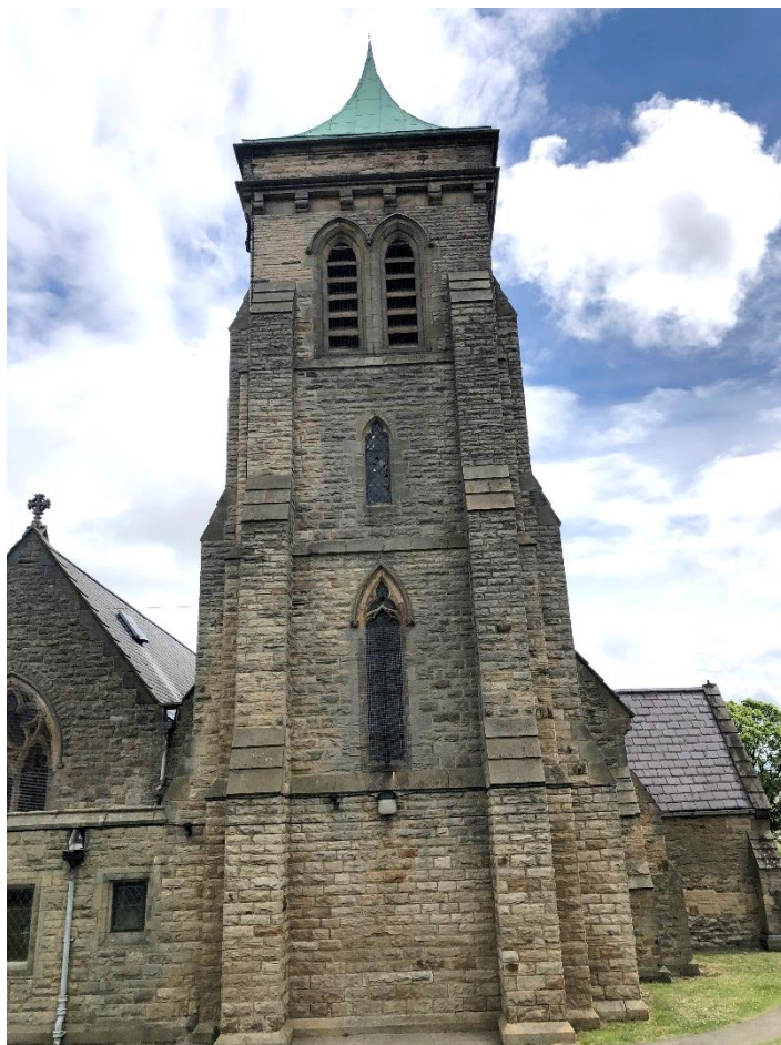
P5 (IMG 7674): Tower, with damaged tracery to lancet window and extensive glass damage to upper lancet window
