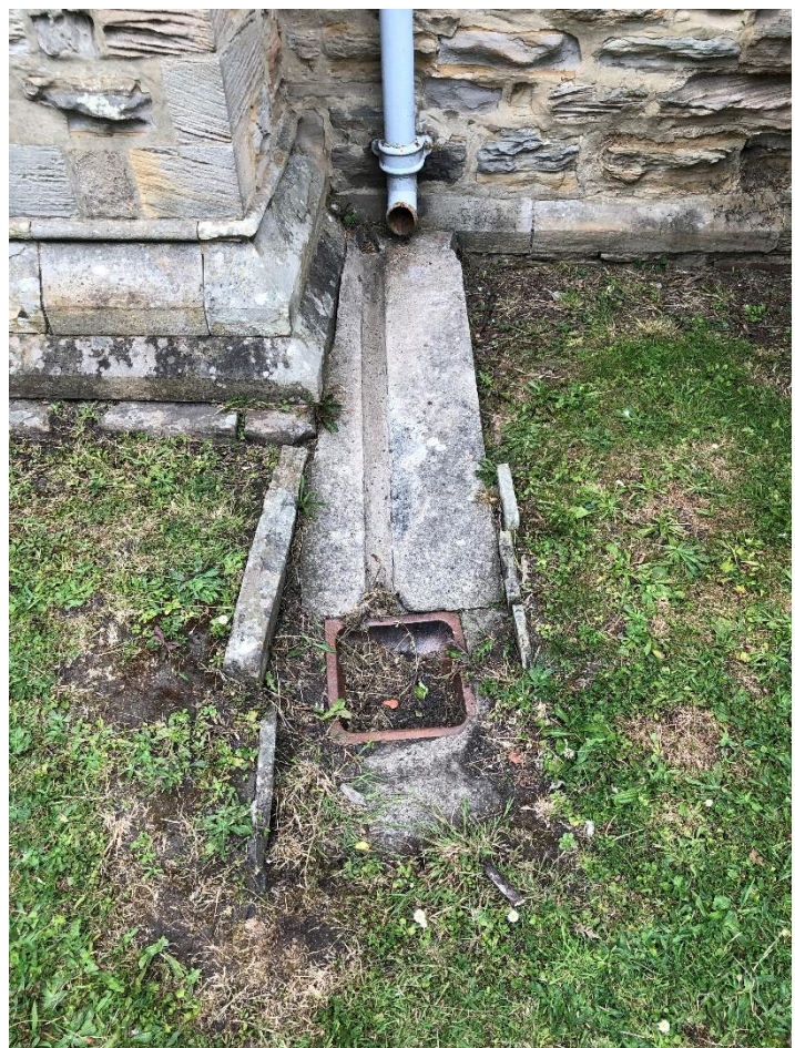
P8 (IMG 7709): Ground gully choked with vegetation
