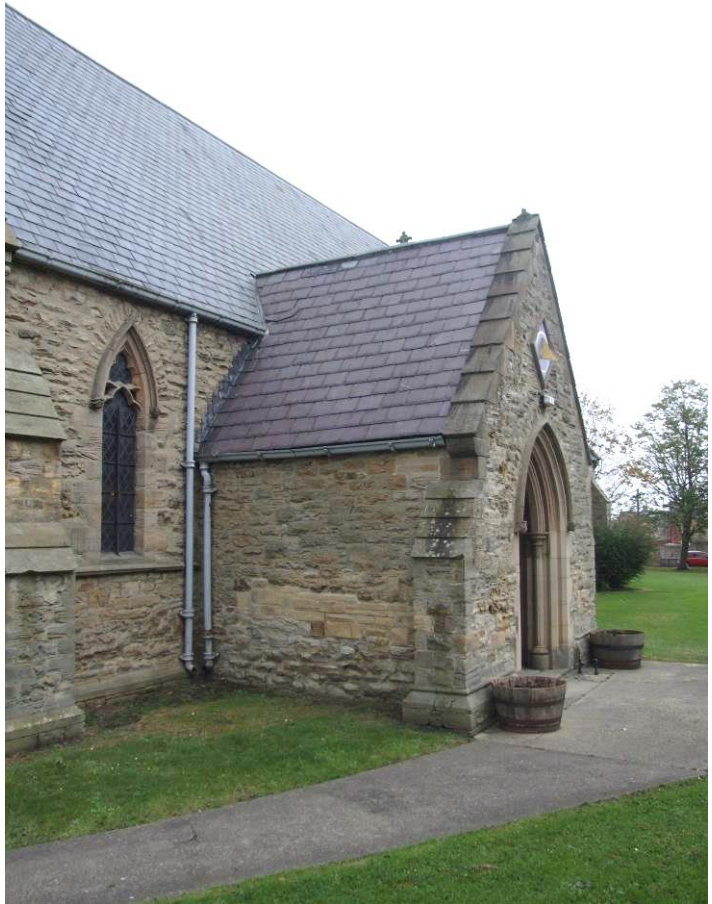
P3 (IMG 458): Porch, with missing apex cross
