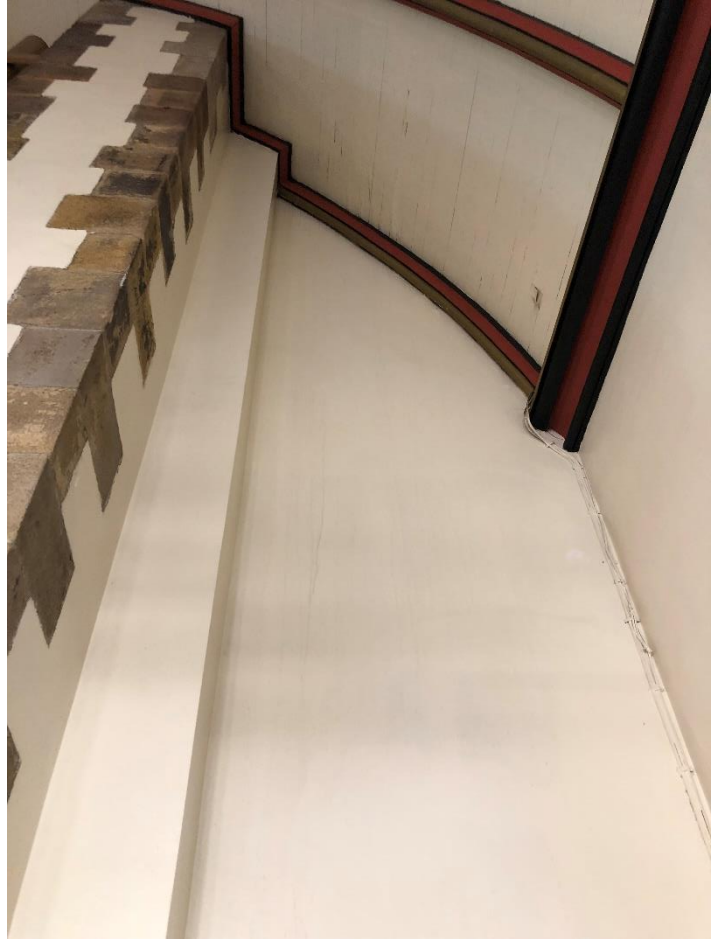
P13 (IMG 7603): Damp stain, northwest corner of aisle
