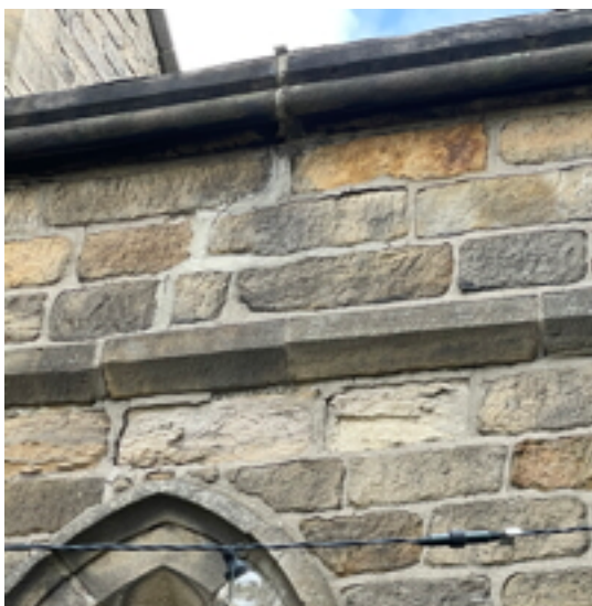
Chancel South Elevation Hard Mortar Pointing
