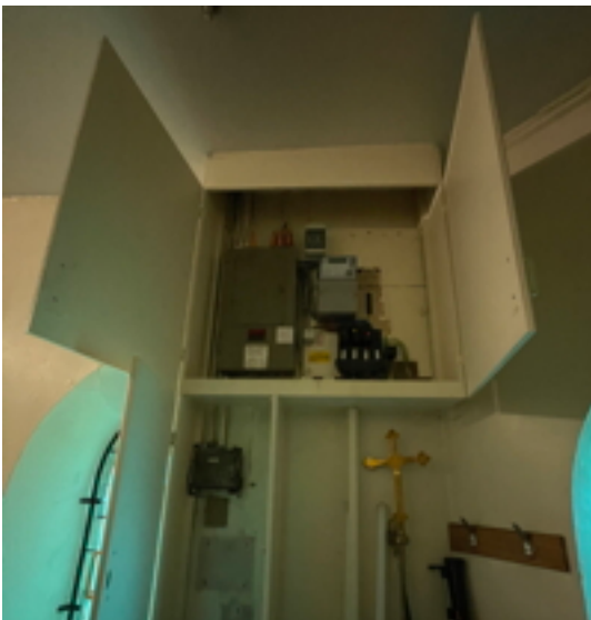
Vestry Incoming Electrics
