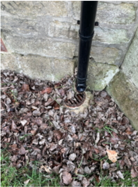
Rainwater Gully Partially Blocked with Leaves
