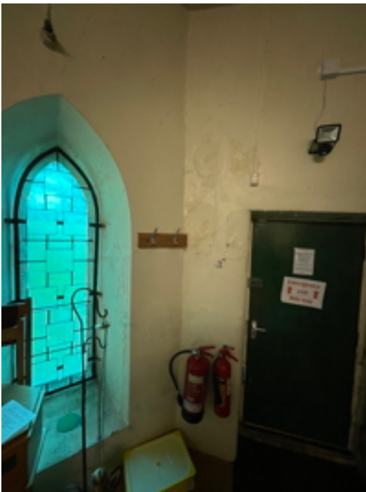
W13 Nave Vestry North East Green Film over Polycarbonate
