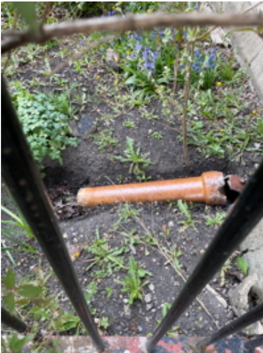
Broken Gully Pipework
