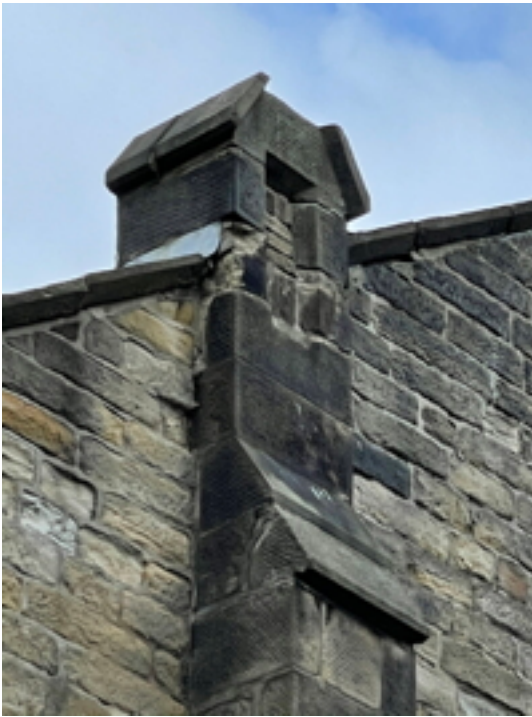
South Gable Chimney
