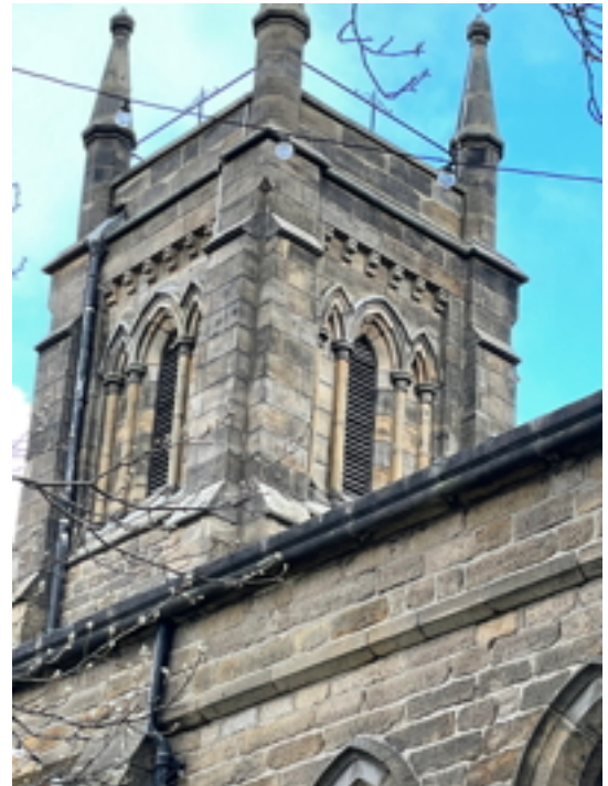
Tower Forth Stage South and East Arcaded Triple Lancets, outer arches blind
