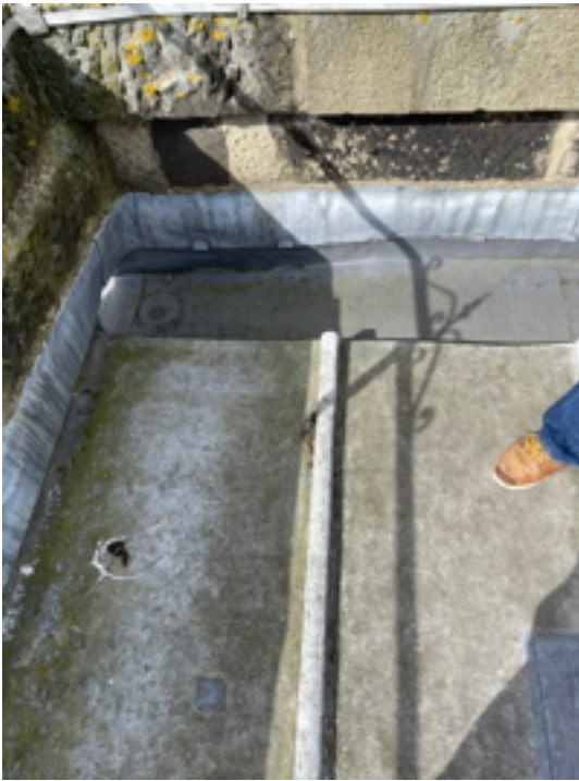
Lead Roof to Tower
