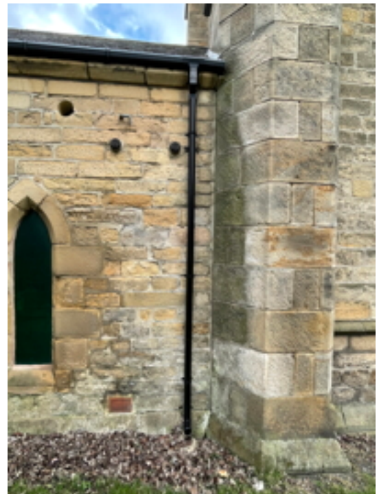
UPVC Rainwater Pipe Vestry North Elevation
