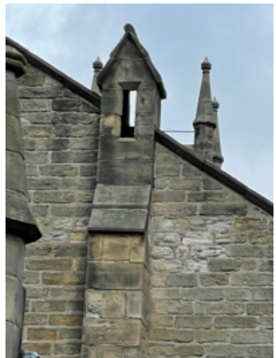
North Gable Chimney
