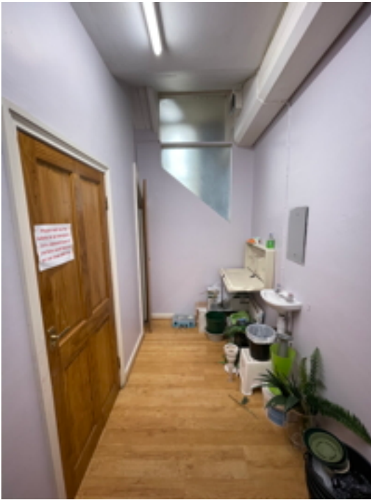
WC Lobby Looking North
