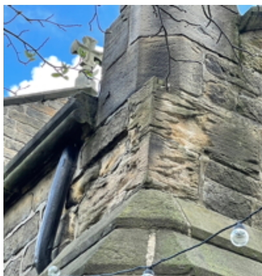
Chancel South East Pinnacle base Deteriorating Stonework
