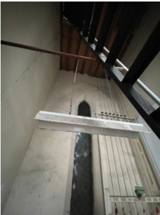
Belfrey Internal East Window Clear Glass with Lead Cames
