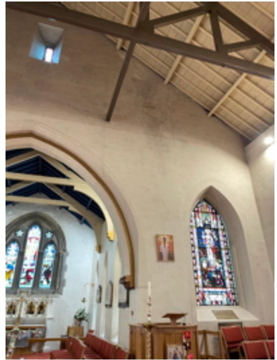
Nave South East End High Level Water Penetration
