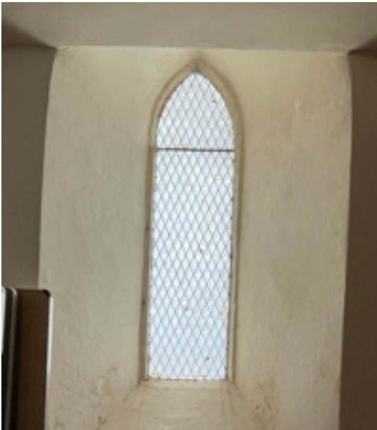
W28 Porch South Window Vandalite Security Glazing
