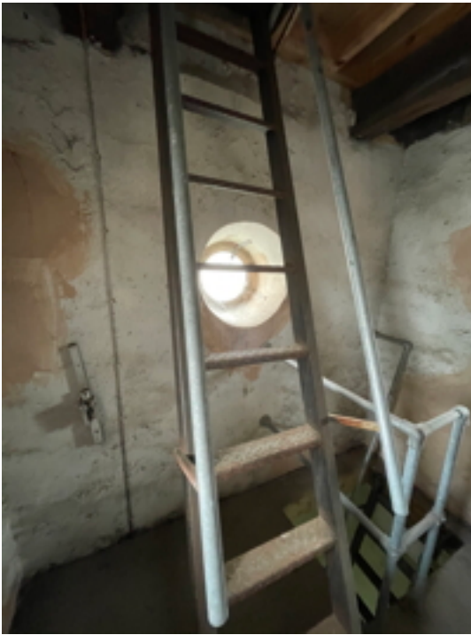
Third Stage with Ladder
