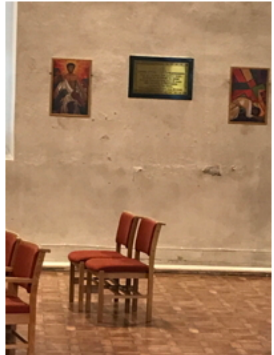
Nave South Elevation Low Level Damp Plasterwork
