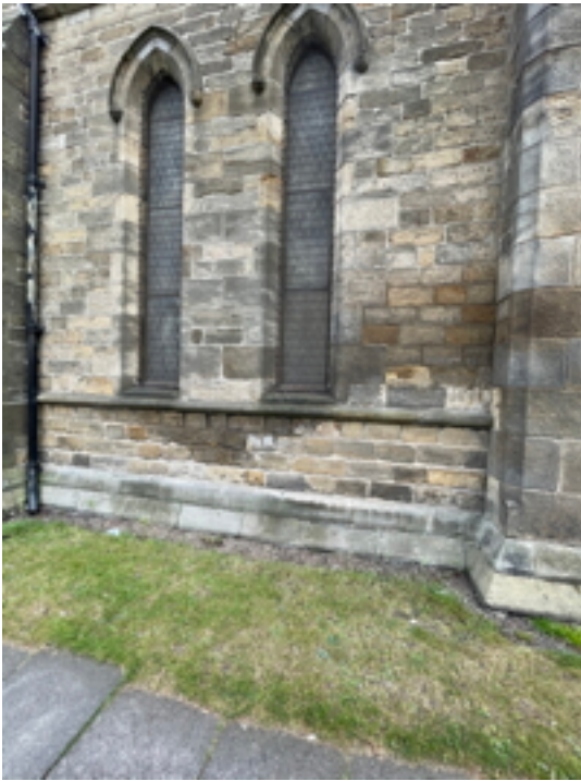
Staining Middle Section South Elevation
