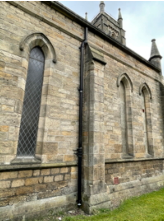
Cast Iron Rainwater Pipe North Elevation
