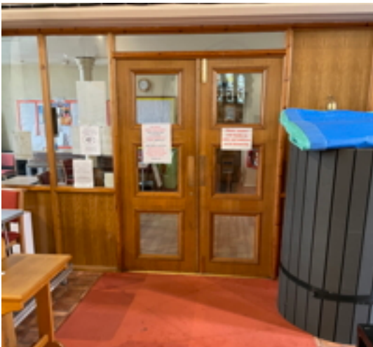
Meeting Room Doors
