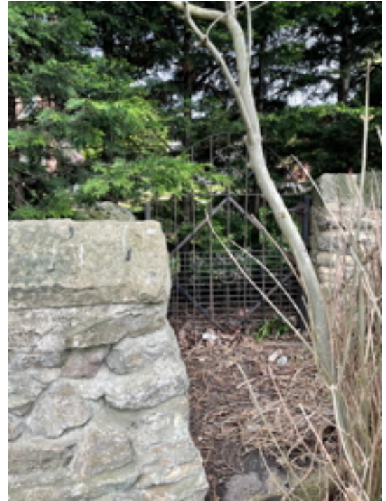
North Wall Gate
