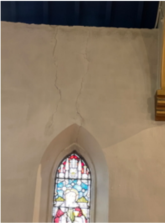
Historic Cracking over Chancel South Windows
