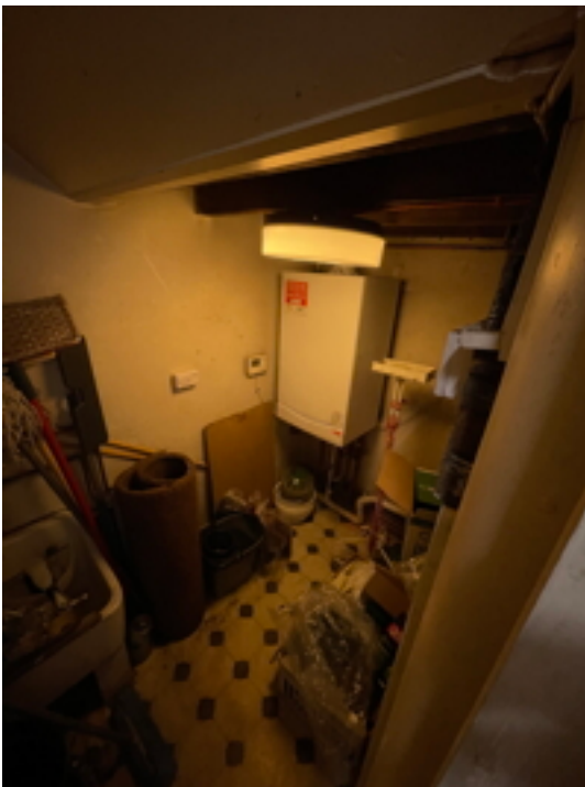
Boiler Cupboard/Cleaners Store
