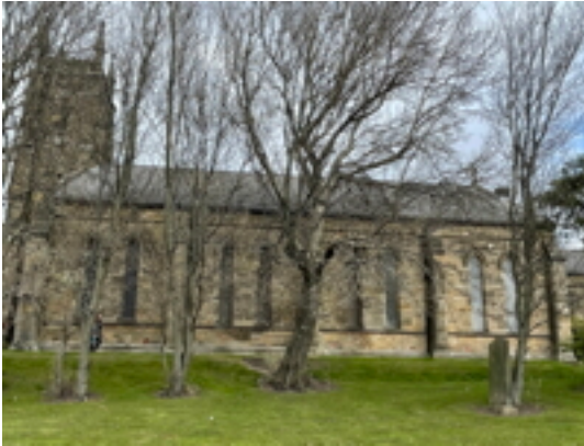
Nave South Roof
