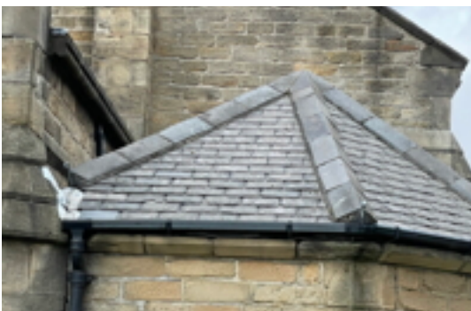
Vestry East Roof
