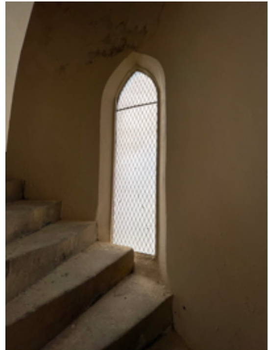
W1 Tower Staircase Vandalite Security Glazing
