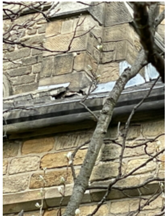
West End Missing Mortar Fillet
