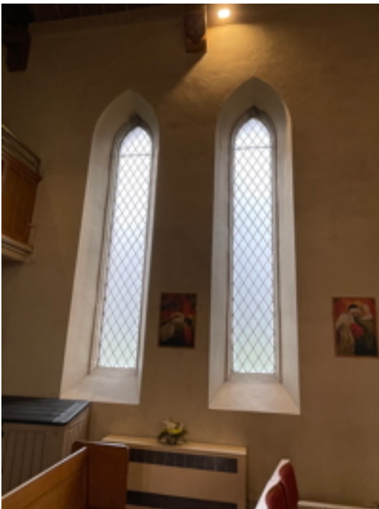
W5 and 6 Nave North West Vandalite Security Glazing
