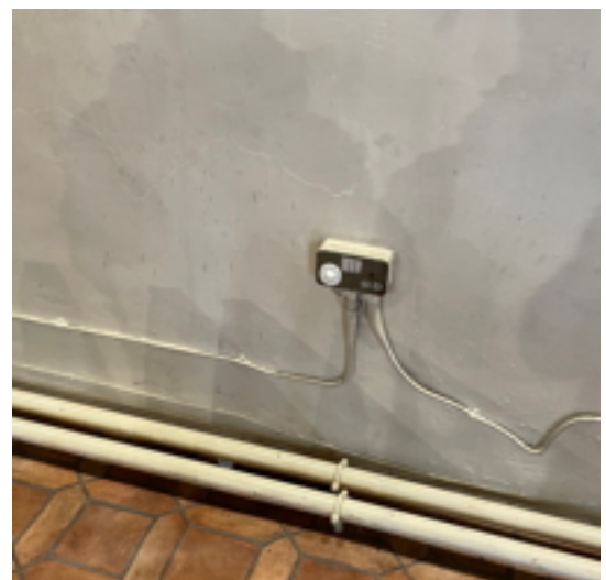
Typical Nave Socket
