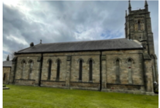
Nave North Roof
