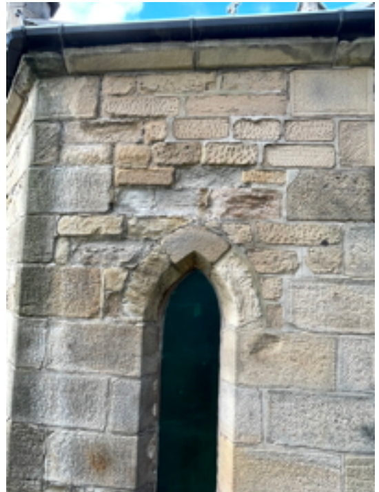
Vestry Deteriorating Stonework
