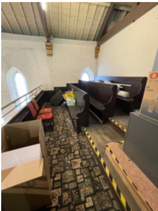
Gallery Looking South
