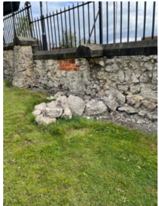
East Wall Damaged Section
