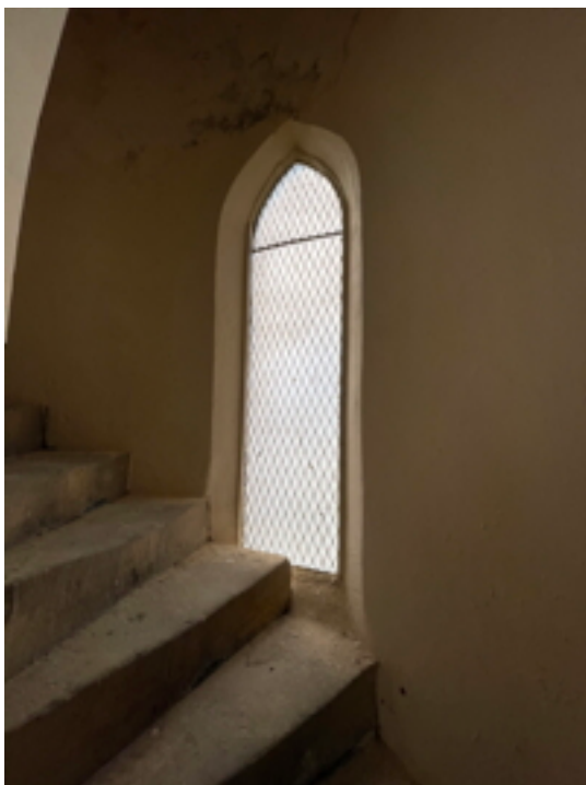
Stone Spiral Stair Leading to Ringing Chamber
