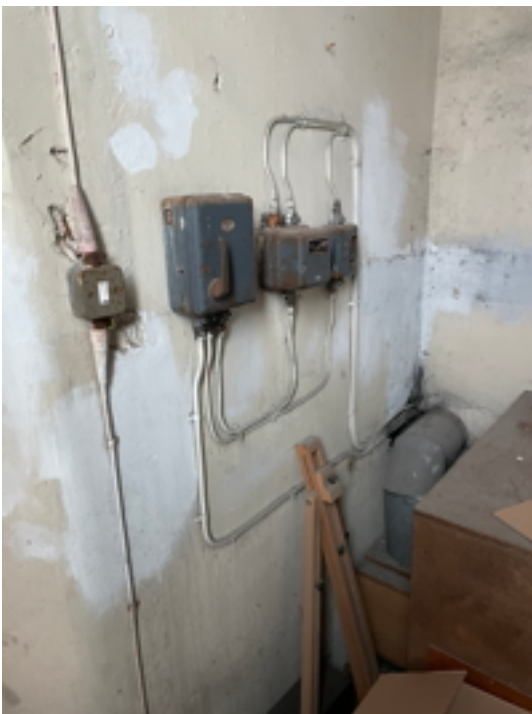
Ring Chamber Distribution Board
