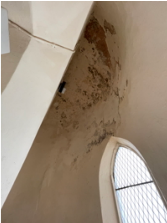
Tower Staircase Ceiling
