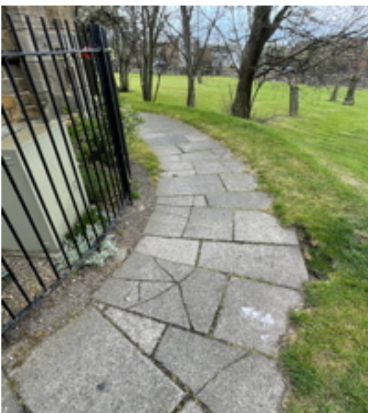
Pathway at South West Corner Broken Flags
