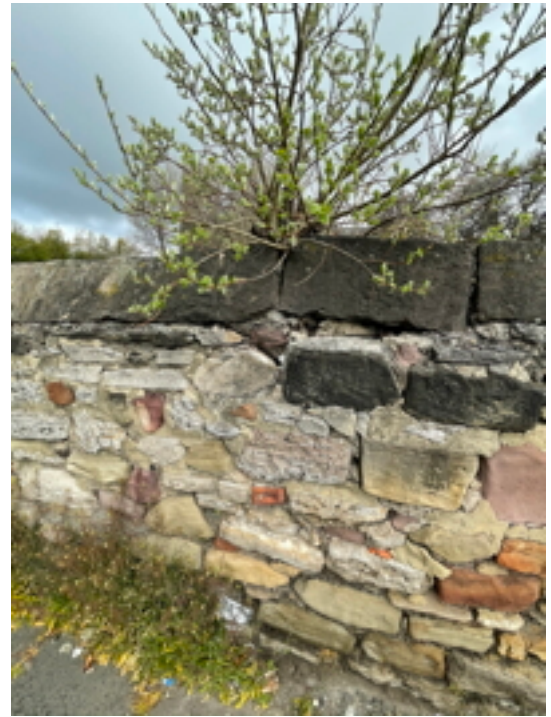
South Wall Damaged Section
