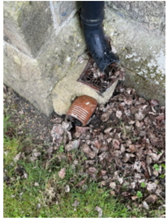
Broken Gully Pipework
