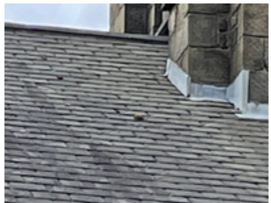
Debris on North Nave Roof
