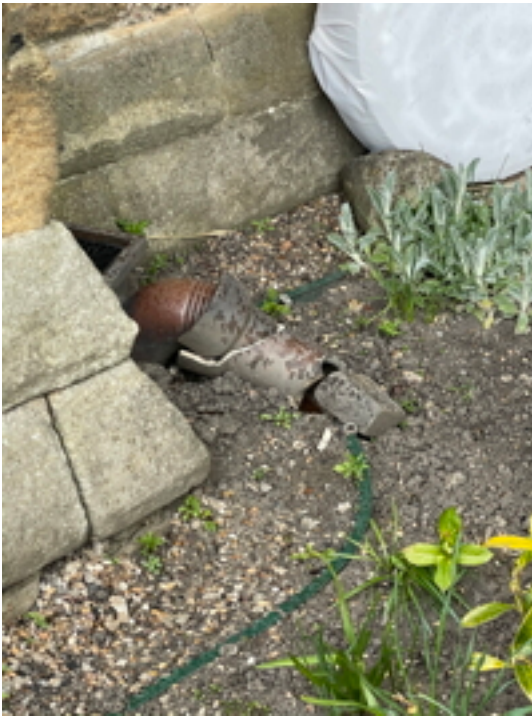
Broken Gully Pipework
