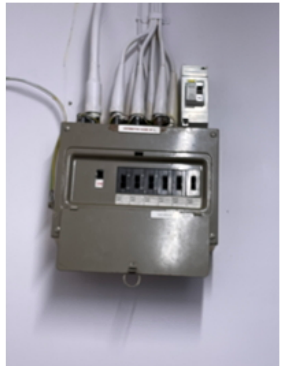
WC Lobby Distribution Board
