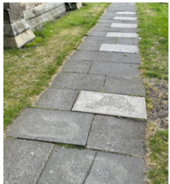
Pathway at South Uneven Flags
