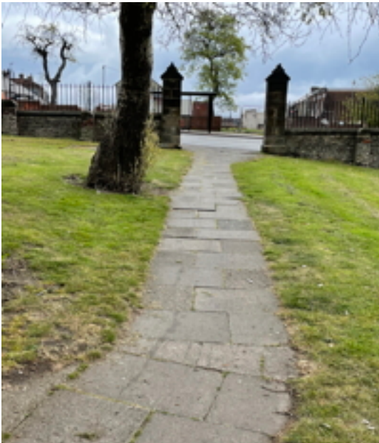
Pathway to East Entrance Uneven Flags
