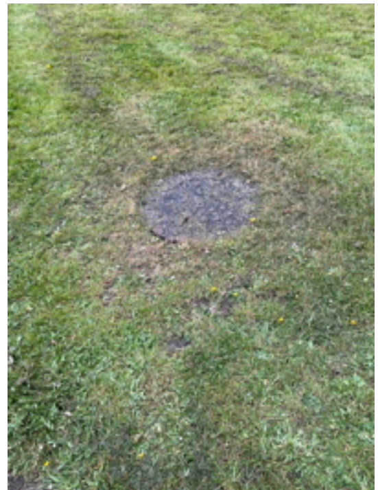
West End Inspection Chamber
