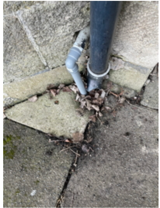
Combined Water Gully Blocked with Leaves
