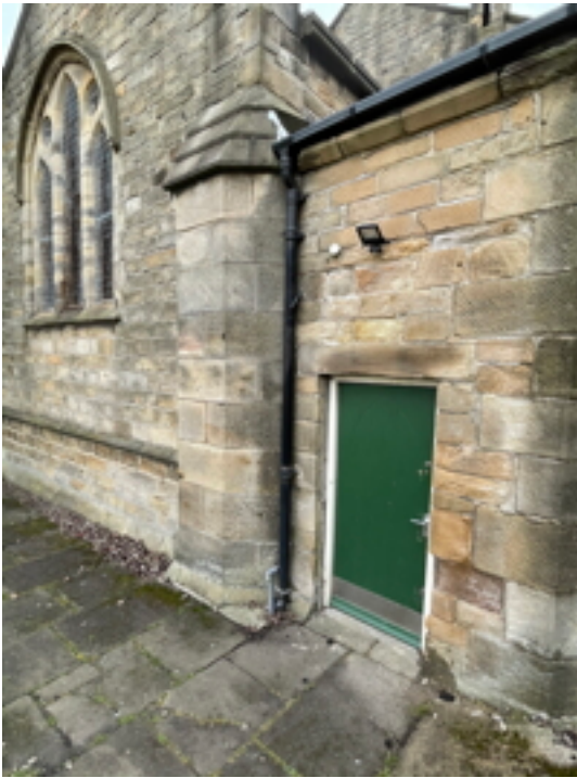
Cast Iron Rainwater Pipe Vestry East Elevation
