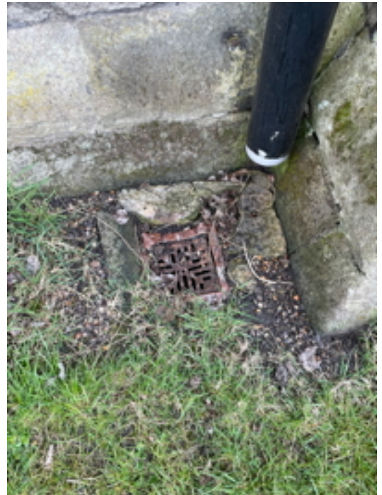
Rainwater Gully with cracked concrete surround
