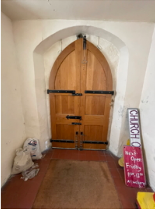
Porch Looking West
