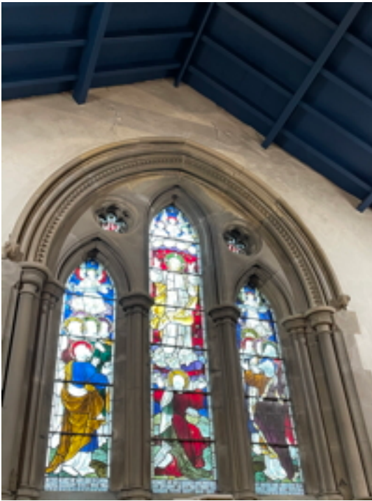
Chancel East End High Level Water Penetration
