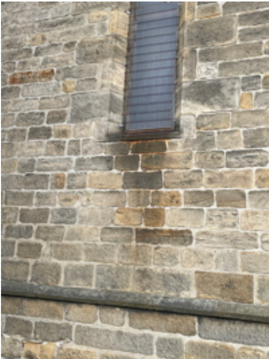
Staining West Elevation South Side
