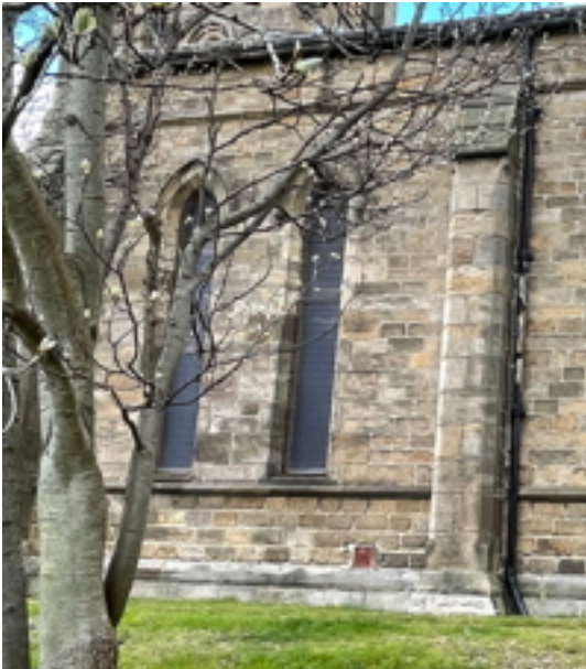
W25 and 26 Meeting Room South Elevation Vandalite Security Glazing
