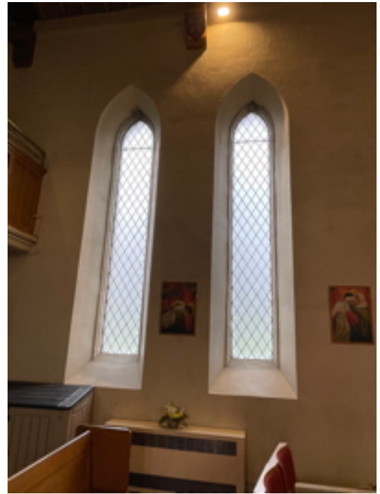
W23 and 24 Nave South Elevation West End Vandalite Security
