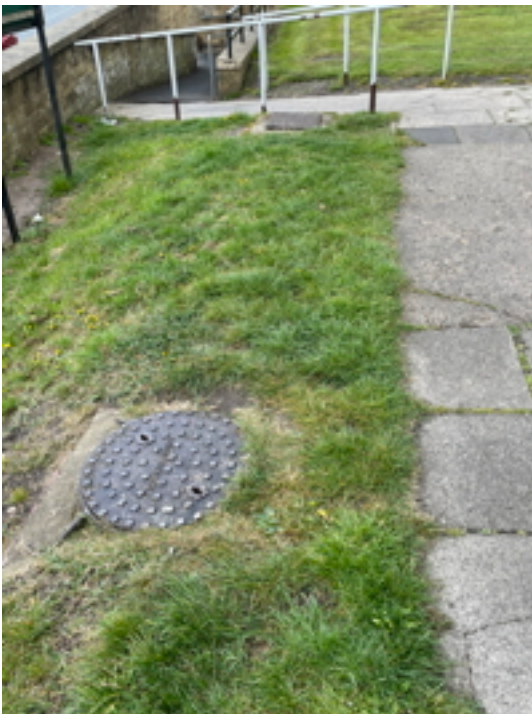
West End Inspection Chambers
