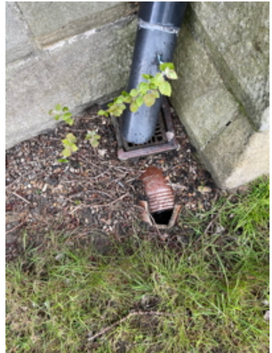
Broken Gully Pipework
