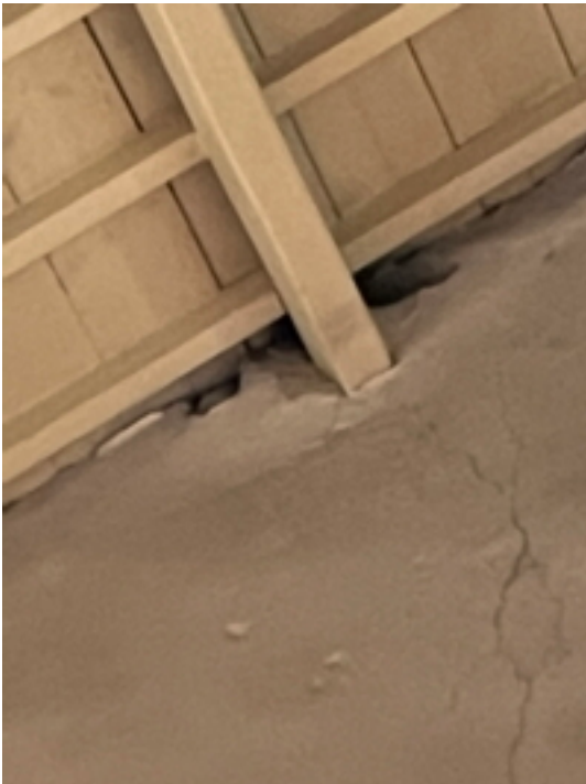
Nave North East End High Level Loose and Cracked Plasterwork
