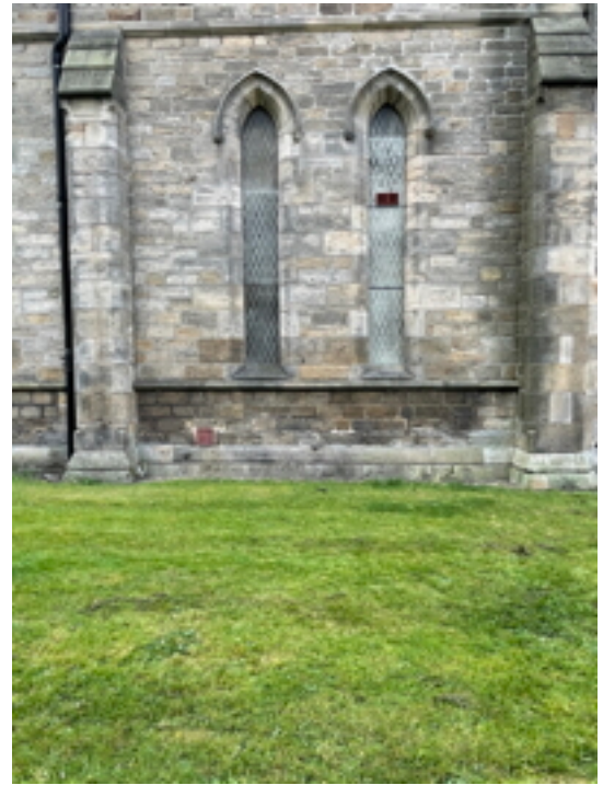
W3 and 4 Gallery Staircase Vandalite Security Glazing
