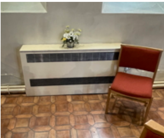
Typical Nave Convector
