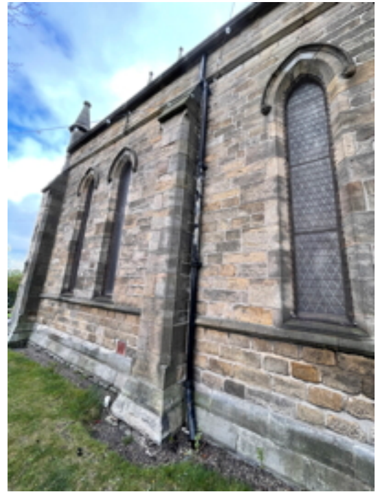
UPVC Rainwater Pipe North Elevation
