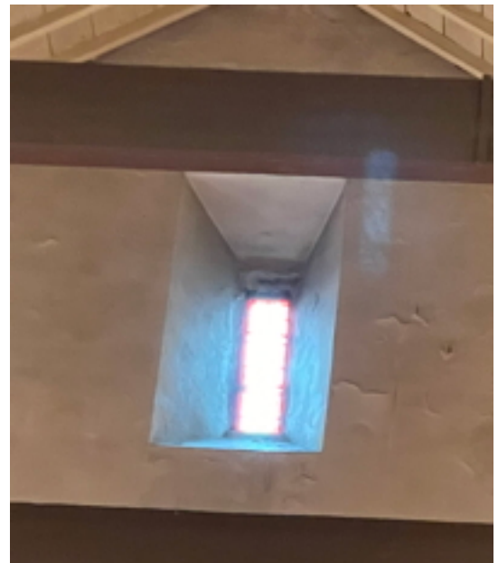
Nave East Gable Window Clear and Coloured Glass with Lead Cames
