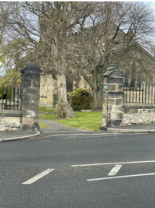
East Wall Piers
