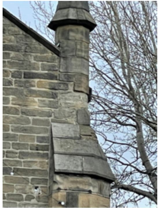
Nave South West Pinnacle base Deteriorating Stonework
