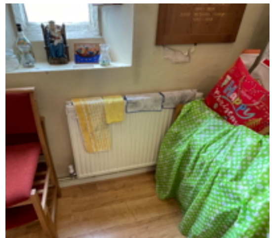
Typical Meeting Room Radiator
