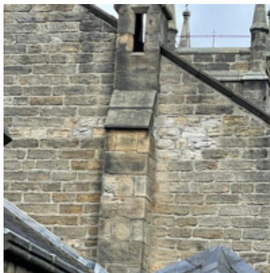
Nave North East Elevation Deteriorating Stonework
