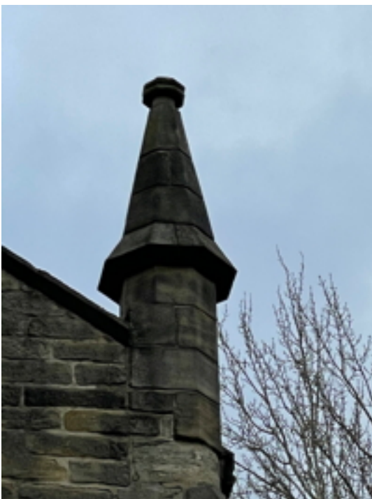
South West Corner Pinnacles
