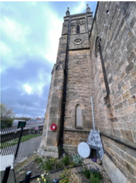
Cast Iron Rainwater Pipe Tower South Elevation
