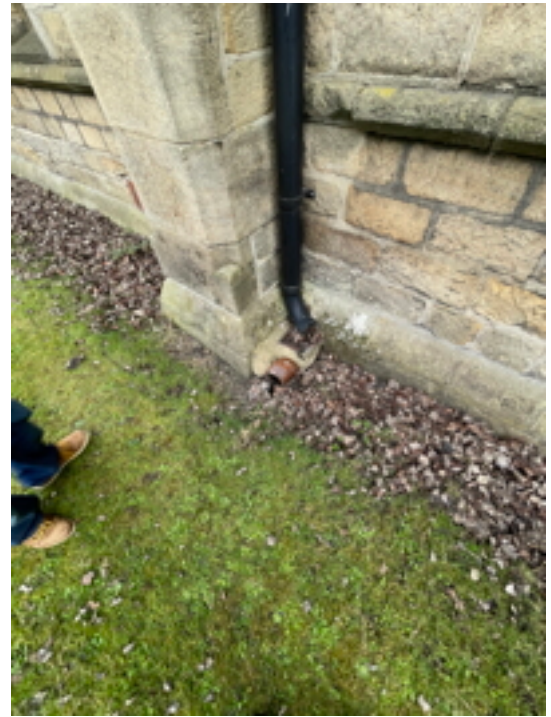
Rainwater Missing Gully North Elevation
