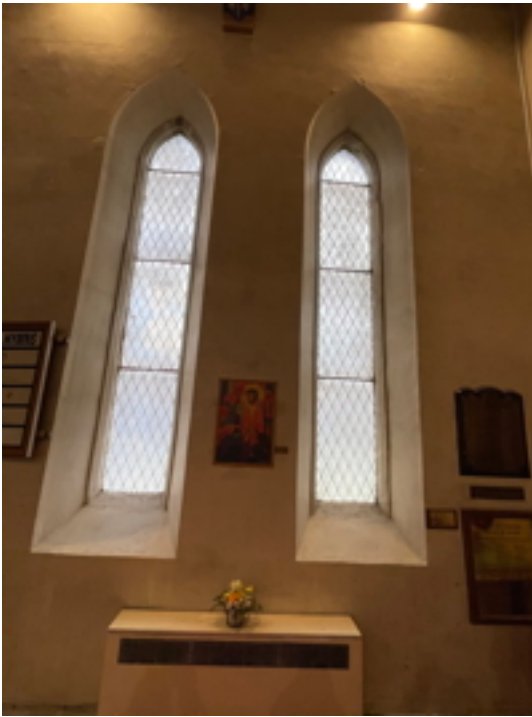
W9 and 10 Nave North East Vandalite Security Glazing
