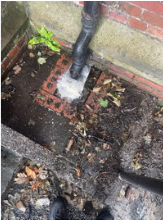
Typical Blocked Gully
