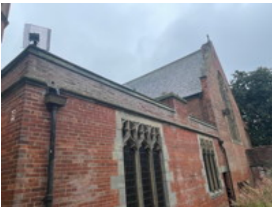
South East Corner Deteriorating Brickwork
