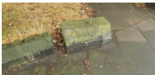
Displaced Plinth Stone
