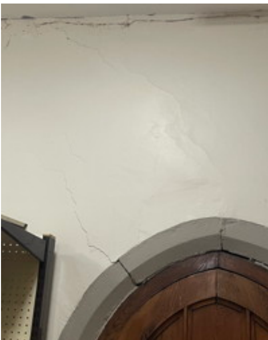
Cracking over the doorway to the South Porch
