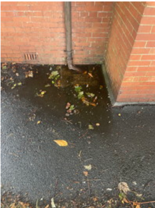
Blocked North Elevation East End Gully
