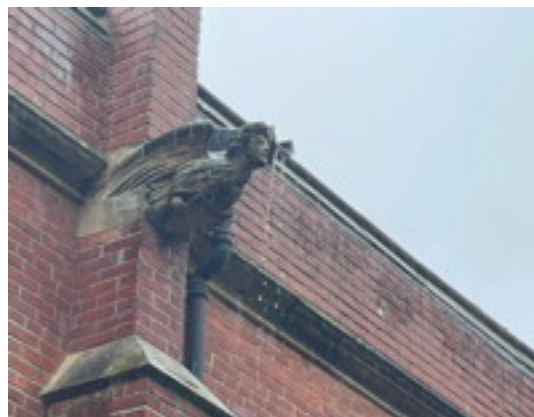
Blocked Parapet Outfall
