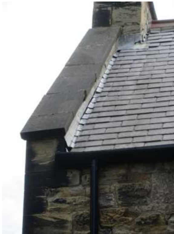
W side of Organ Chamber – lead flashings pulled apart show the gable has moved away from the slate roof
