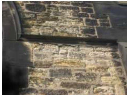
stone decay next to over-hard pointing under the E window and under the string course near the N buttress
