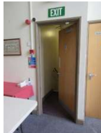
Door at top of stair binds on floor
