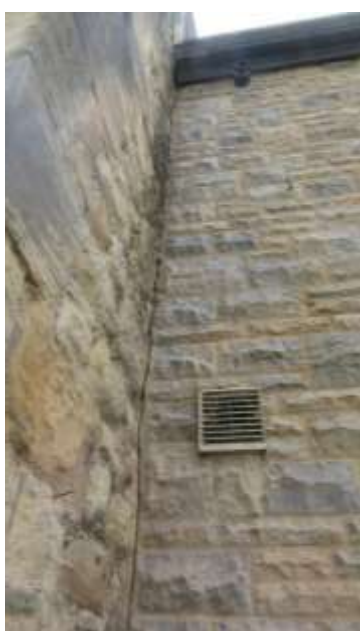
Cracked joint at N side
