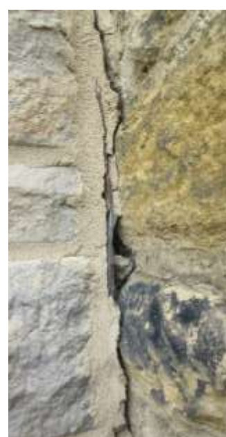
Cracked joint at S side
