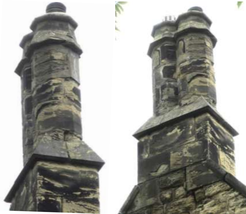
From NW – two N flue stones decaying and hole and open joint between sloped cap on base
