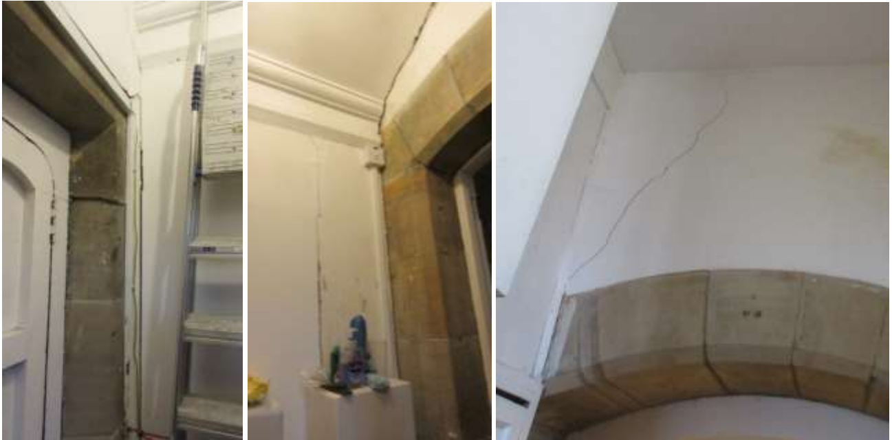
Hairline crack at Organ side of arch to N Porch (para 10)
