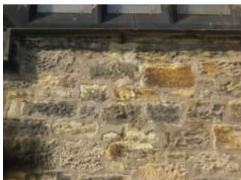
stone decay next to over-hard pointing under the E window and under the string course near the N buttress
