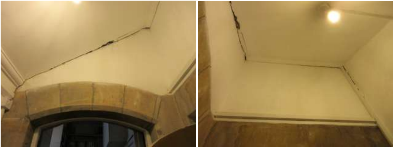
Cracked plaster at all sides of the N Porch
