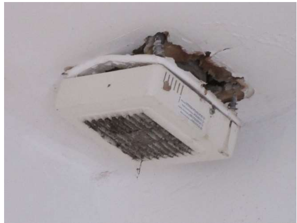
Vent pipe through void over wc off Kitchen and its dropped fan
