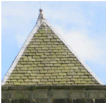
Slate missing from Tower N side
