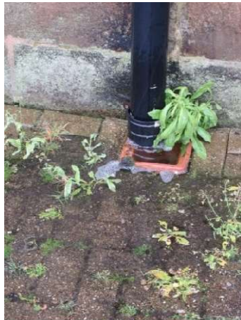
In rain N Nave W gully spills across the public pavement
