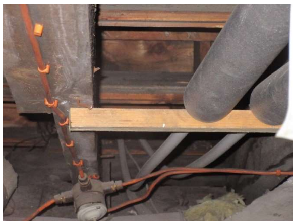
Heating pipework under Gallery part insulated
