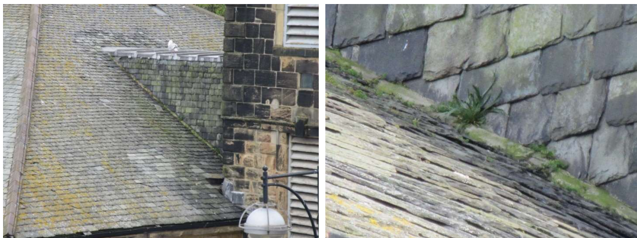
plants in cracked mortar fillet N of the tunnel between Tower and Nave roof and a slipped slate lies on lower slates
