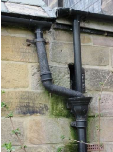
Song Room NE - 2019 photos repeated because now hidden by growth - Misaligned pipe misses the hopper
