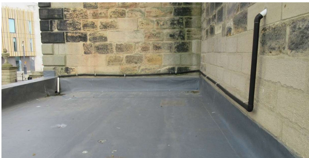
Kitchen roof with condensate drain from boilers now extended to outlet sump
