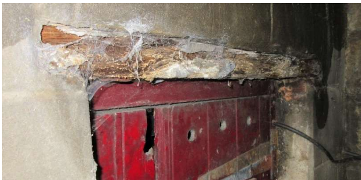
Decaying Lintel at Blower door
