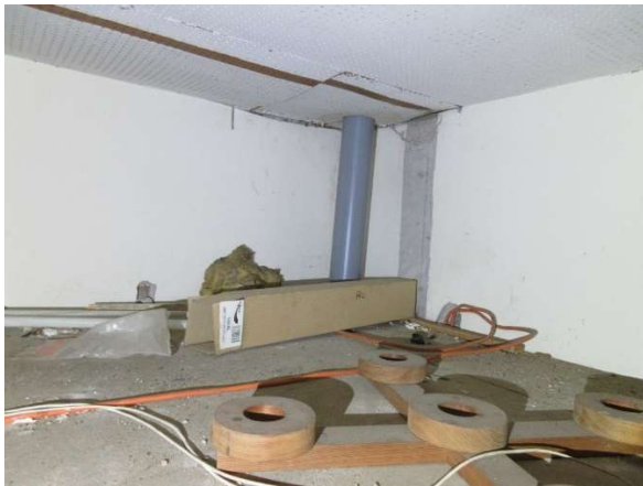
Vent pipe through void over wc off Kitchen and its dropped fan
