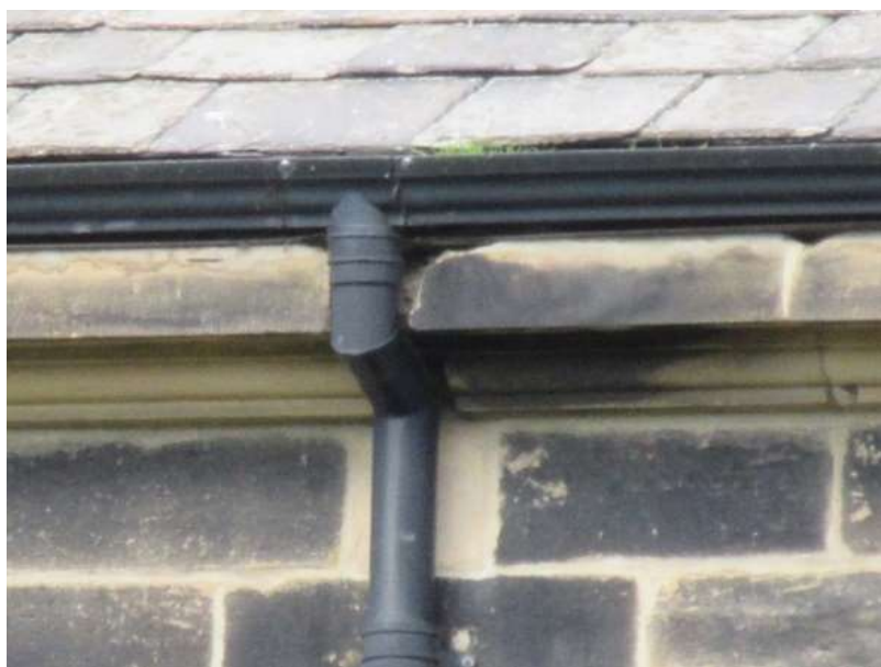
Typical Nave gutter - N gutter E outlet
