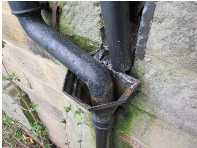
Song Room NE - 2019 photos repeated because now hidden by growth - Misaligned pipe misses the hopper
