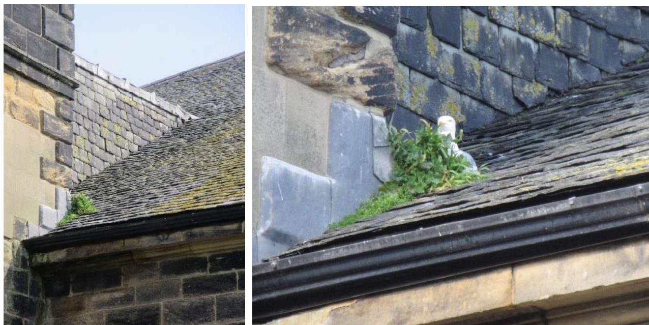
plants in cracked mortar fillet N of the tunnel between Tower and Nave roof and a slipped slate lies on lower slates
