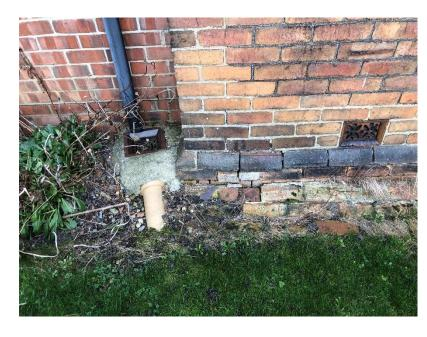
P12 (5958): Plinth brickwork displacement
