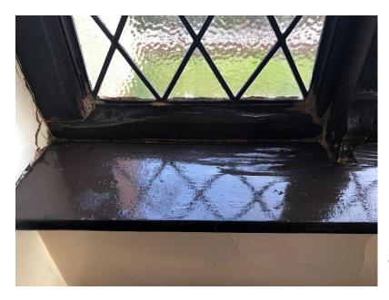
P1 (5806): Wet rot to window frame and sill
