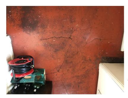
P8 (5856): Vestry floor cracking
