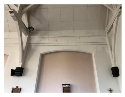
P2 (5818): Eaves paint flaking (west/nave); ceiling tiles composition TBC (possible asbestos?)
