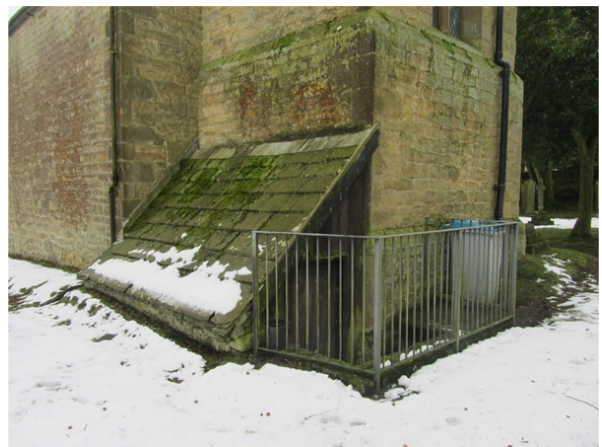
Boiler House (6.2, 6.8 and 12.3)
