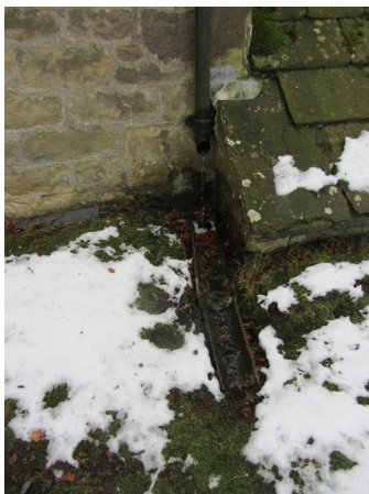
Drainage by Nave north downpipe (6.2)
