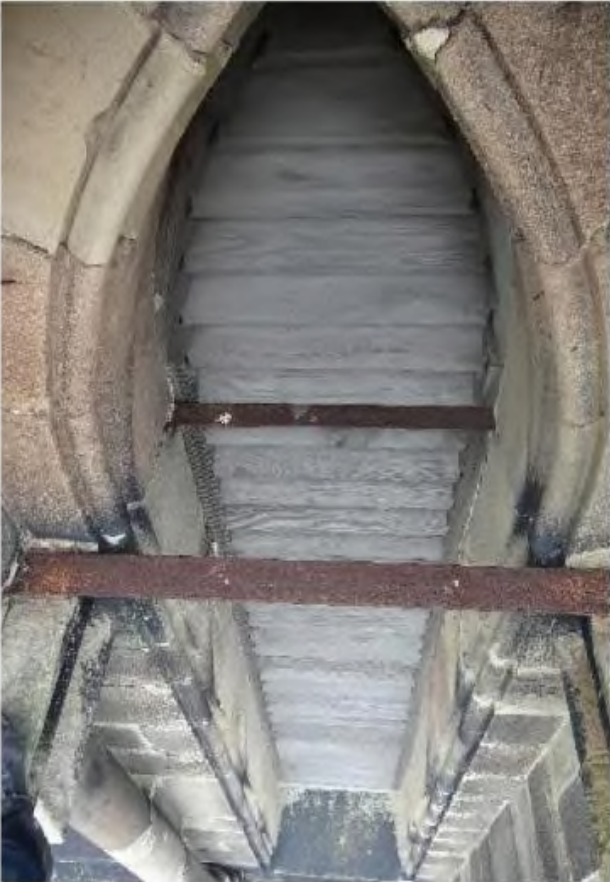
Examples of uppermost stringcourse (South Face).
