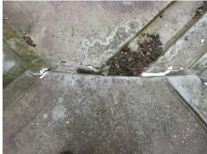
30. The Boiler room and Kitchen flat roofs also changed from felt to glass reinforced plastic with very slight falls to two internal outlets, seems sound.
