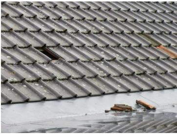
23. The Hall tiles are black in better condition with little moss. Some black and red replacements. 12 glass tiles over the upper wcs and stair. Wire clipped bottom course of tiles over the flat roofed dormer. At the E offshot a rubber valley lining at N, lead at S.
