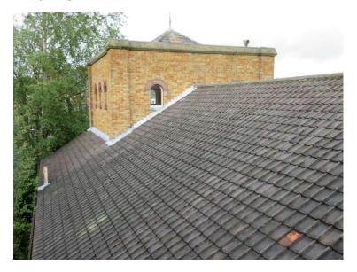
19. Round ridge and hip tiles. Mortared verges and the valleys lead lined except where substitute fitted at E after theft.
