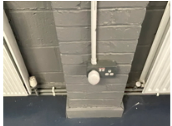
Typical Hall Socket
