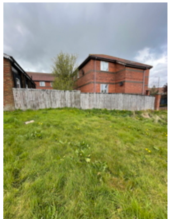
South West Boundary Fencing
