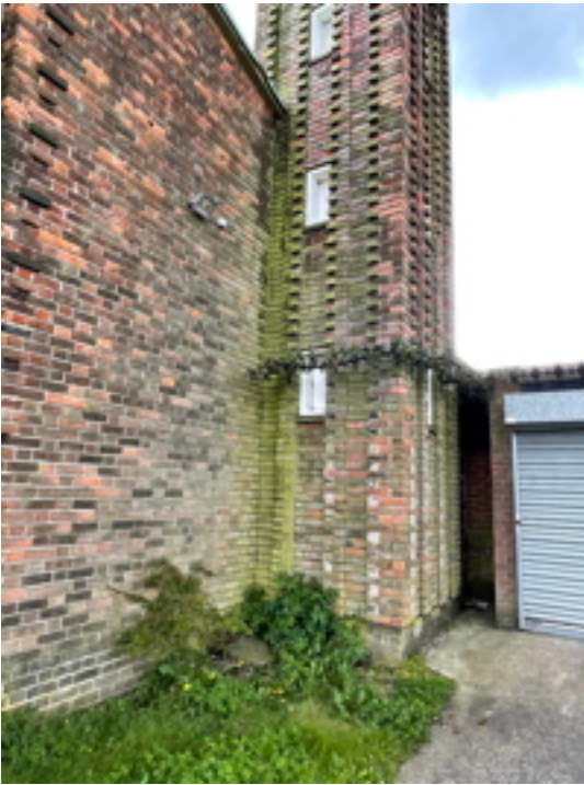
Tower North West Corner Bottom Section
