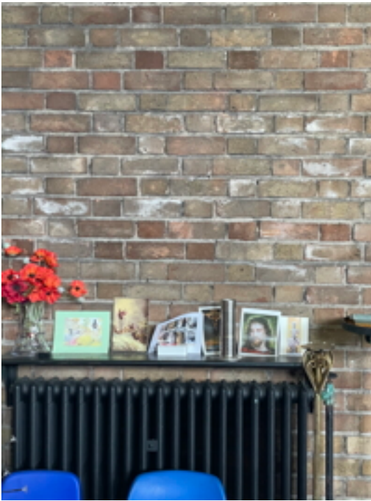
Salts to North West Corner Brickwork
