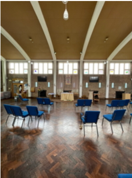
Herringbone Flooring to Nave
