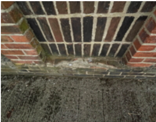
Sanctuary North West Elevation Broken Creasing Tiles
