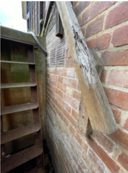
Boiler Room Ladder and Handrail
