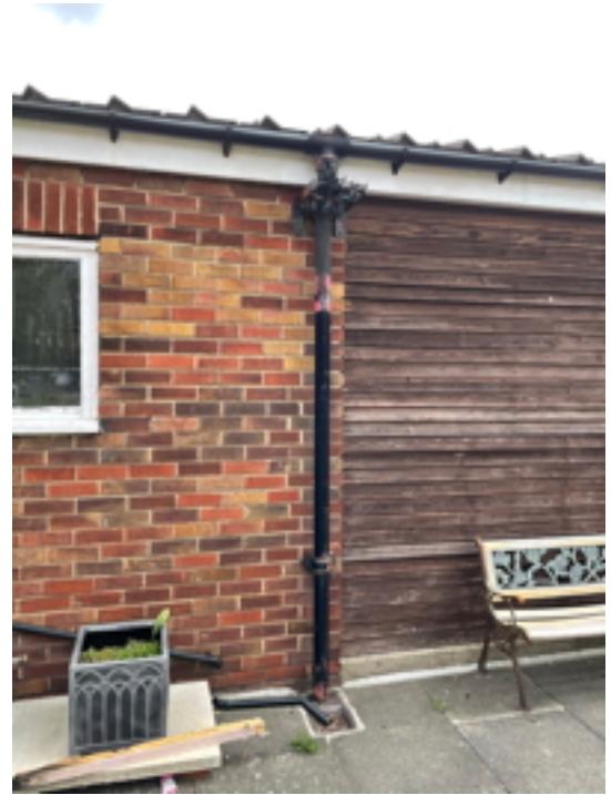
Hall East Rainwater Pipe
