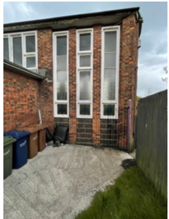
Sanctuary South Elevation
