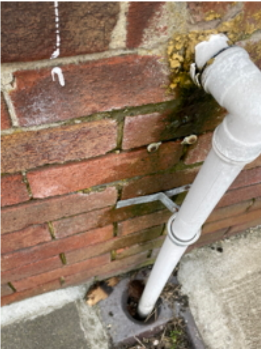
Leaking Waste Pipe
