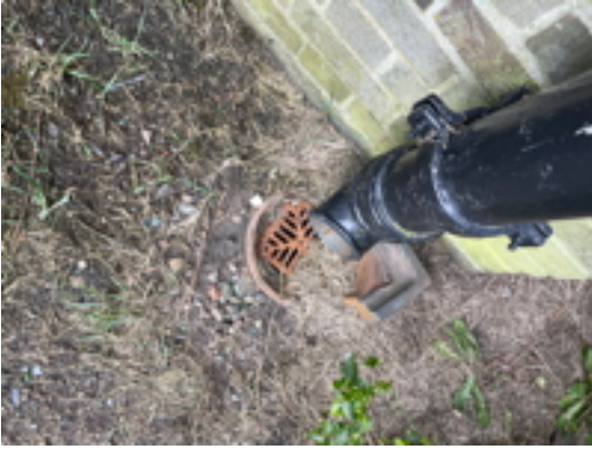
Partly Blocked Gully
