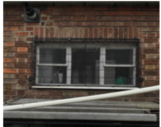
South Elevation Church Kitchen Window
