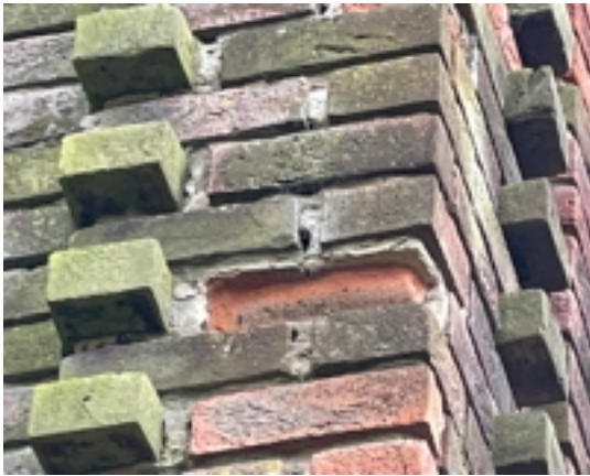
Hall West North West Corner Spalling Brickwork
