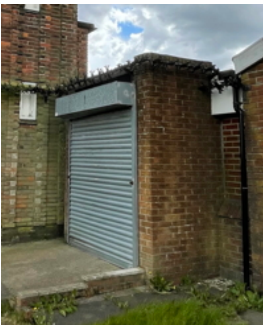
Hall Link Lobby North Elevation Roller Shutter
