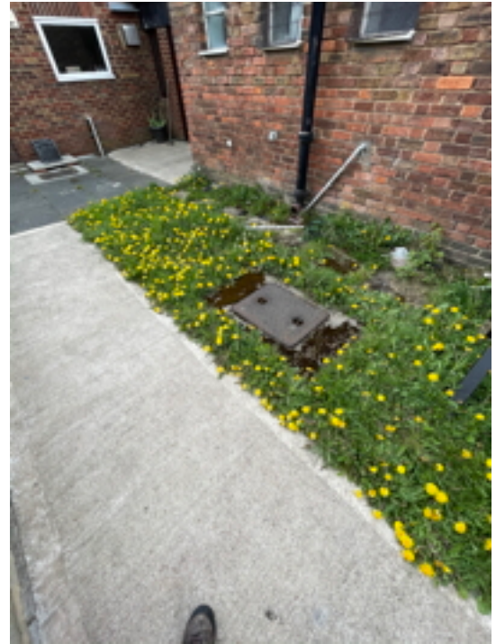
South Elevation Inspection Chambers
