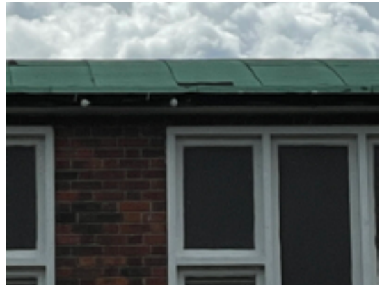
Church Roof Lift Felt North Elevation
