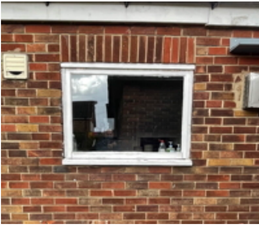
Hall Kitchen East Elevation Window
