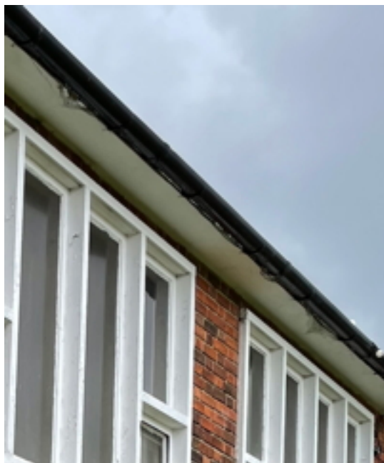
Nave North Eaves Spalling Concrete
