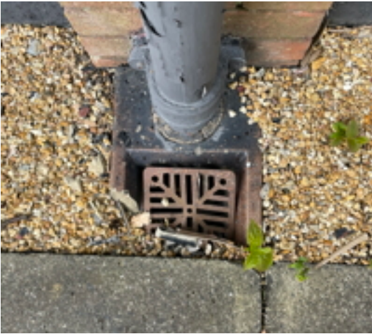
Partly Broken Gully
