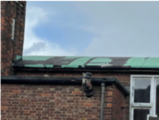
Church Roof Patching South Elevation
