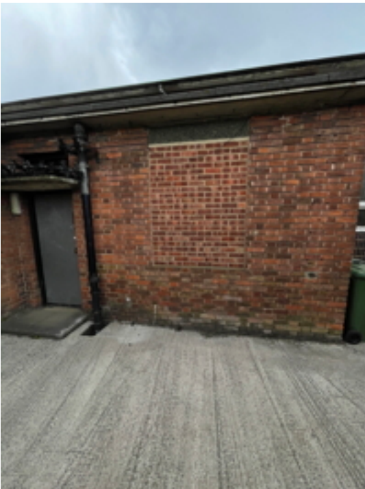
Vicar's Vestry Blocked-up South Elevation Window
