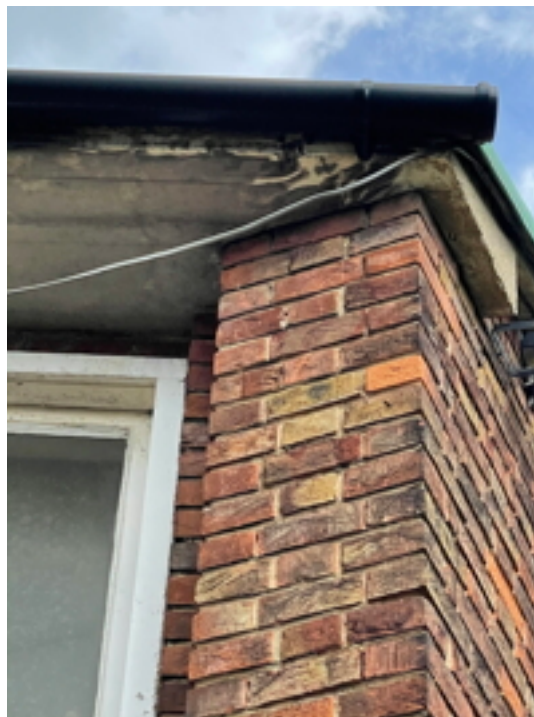
Nave South East Eaves Probably Spalling Concrete
