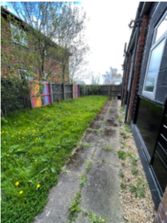
West Boundary Fencing
