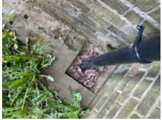
Partly Blocked Gully
