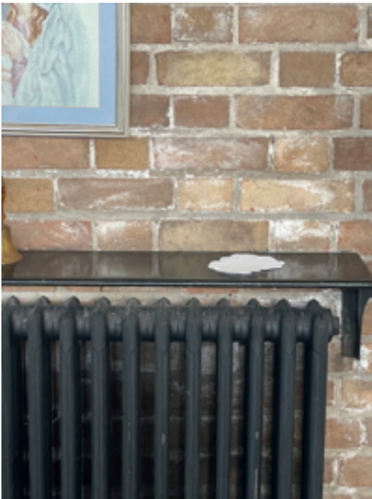
Salts to North Wall, East End Brickwork
