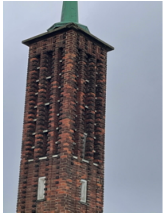
Tower North West Corner Top Section
