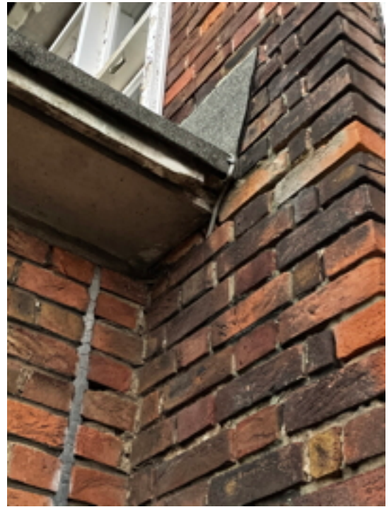
Vicar's Vestry South East Eaves Spalling Concrete
