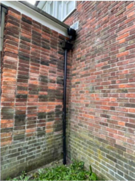
North Porch Rainwater Pipe
