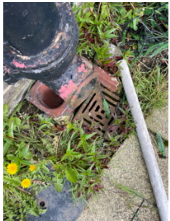
Partly Broken Gully
