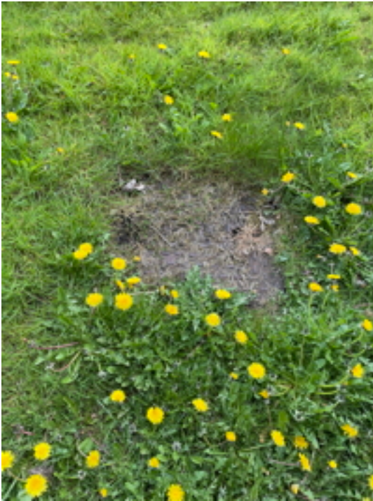
West Elevation Inspection Chamber
