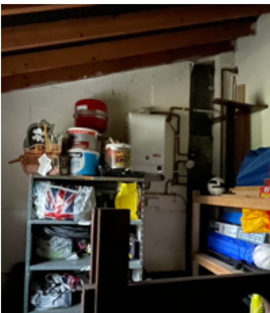
Hall Store Looking South
