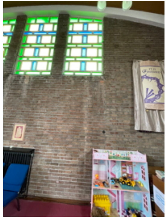
Staining to Brickwork Below West Window
