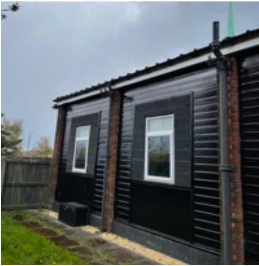
Hall West Elevation Timber and Painted Blockwork Infill
