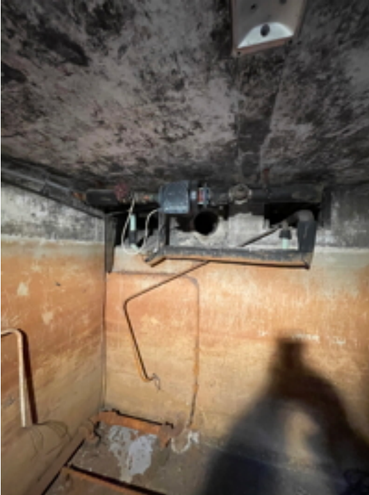
Boiler Room with Pump
