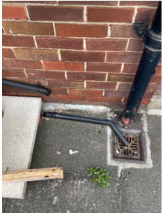
Broken Waste Pipe
