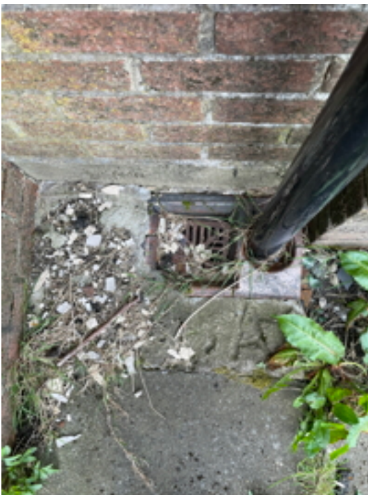
Partly Blocked Gully
