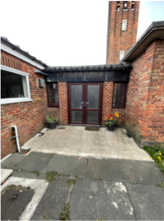
Hall Lobby Link Fascia Requires Decoration
