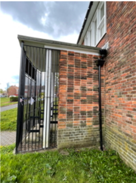
North Porch West Elevation
