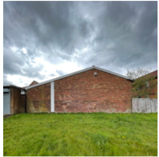
Hall North Elevation
