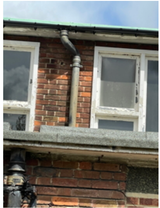
Nave South Rainwater Pipe
