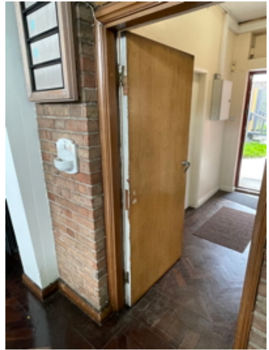
South Lobby Door
