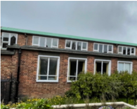
South Elevation Nave and Choir Vestry/Meeting Room Windows
