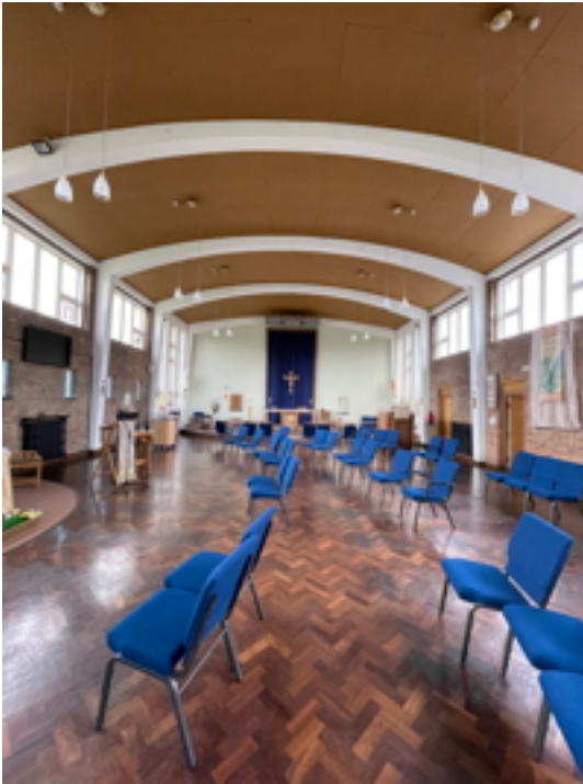
Roof Looking East
