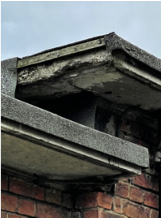
Choir Vestry/Meeting Room South West Eaves Spalling Concrete
