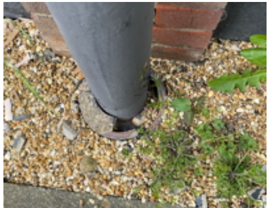
Missing Concrete Haunching
