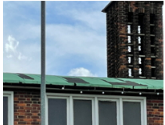
Church Roof Patching North Elevation
