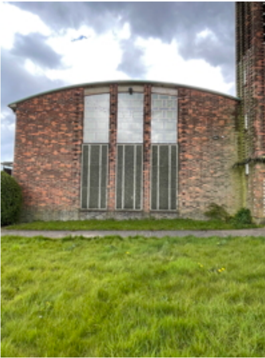
Nave West Elevation
