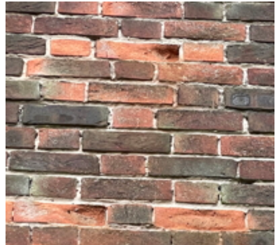
Nave West North West Elevation Spalling Brickwork
