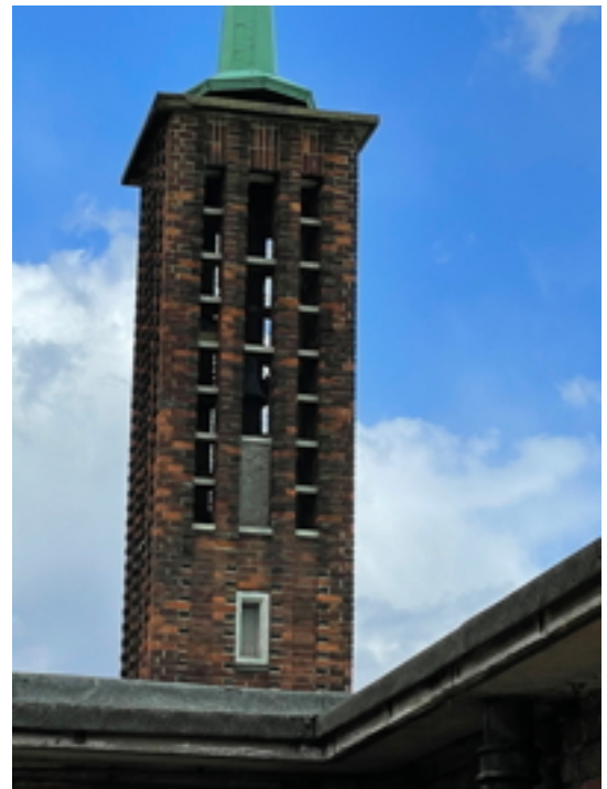
Tower Brickwork Openings
