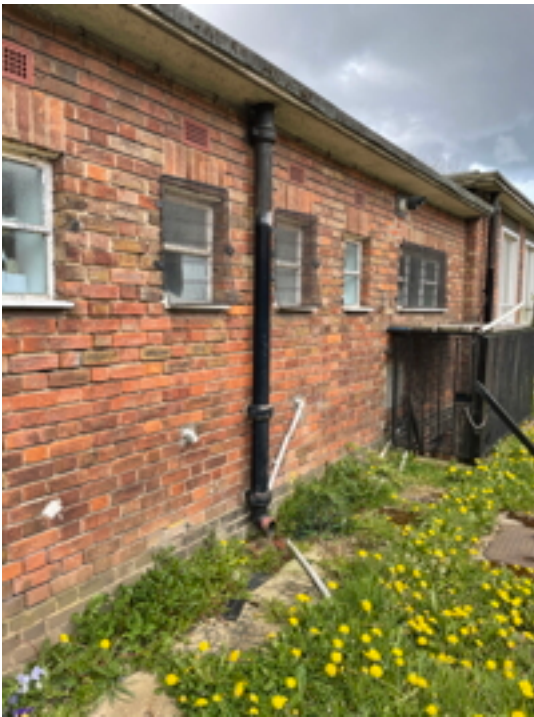
WCs South Rainwater Pipe
