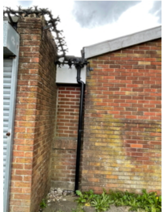
Hall Lobby Link North Rainwater Pipe
