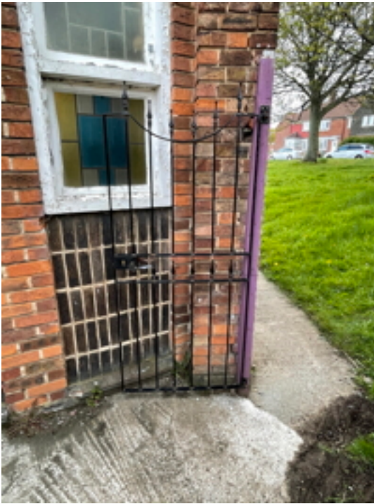
South East Corner Gate
