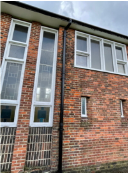
Nave North East Rainwater Pipe
