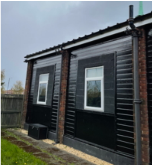
Hall West Elevation Windows
