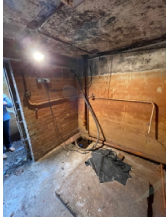
Boiler Room with Sump
