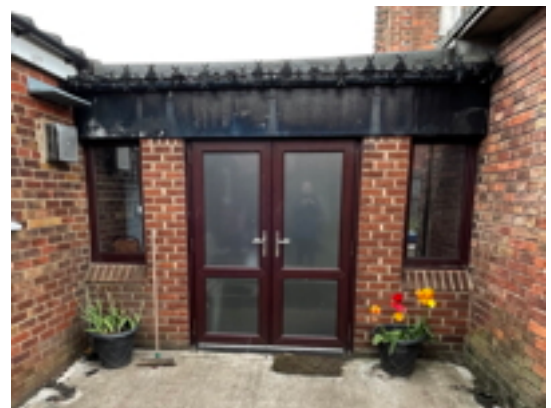
Hall Link Lobby South Elevation Windows and Doors
