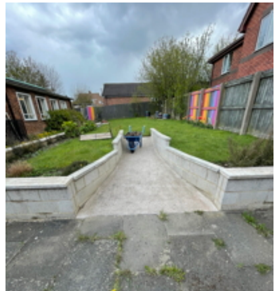
Raised Garden to South
