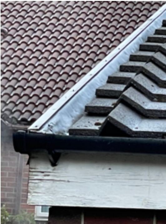
Hall South East Lead Gutter and Rotten Eaves
