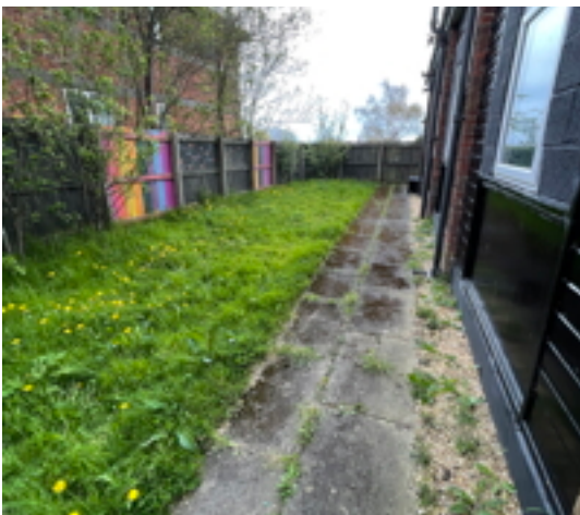
Grass and Paving to Hall West Elevation
