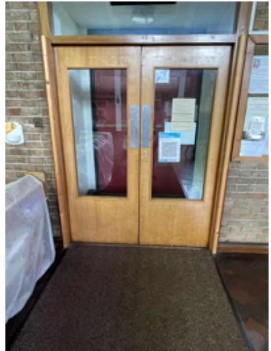
North Porch Doors
