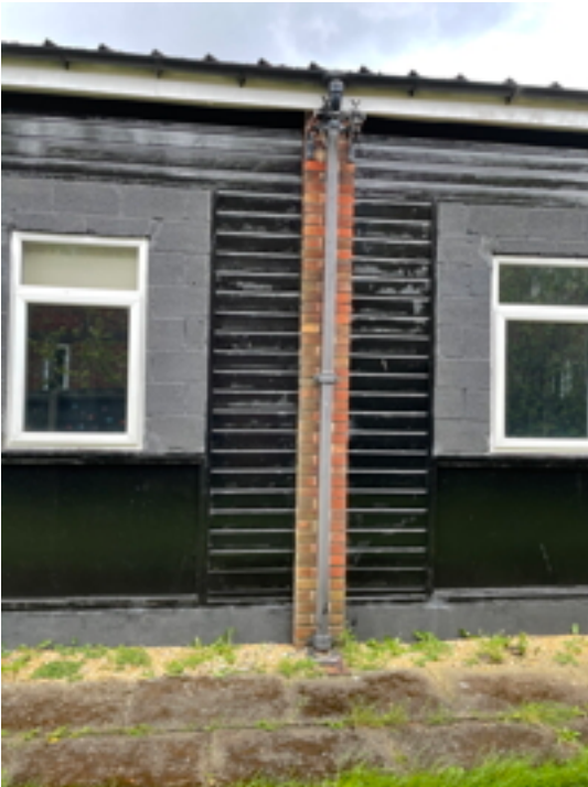
Hall West Rainwater Pipe
