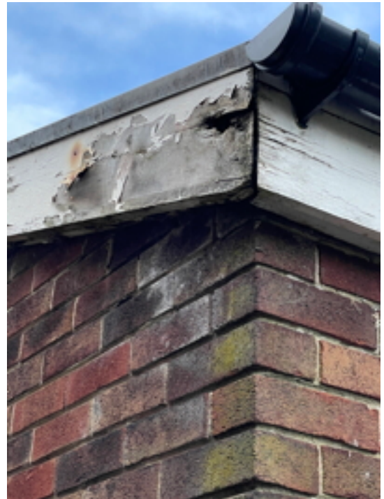
Hall South East Rotten Verge
