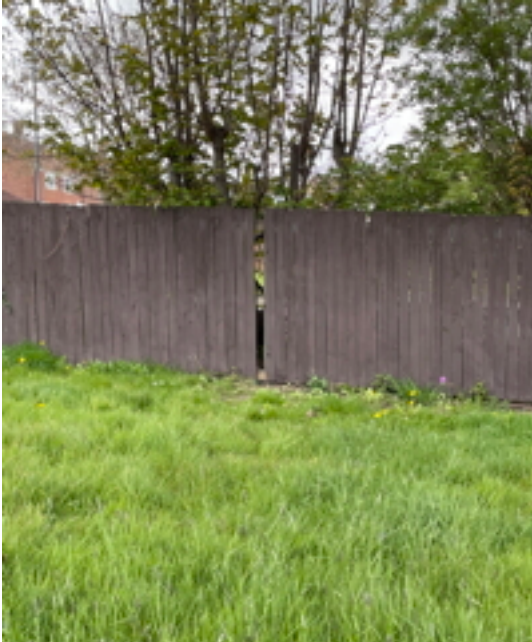
South East Boundary Fencing
