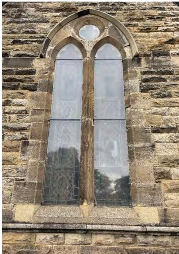
W19 – General overview of window.
