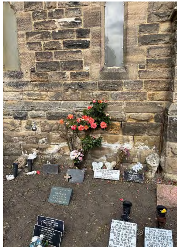
Memorials to base of church walls to South and West elevations.
