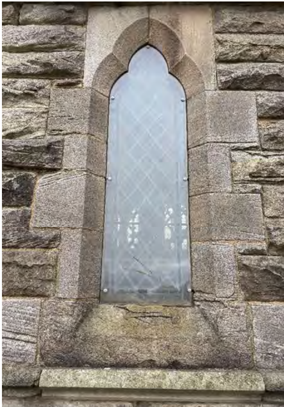
W11 – General overview of window.
