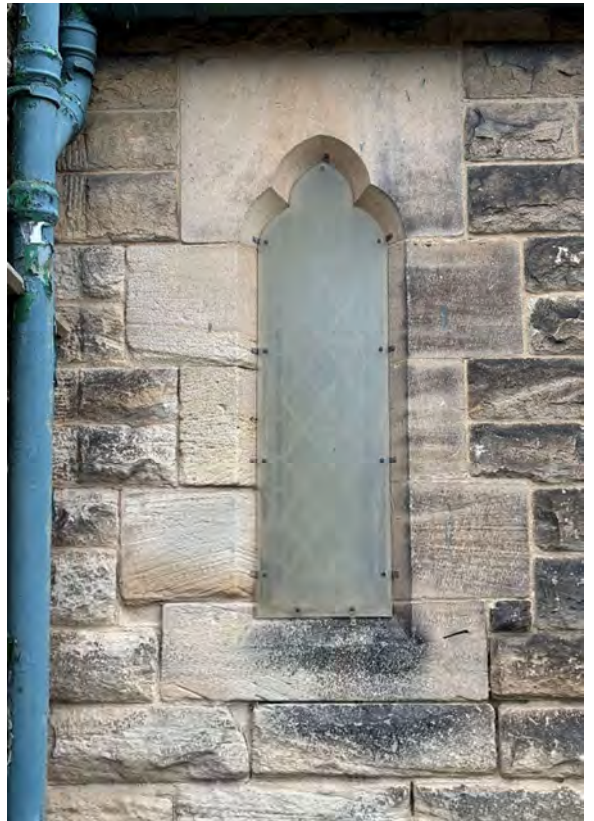
W26 – General overview of window. Some discolouration to external protection.
