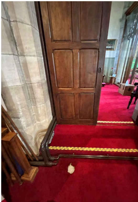
Patch of carpet missing upon approach to Memorial Chapel
