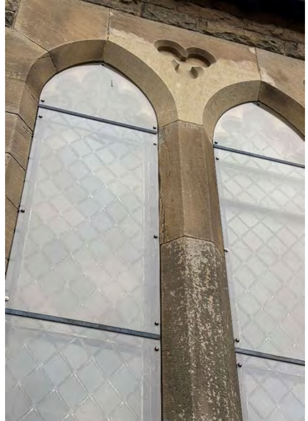
W5 – Some delamination to upper left mullion.
