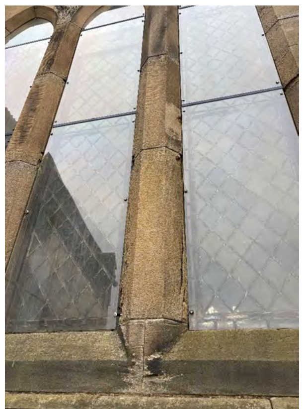
W5 – Some delamination to upper left mullion.
