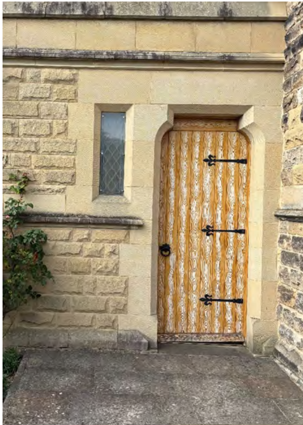
Overview of accessible entrance door.
