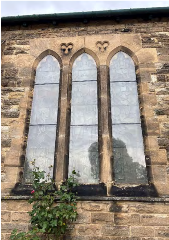
W21 – General overview of window.
