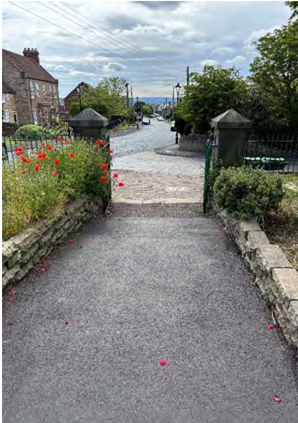
Approach to church – accessible route. However paving to entrance is uneven.
