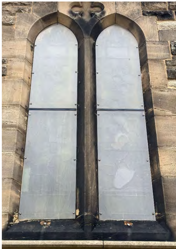
W15 – General overview of window.
