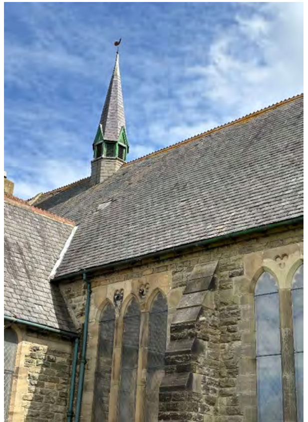
Overview of areas of North Roof
