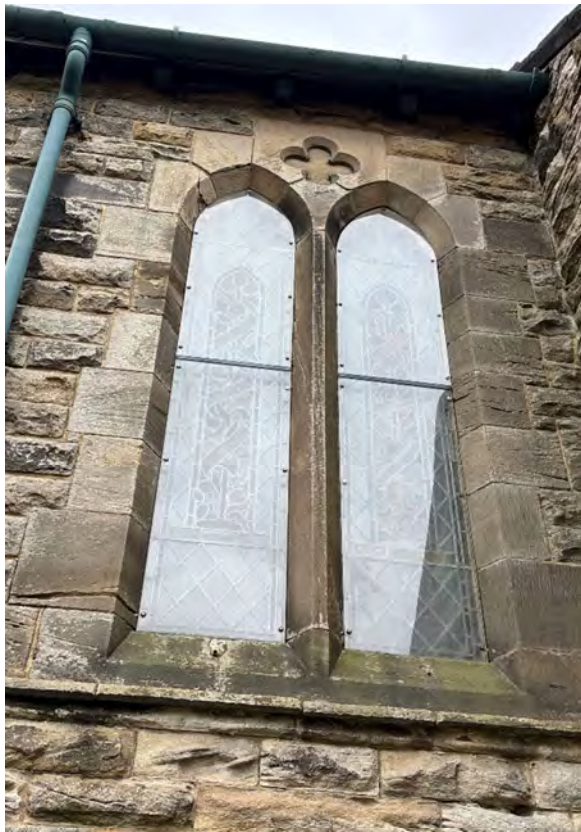
W12a – General overview of window.
