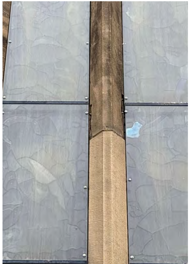
W2 – Weathering of stone around central mullion.
