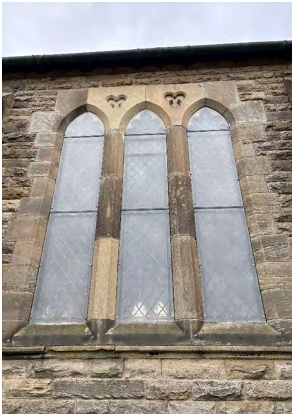
W4 – General overview of window.
