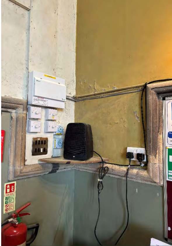
Evidence of flaking yellow paint to West Wall
