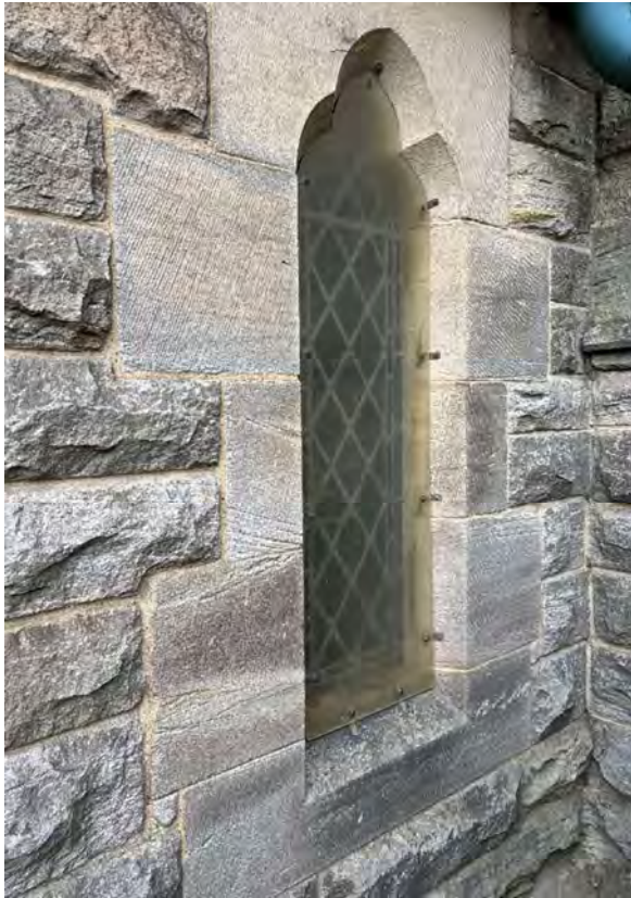
W23 – General overview of window. Some discolouration to external protection.
