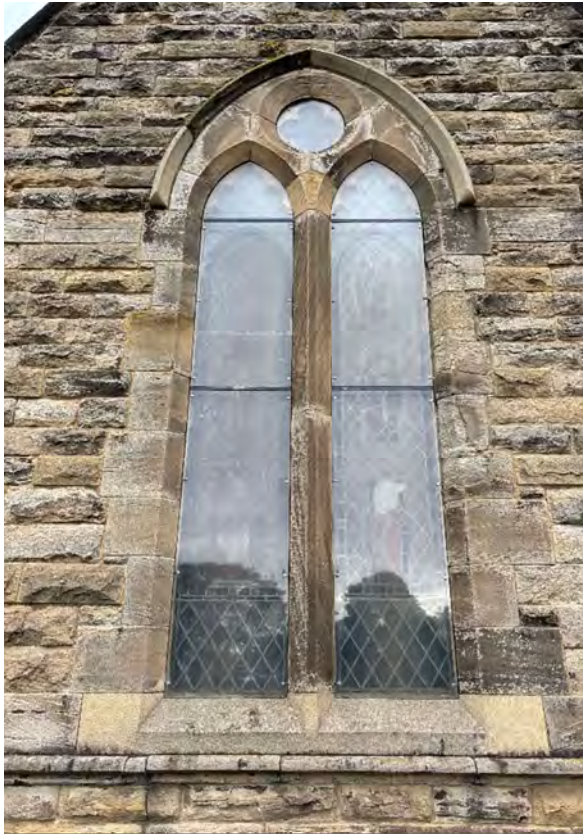
W18 – General overview of window.
