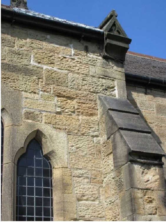
Slight stone decay above R side of E window in the S Nave
