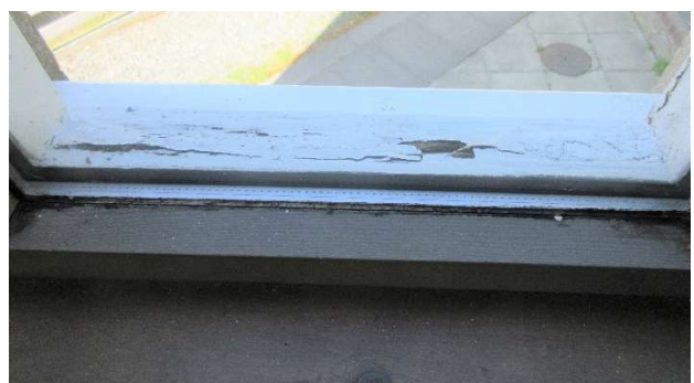
First floor N
