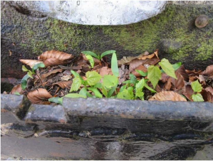
Hopper at N valley gutter before clearance at the inspection
