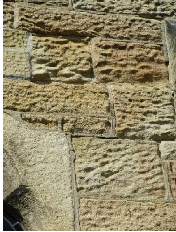
Slight stone decay above R side of E window in the S Nave
