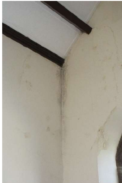
Baptistry NW corner
