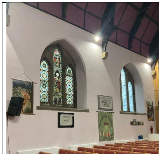
Southern Wall in Nave
