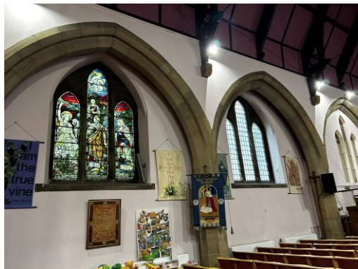
Northern Wall in Nave
