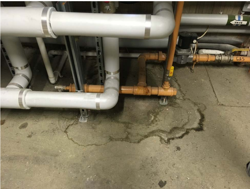
Photo 22 Leak onto chipboard floor below boiler
