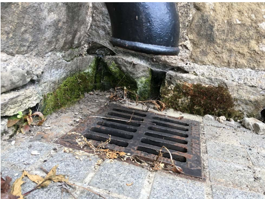
Photo 7 Rainwater runs into building at gullies south side
