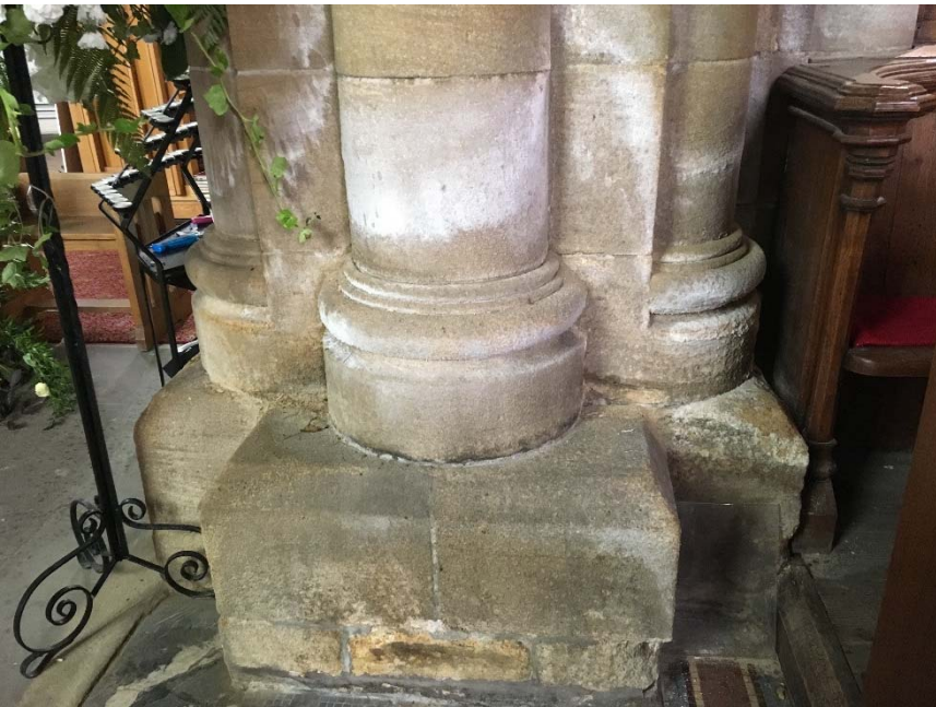
Photo 19 Efflorescence on north Chancel arch pier
