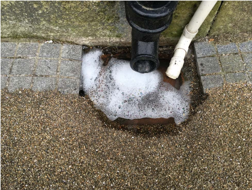
Photo 8 Blocked gully to kitchen seeps below building
