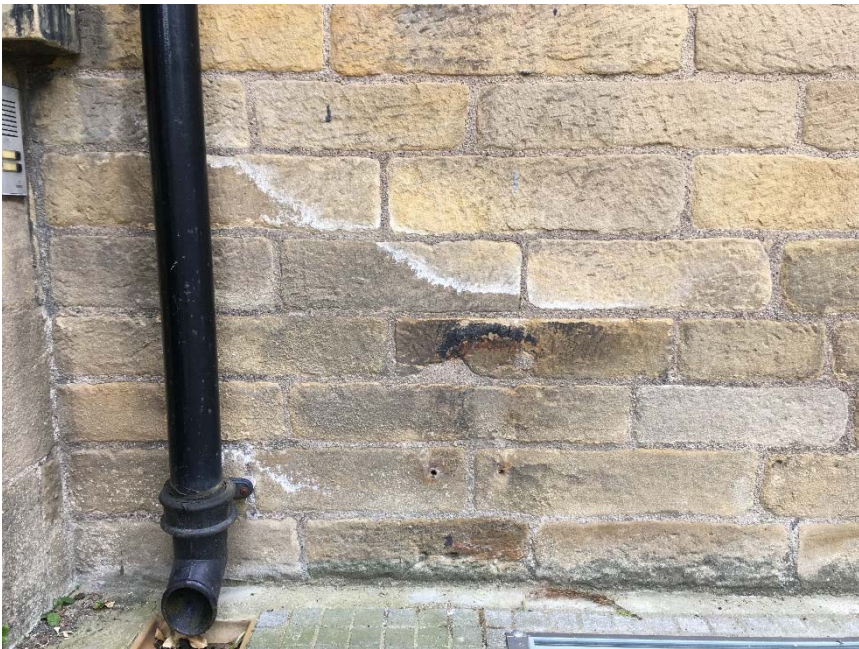
Photo 9 Efflorescence on external North Transept wall
