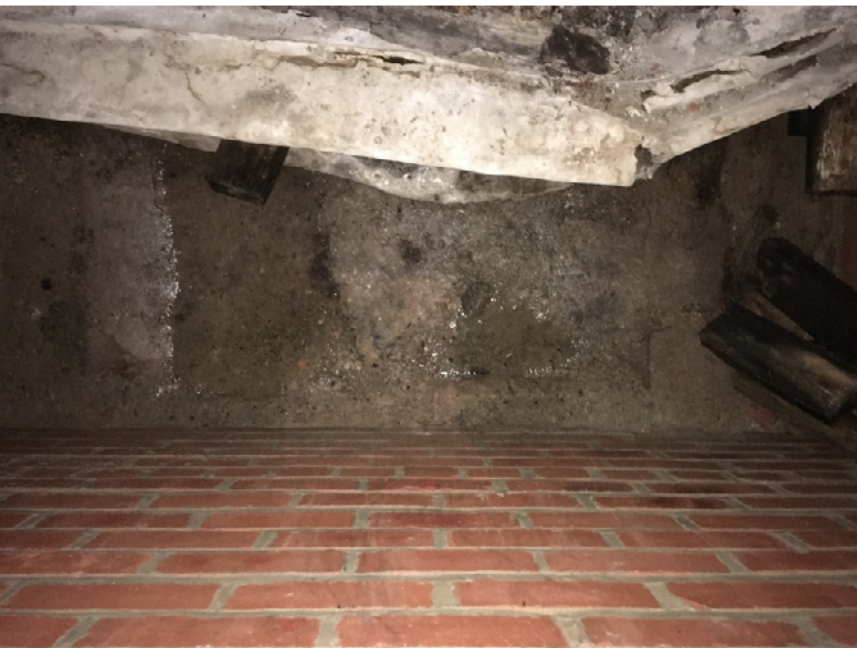
Photo 20 Water standing in chamber below North Transept floor
