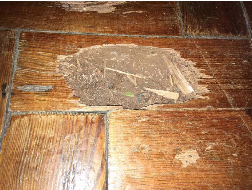
Photo 21 Rot in woodblock flooring
