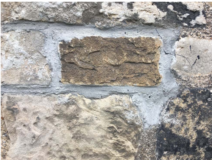
Photo 13 Recent infill stones to former flues in hard cement mortar
