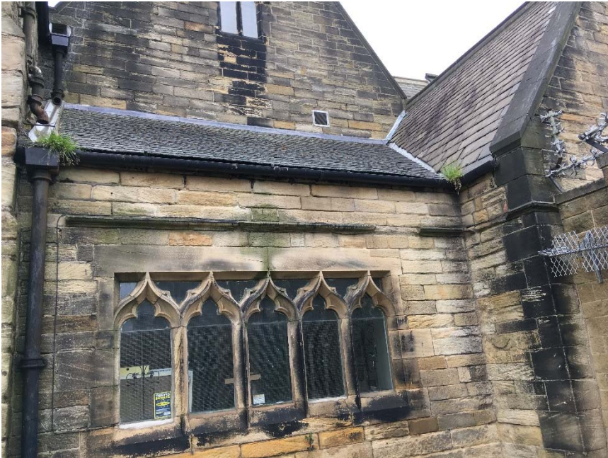
Photo 5 Debris in gutter and eroded mortar and window cills on Vestry
