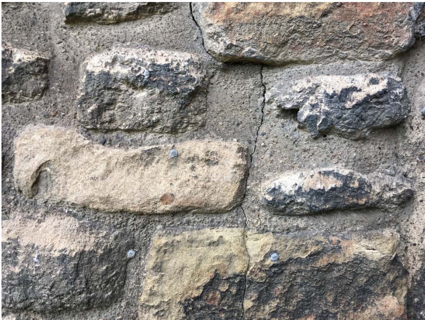
Photo 12 Cracking through wide gauged cement pointing on Tower
