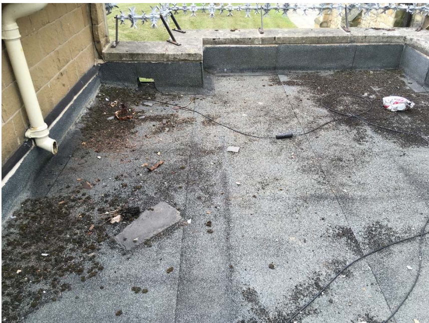
Photo 4 Slate and debris on Bake House link roof
