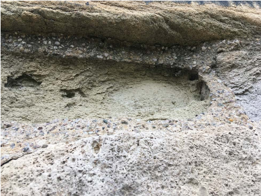
Photo 11 Localised stone decay in gauged cement pointing
