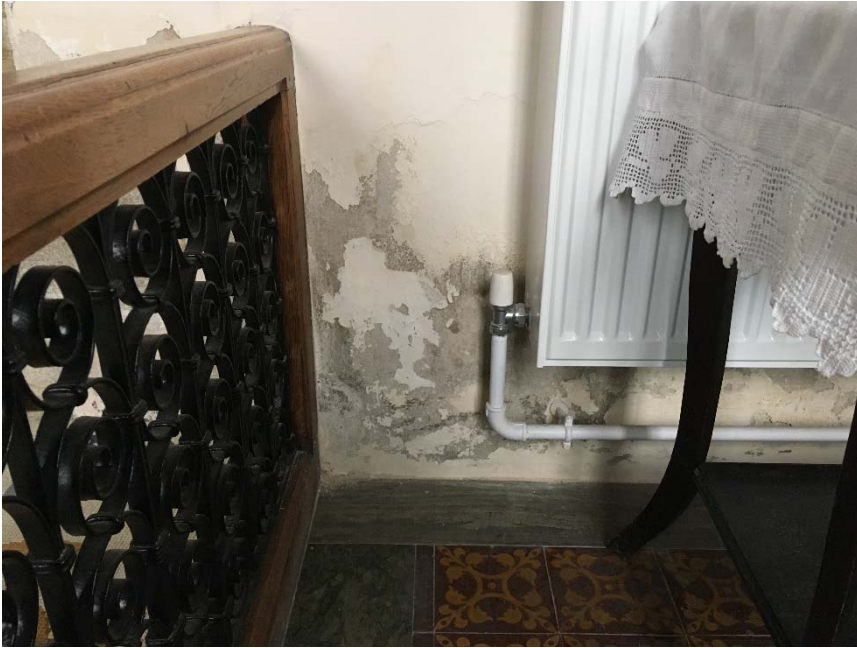
Photo 16 Plaster damage above raised floor in Sanctuary
