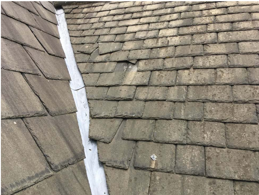
Photo 3 Slipped slates on North Transept valley roof
