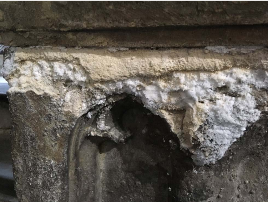
Photo 18 Efflorescence on tomb below Chancel screen
