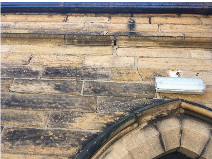
Photo 10 Movement and cement patch pointing over North vestry door
