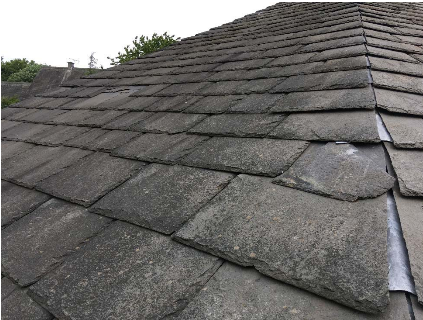
Photo 6 Slipped and missing slates on Bake House roof
