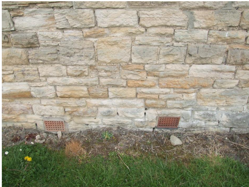
P2 (2352): South elevation nave, additional underfloor ventilation/mortar gaps
