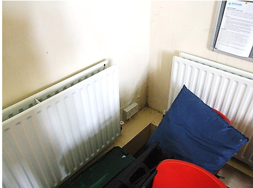
P5 (2458): Low level damp/salts to left hand side of south wall
