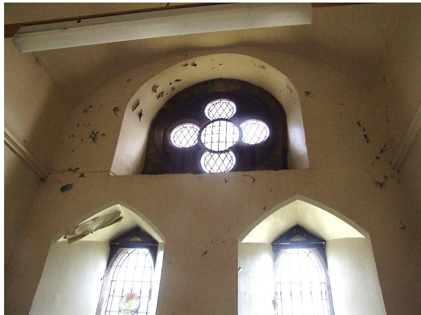
P8 (2476): Gabled vestry, peeling paint at high level
