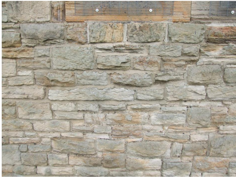
P1 (2353): South elevation nave, localised inappropriate pointing, exposed original mortar with coal
