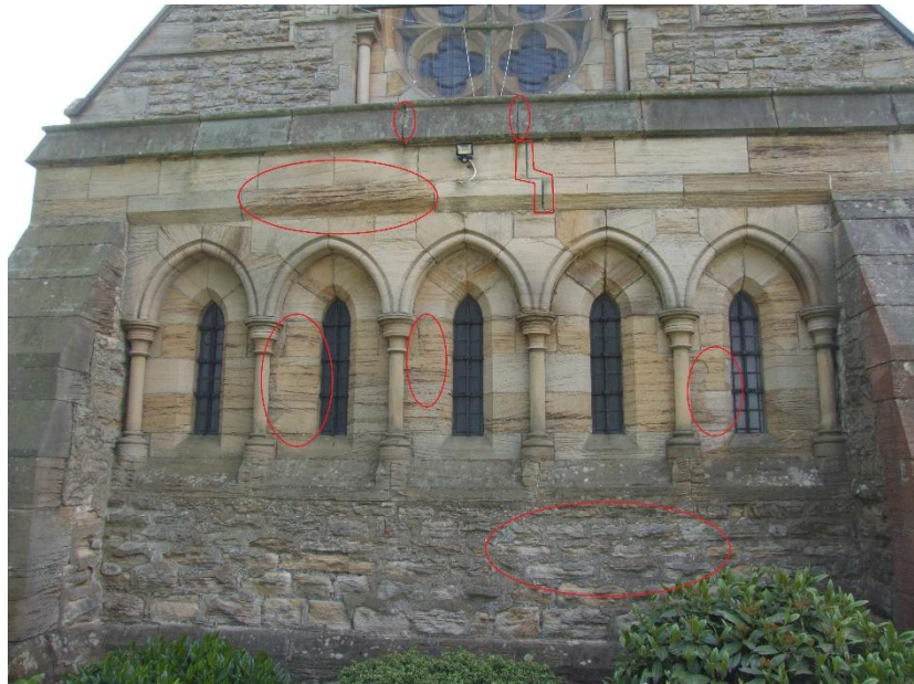
P11 (2537): Western porch, eroded stonework/open joints
