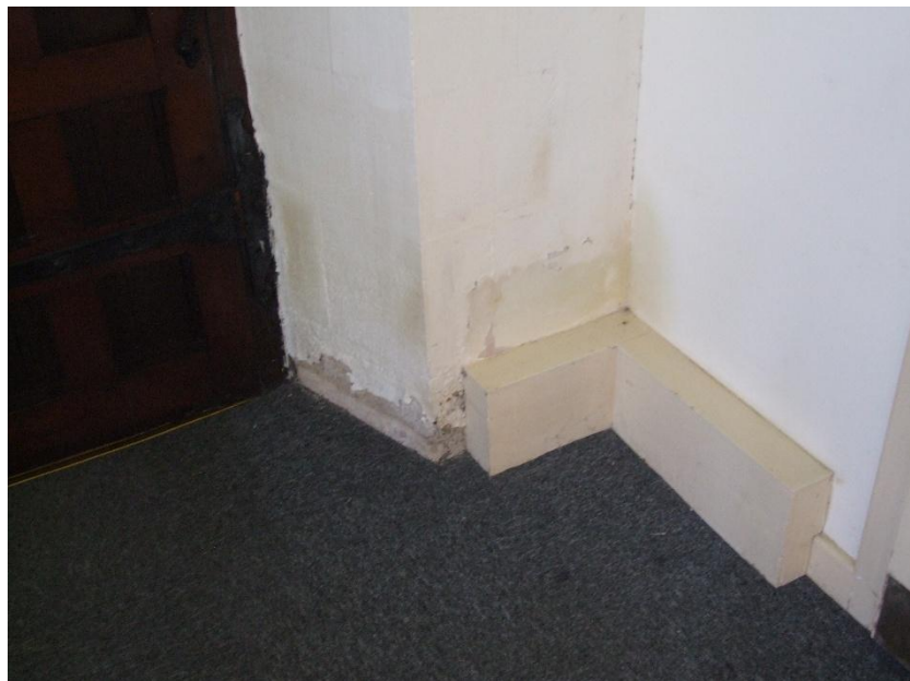
P4 (2453): Low level damp/salts to right hand side of entrance door
