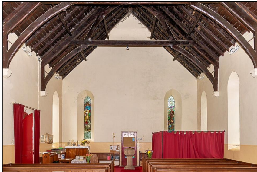
Nave looking west
