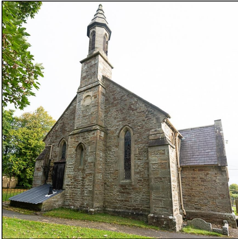
Nave and Porch: West Elevation
