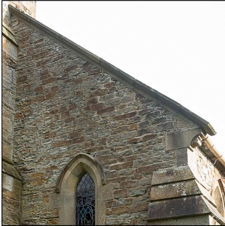
Fissures in the pointing are apparent above the hood moulding of W2 and in the masonry above.
