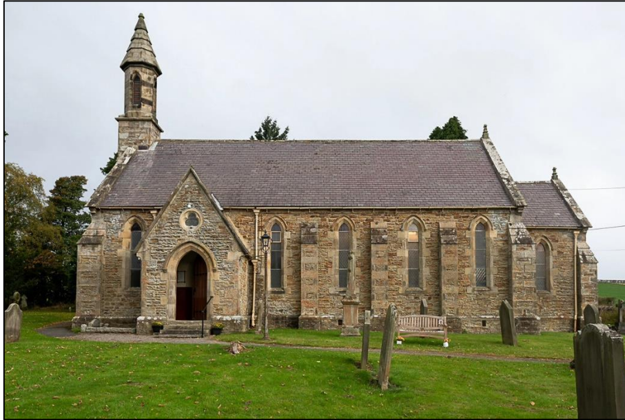
View from the south
