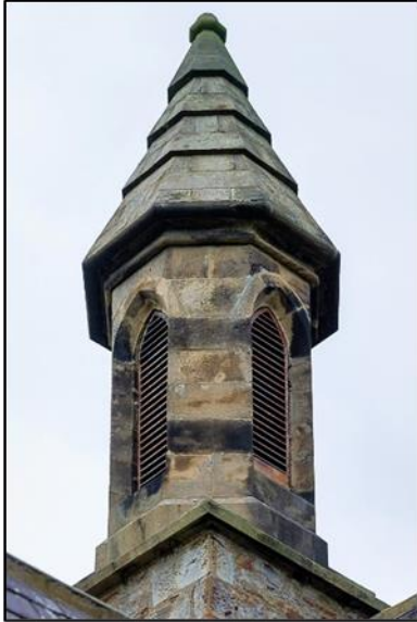
The bellcote from the southeast.
