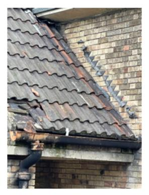
Typical cast iron gutter and rainwater pipe to pantiled roof
