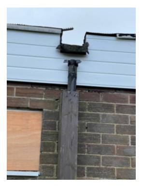
Missing hopper head to Hall west elevation
