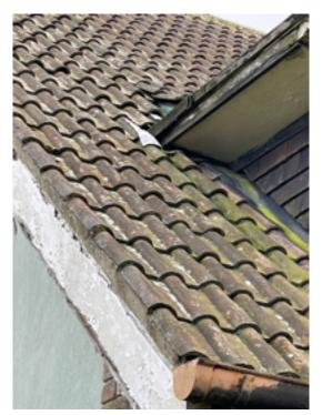
Possible leaking roof junction north east corner
