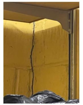
Cracking to Stage Area Store Blockwork
