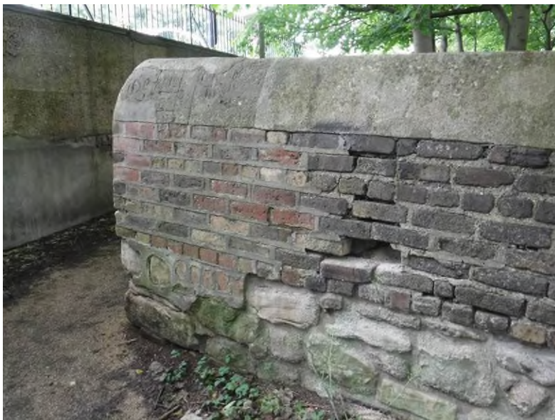
Brick erosion at sw corner. Pic from 2020
