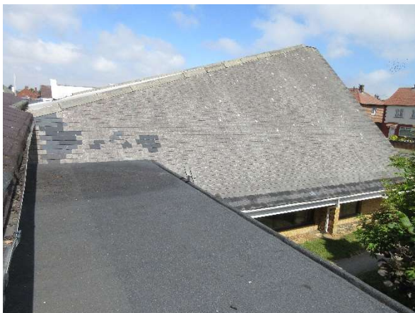
Narrow hidden gutter where the Church S slates butt to the flat roofed SE entry (para 16)
