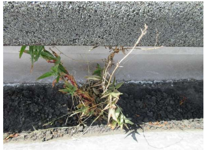
Plant in a gutter outlet before part clearance at the inspection
