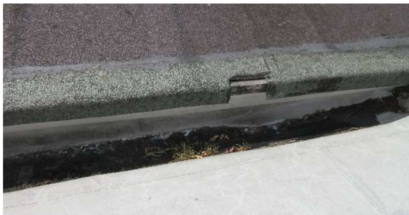
Missing felt at drip and plants in the silted box gutter
