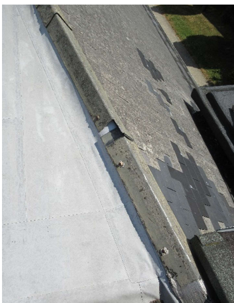
Gutter hidden under flat roof edge (para 16)
