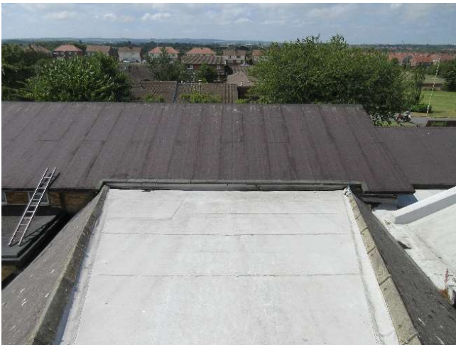
Internal gutter between Church and Hall
