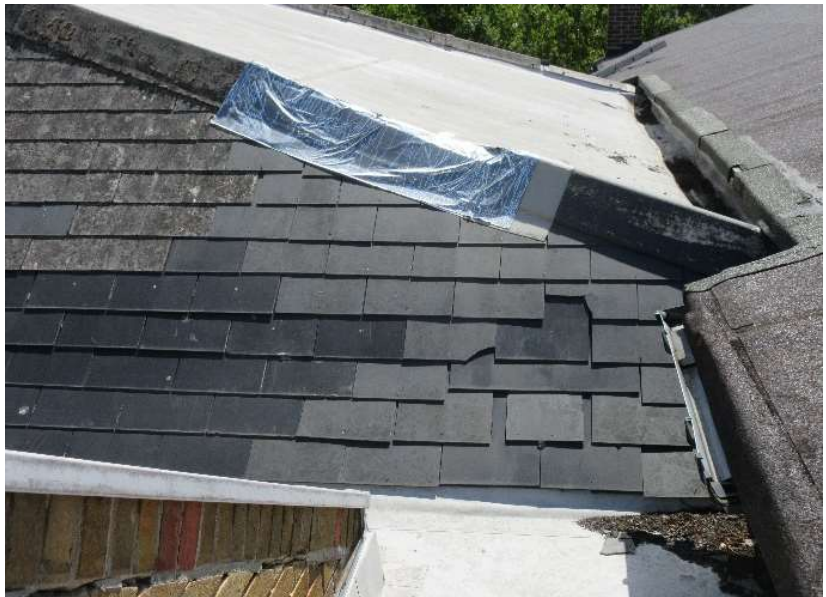
Internal gutter between Church and Hall Broken tiles at both hips, one patched with flashband
