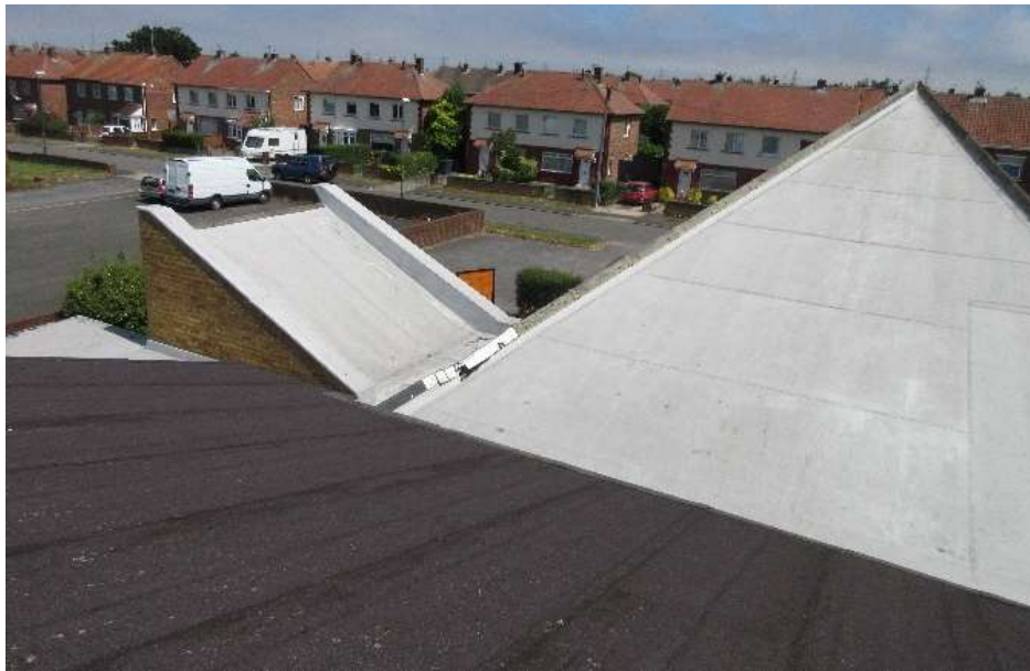
the hidden Sarnafil coverings on the Church hip and Porch from the Hall roof
