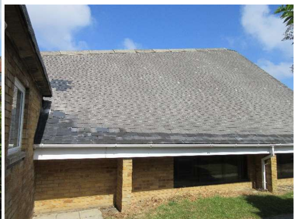
Narrow hidden gutter where the Church S slates butt to the flat roofed SE entry (para 16)
