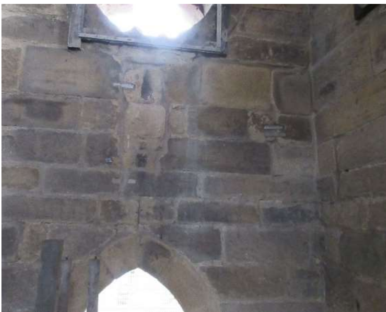
1992 stapled cracks between Belfry openings
