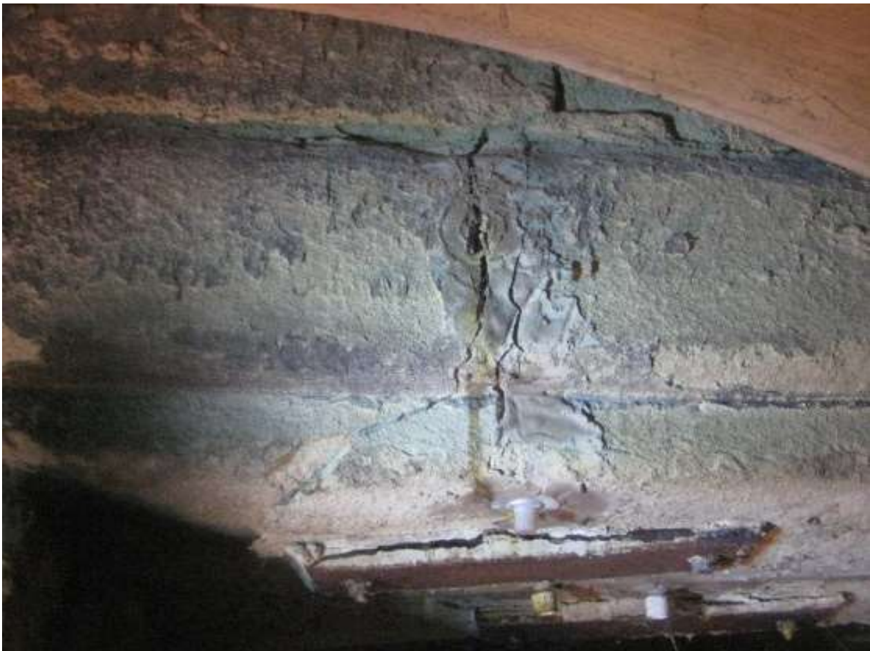
Rusting plates across cracked lintels at top of spiral 2012
