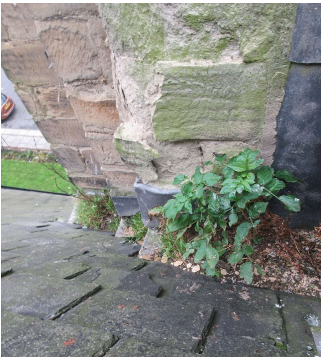
Blocked back gutters between Tower and Nave and deep decay at Tower SW buttress masonry
