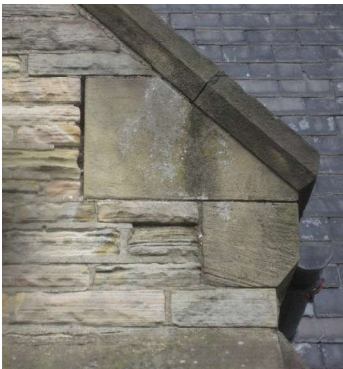
Open joints around the SW kneeler
