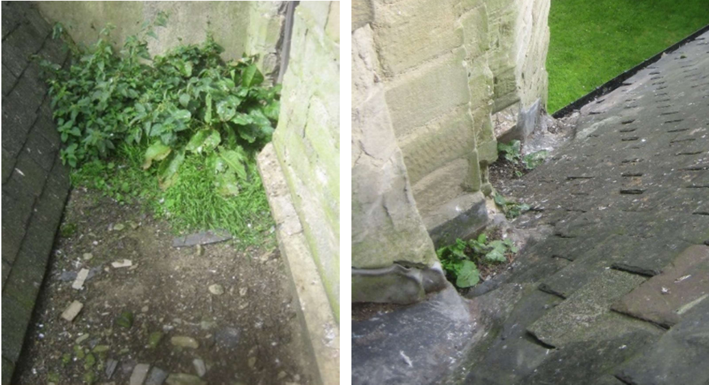
Abutment and Tower SE gutters before clearance October 2017
