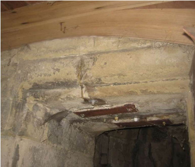
Rusting plates across cracked lintels at top of spiral 2012
