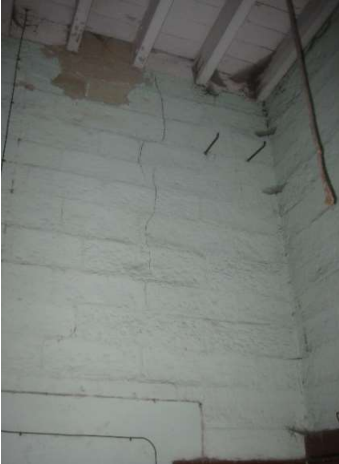
crack in ringing chamber 2012
