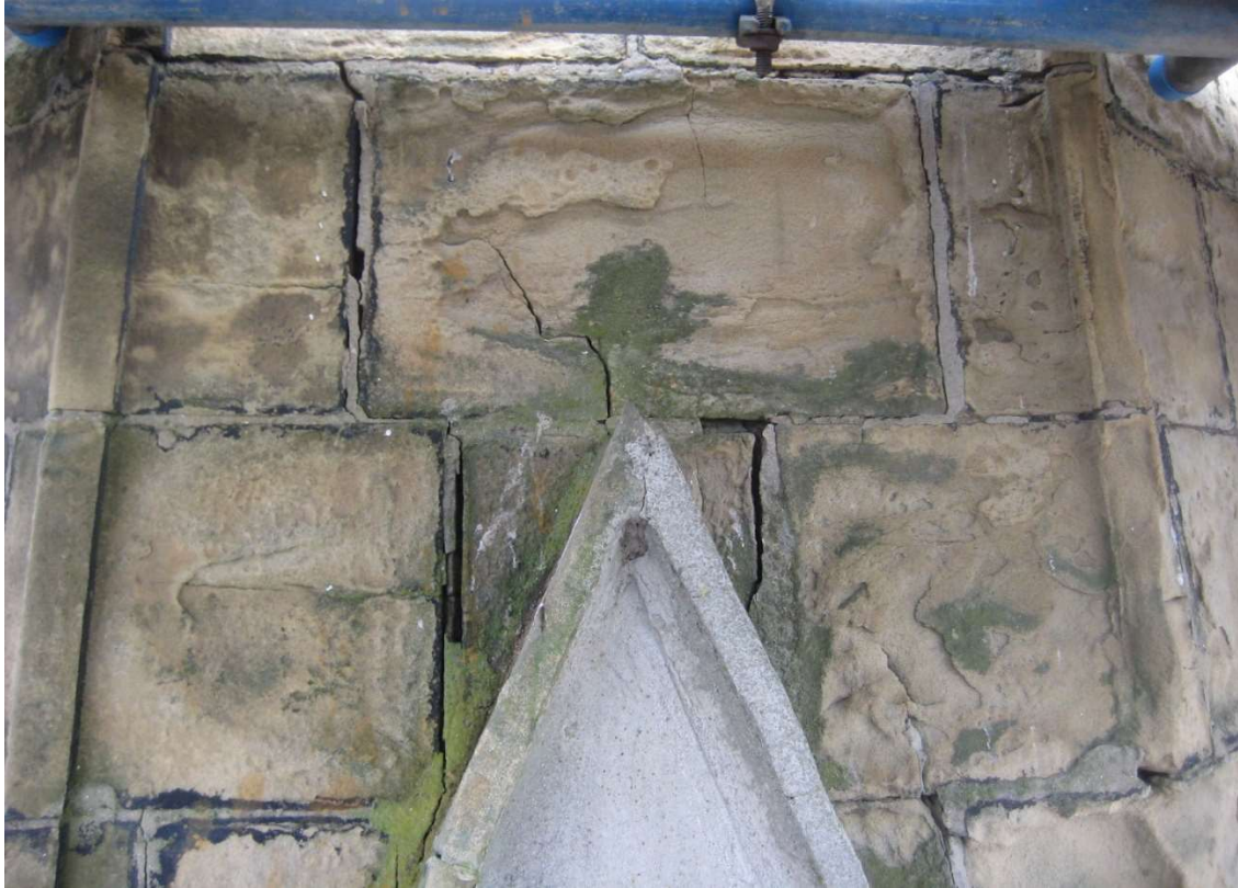
COMMON SPIRE DEFECTS 2011 photos – cracked stones and joints, past mortar patching at openings and further wind erosion
