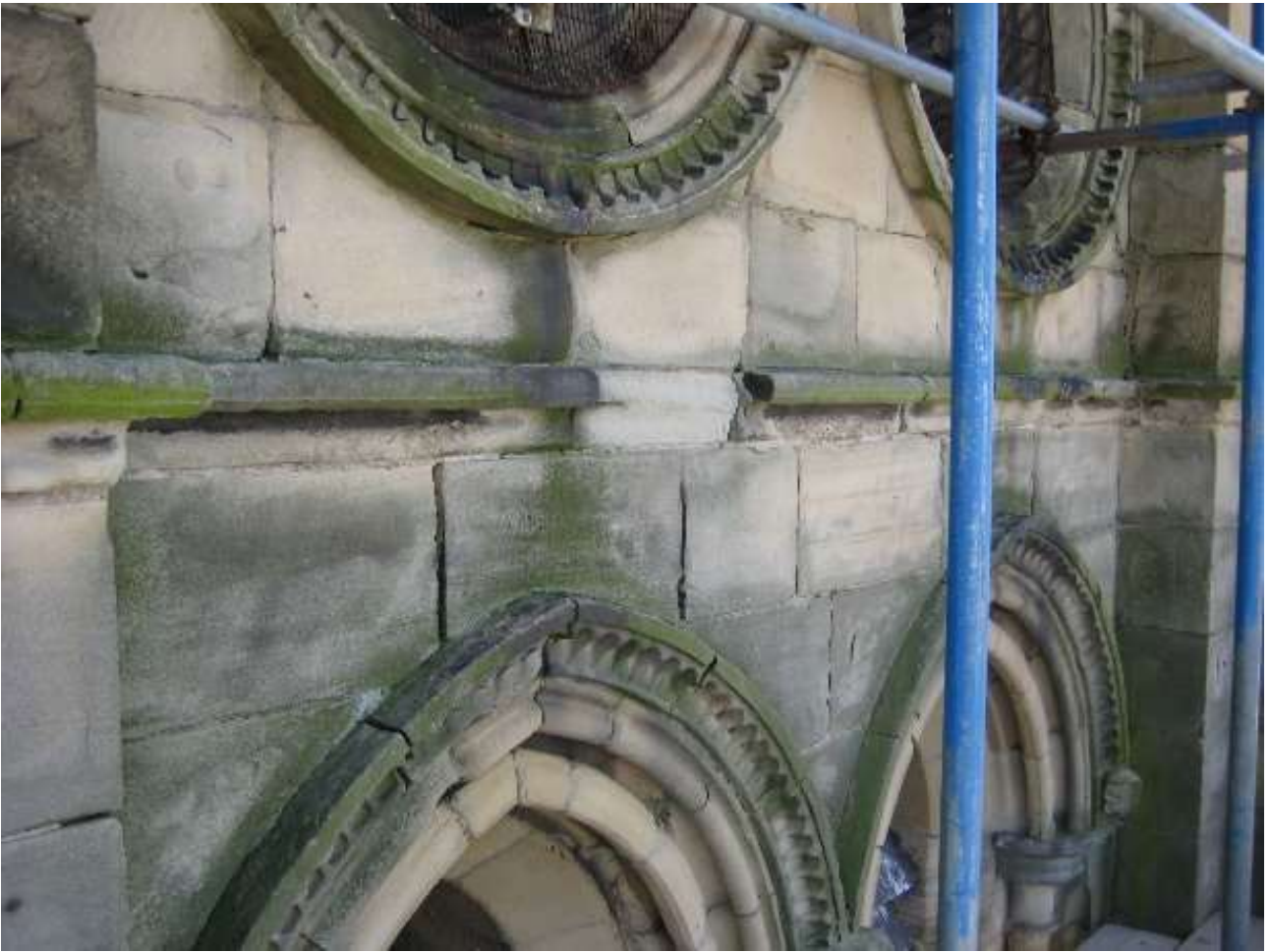
North Tower top lift 4
