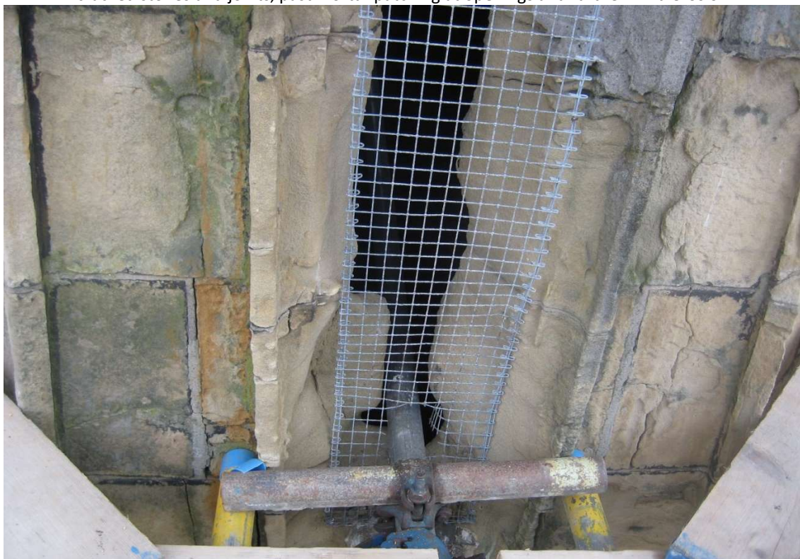
COMMON SPIRE DEFECTS 2011 photos – cracked stones and joints, past mortar patching at openings and further wind erosion
