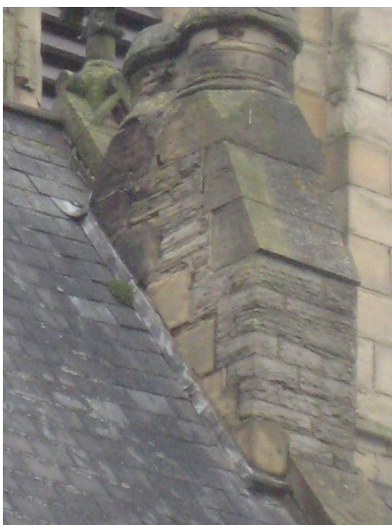
Plant in the slates and open joints at Chimney
