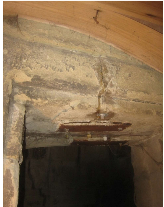
2017 – cracks wider than 2012?
