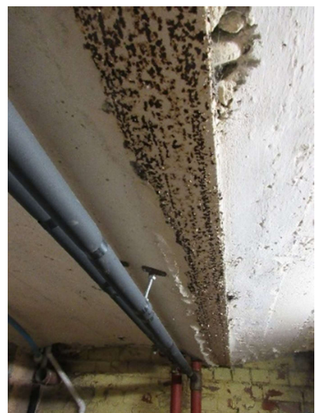
Insulation quilt not relaid over ceiling N of the wc steels at boiler ceiling
