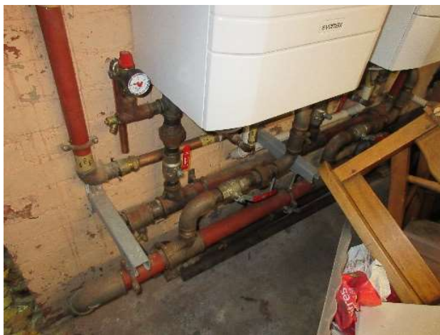
Scope for economy by more lagging at boilers
