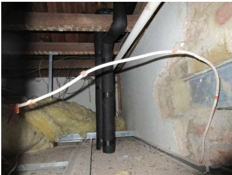
Insulation quilt not relaid over ceiling N of the wc steels at boiler ceiling
