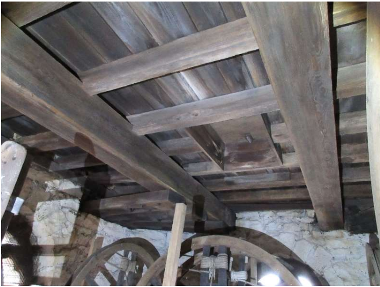
Tower roof structure
