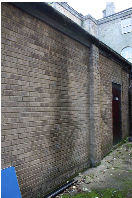
Damp patch to Hall wall due to leaking gutter
