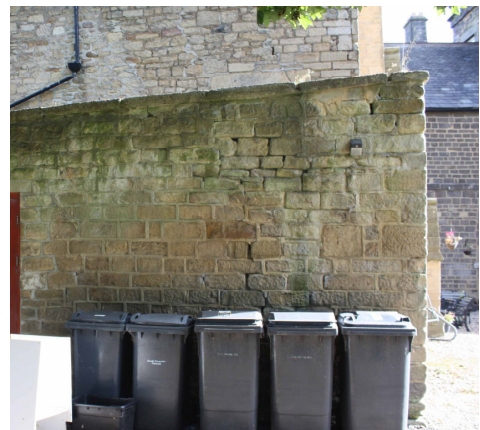
Prayer Room north wall with open joints
