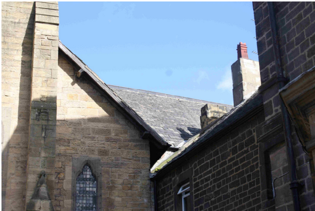
Nave gable with missing pointing to verge
