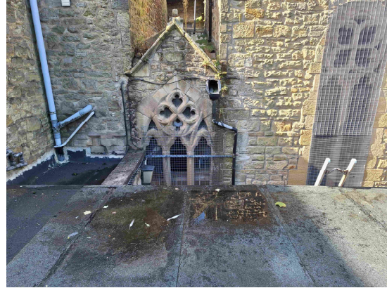
Hall flat roof ponding/ vegetation to gable beyond
