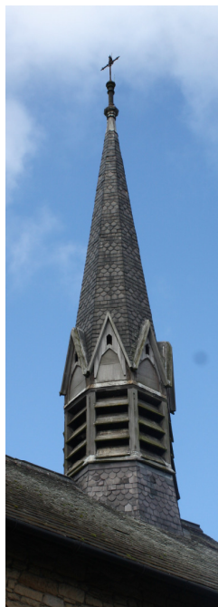
Fleche – missing mesh to louvred openings
