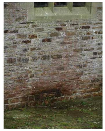
Splashback from leaking gutters causing damp walls
