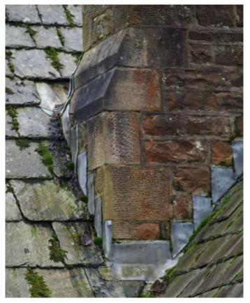
The back-gutter to the bellcote is almost certainly leaking - it should be renewed
