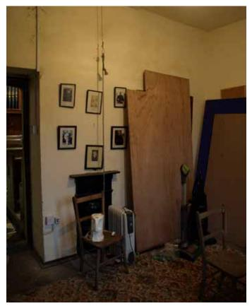
The Vestry is very damp. Remove stored materials, open the built-in cupboard, increase ventilation, remove pictures from damp wall. Fix source of water ingress
