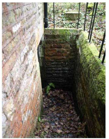
Boiler Room is very wet - a pump system should be arranged to drain the collecting water
