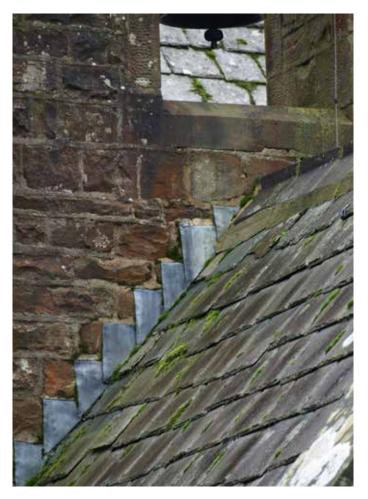
Masonry to the belicote requires fully re-pointing. Ideally the structure should be re-built on a lead tray
