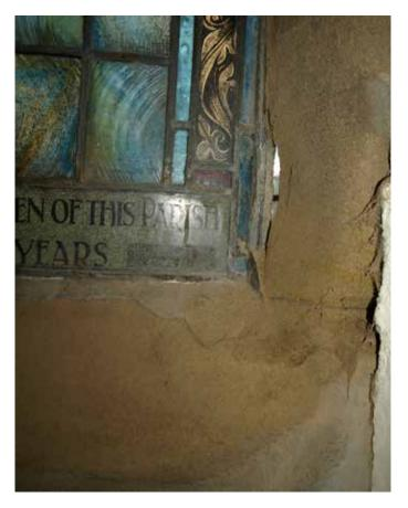
Window sIII - severe stone decay has opened up a gap against the glazing which will admit rain. Urgent repair required
