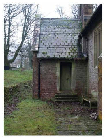
A build-up of vegetation around the building encourages damp conditions and prevents drying of the ground and walls at low level
