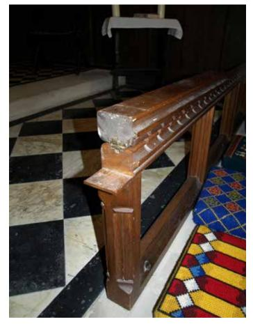
Altar rail hinges are badly worn, and the opening section lacks any proper support
