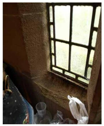
Vestry window (nll) in poor condition due to algae, stone decay, rusting metalwork
