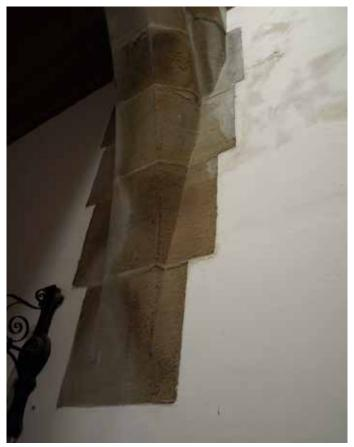
Leaking bellcote is now affecting the Chancel arch, causing rapid decay of the dressed stone
