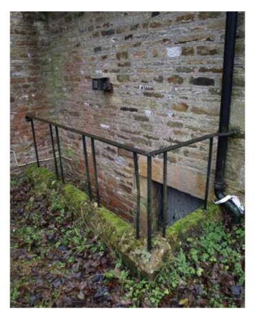
Railings to Boiler Room steps need to be repaired
