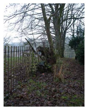
Damage caused by trees to boundary fencing should be made good
