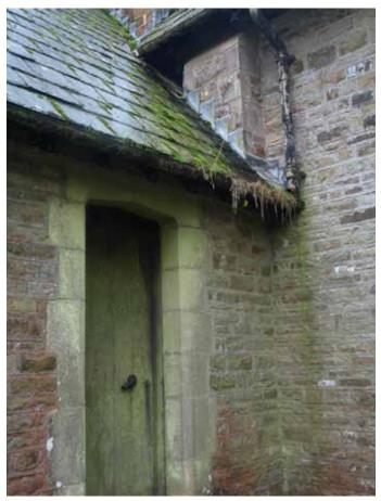
Gutters are full of debris and vegetation in places. Clean out every 6 months to avoid overflow and resultant water ingress
