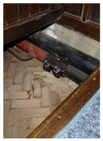
Recent heating pipe repairs have stopped the leaks which were affecting areas of the woodblock flooring
