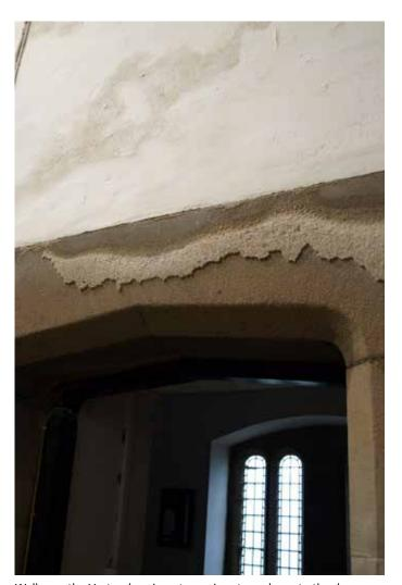
Wall over the Vestry door is wet, causing stone decay to the door surround. Due to leaking bellcote above
