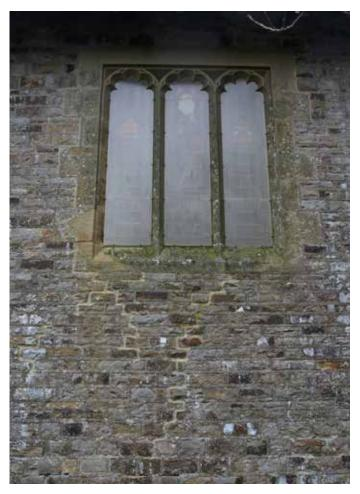
Earlier cracking below south windows, pointed up and in places opening up again
