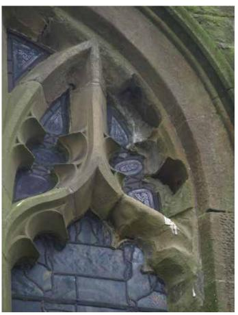
West window - deterioration of masonry and poor quality repairs
