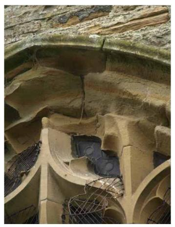
East window - deterioration of masonry surround, failure of grilles
