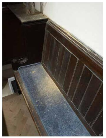
Deposits of stone dust are indicative of the rate of decay. This should be removed by vacuum cleaning
