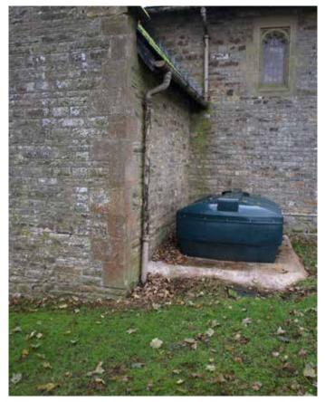
The plinth to the recent oil tank has been built above ground level against the Transept wall, causing damp to the base of the wall internally
