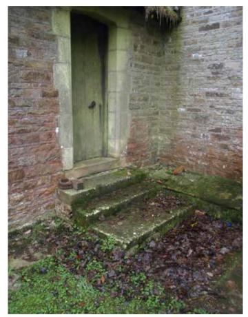
Accumulation of debris, moss, and vegetation to surfaces prevents drying out and leads to further colonisation. Debris on steps and paths is a safety hazard
