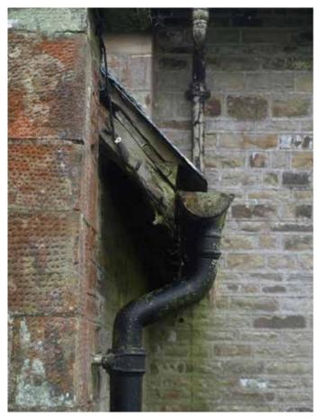
Rafter ends in poor condition, and covering bargeboard missing
