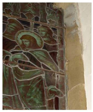
East window - no longer weather-tight due to erosion of the sandstone surround. Note also rusting saddle bars
