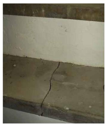
Cracking in the internal cill of window sIV - should be monitored for change over time
