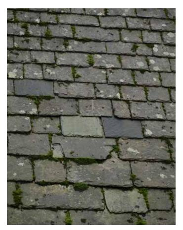
Poorly matched replacement slates. Adjacent slates appear to have been damaged during the work
