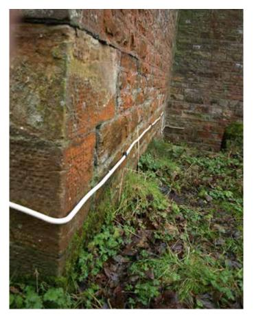
New feed pipe to boiler from recent oil tank installation
