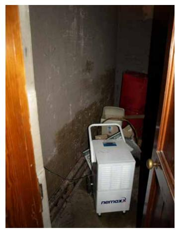
South Transept is extremely damp. Fix sources of ingress, remove plaster from walls, provide drain for dehumidifier so it can work, increase ventilation
