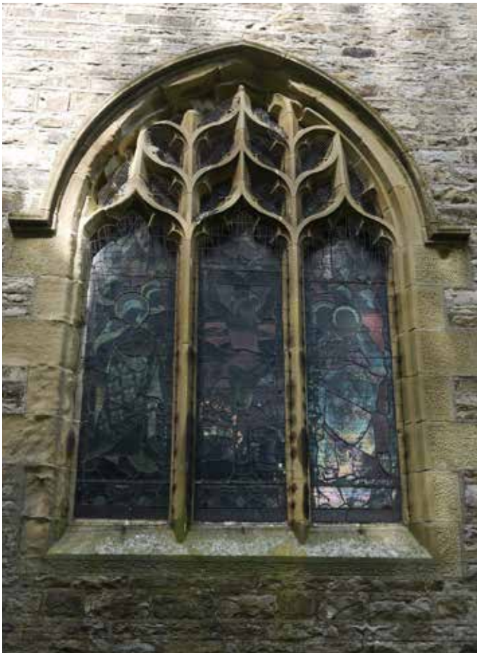
Main east window deterioration
