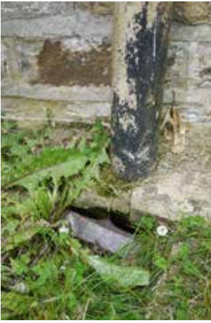
Stone/concrete caps over gullies can cause more of an issue with vegetation becoming trapped, and they less easy to clear out
