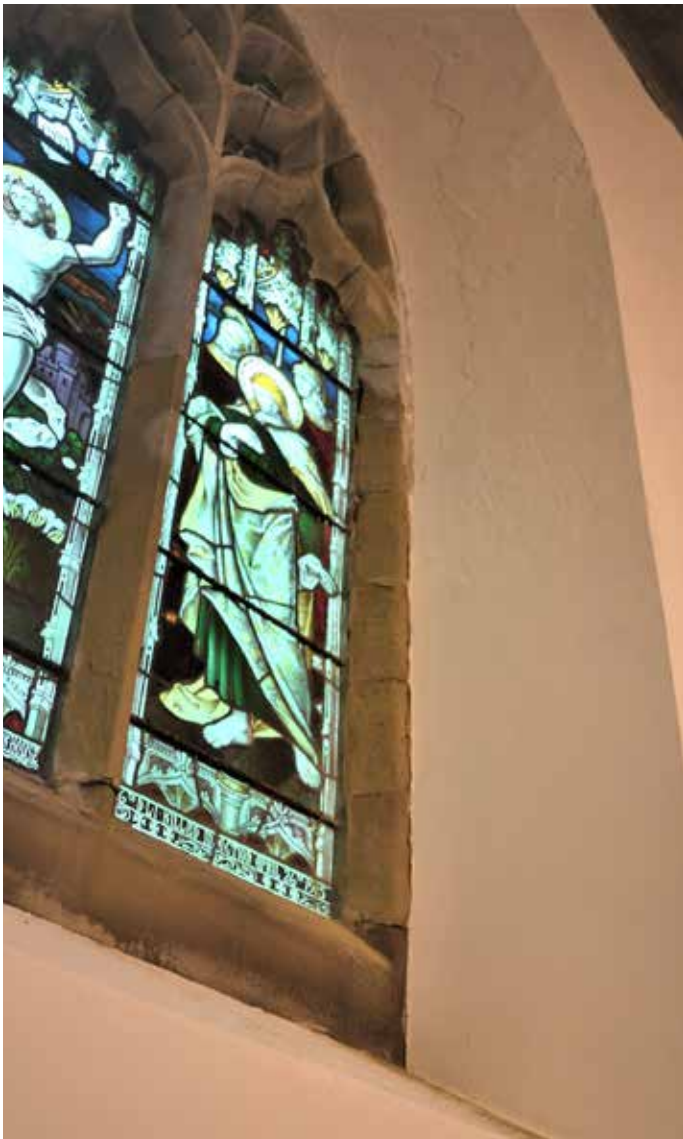
East window stonework deteriorating due to salt damage internally
