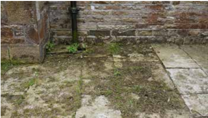
Stone/concrete caps over gullies can cause more of an issue with vegetation becoming trapped, and they less easy to clear out
