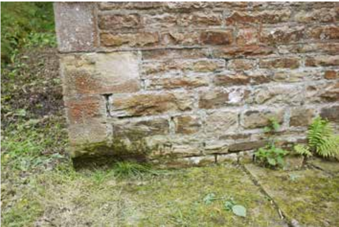
Damp and deterioration at base of wall
