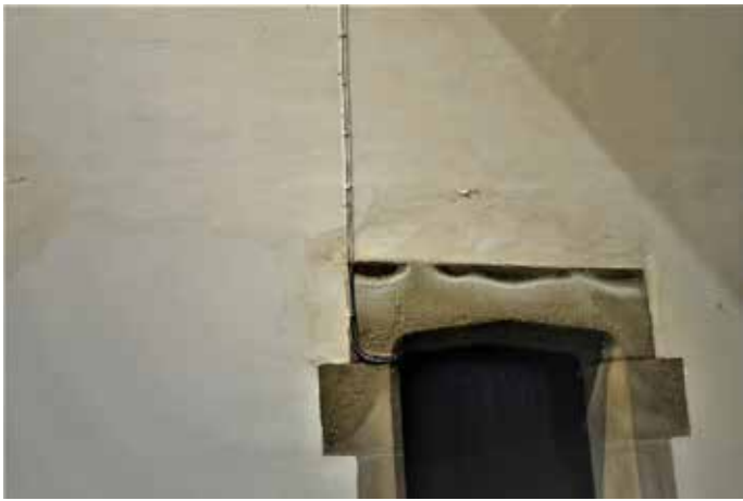
Deterioration of stone reveal to vestry and of plasterwork above, caused by issues with bellcote and chimney over
