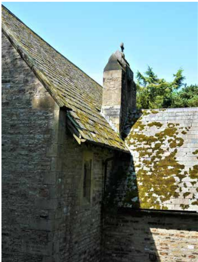
Timberwork and gutters require repair and redecoration, leaks from bellcote to be investigated
