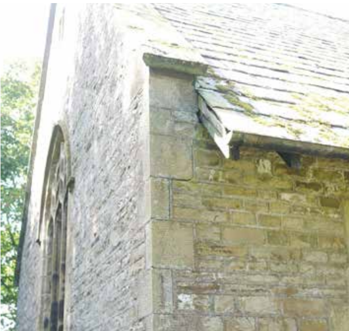
Hairline crack around quoins below watertabling at north-east corner of chancel
