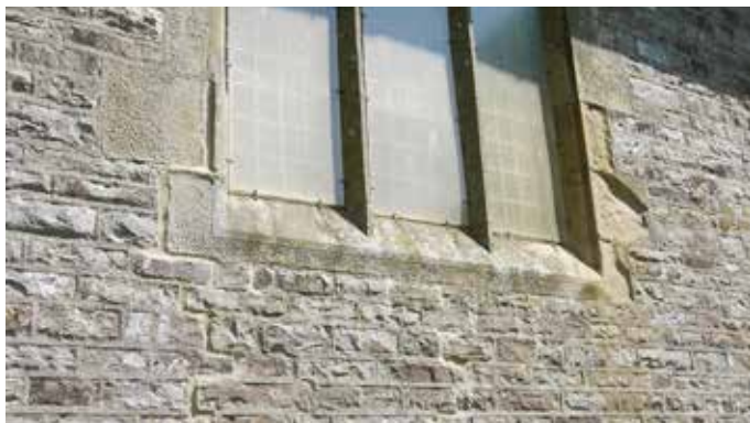
Cracking below windows (south nave) and deterioration of dressed sandstone reveals jamb stones
