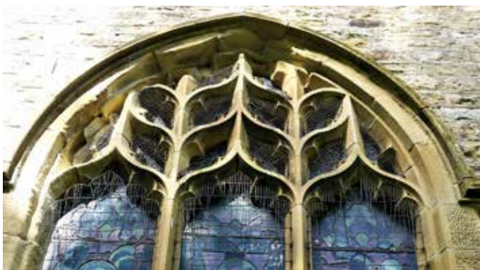
Deterioration of tracery at the top of main east window. Ferrous fixings of deteriorated wire guards causing localised rusting
