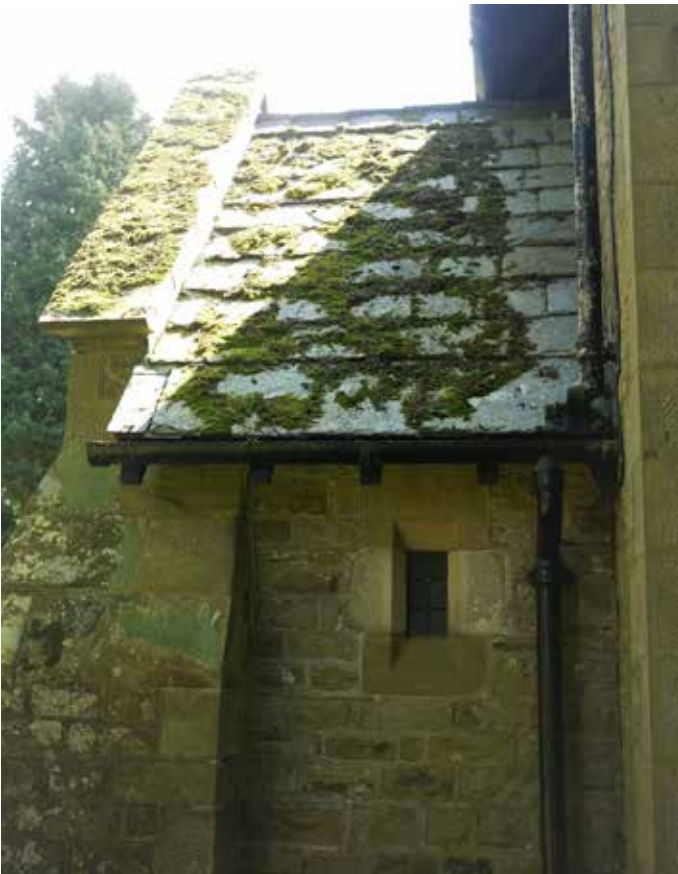
Moss build up, encouraged by lack of light and proximity of trees
