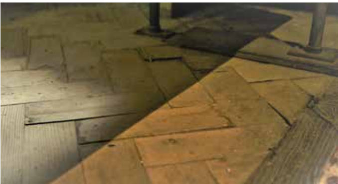
Movement in woodblock at east end of north aisle, indicating possible ground movement
