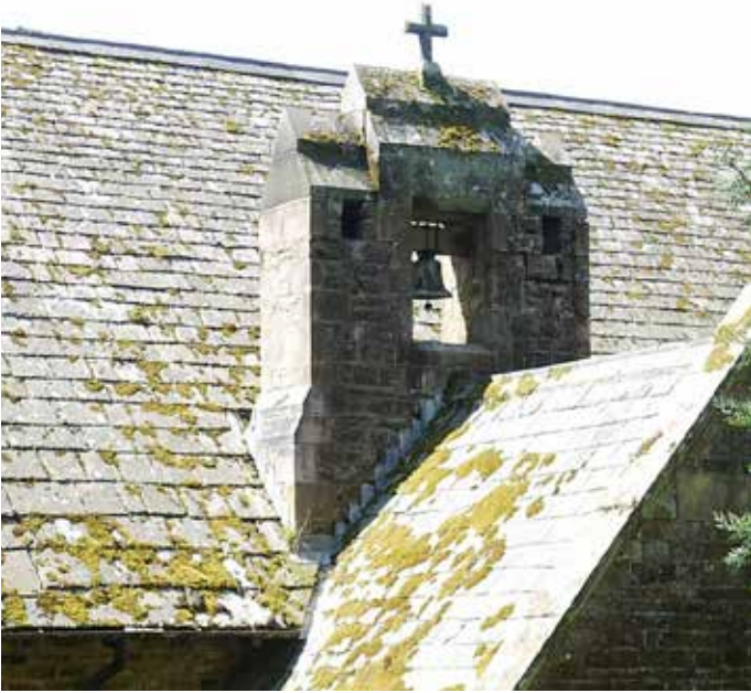
Bellcote requires some repair to stop water ingress below
