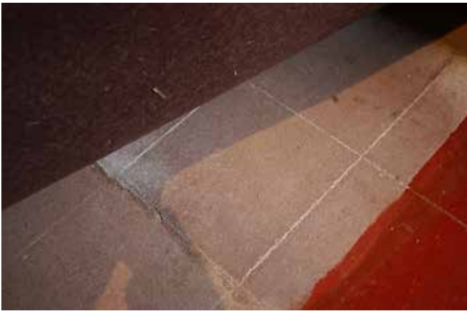
Beneath carpet - junction of original sandstone flags (top) with concrete floor, lined (below) and red paint to perimeter where exposed
