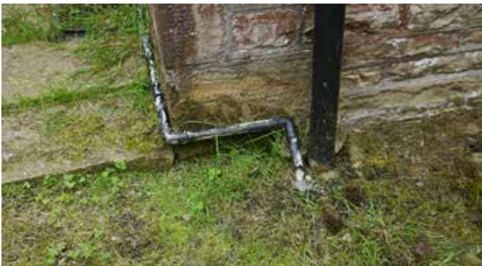
Outlet from vestry sink flows into blocked gully
