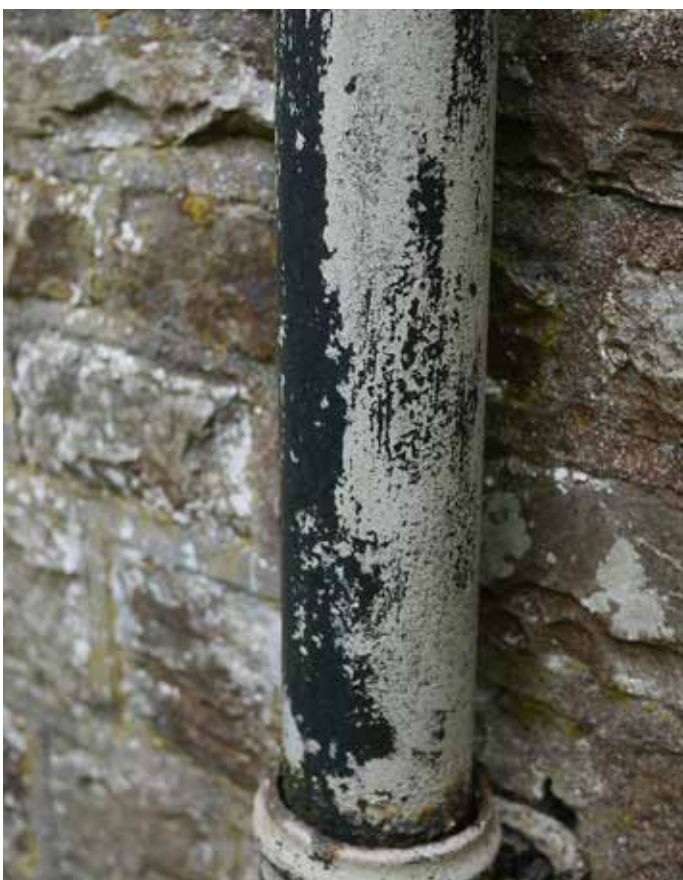
Rainwater goods would benefit from redecoration, as well as regular clearing out
