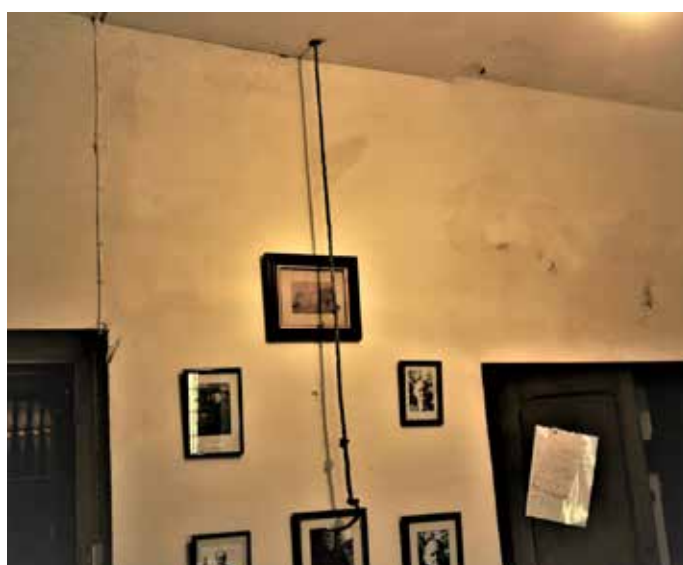
Damp in south wall of vestry, below chimney and bellcote
