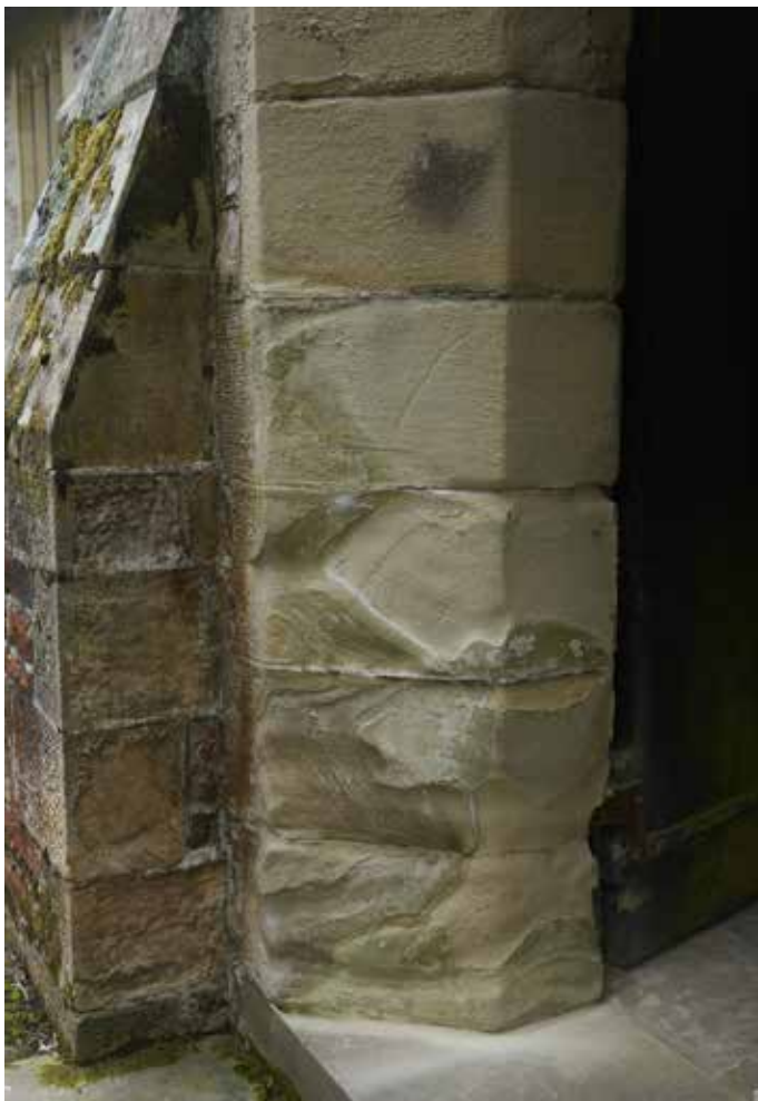
Severe deterioration to eastern jamb of porch archway
