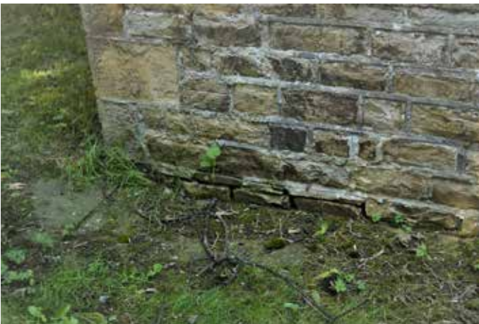
Stone flags laid up against the wall trap moisture in the ground and encourage damp to rise in the masonry walls. This is beginning to damage stonework and pointing at low level.
