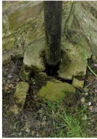
Stone/concrete caps over gullies can cause more of an issue with vegetation becoming trapped, and they less easy to clear out
