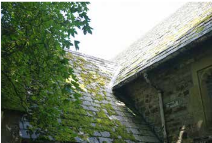
Moss build up, encouraged by lack of light and proximity of trees
