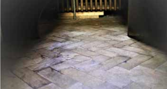
Staining to woodblock - could either be leaking pipework, or damp from below
