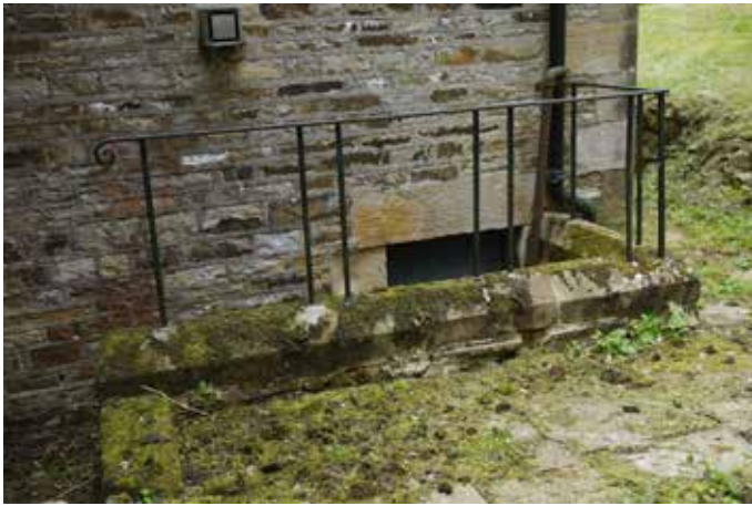
Flagged areas and cellar steps would benefit from a tidy up
