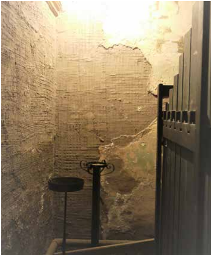
Organ loft / south transept - new render is too hard and not assisting the drying out of the walls - should be removed to expose stonework and walls allowed to dry out
