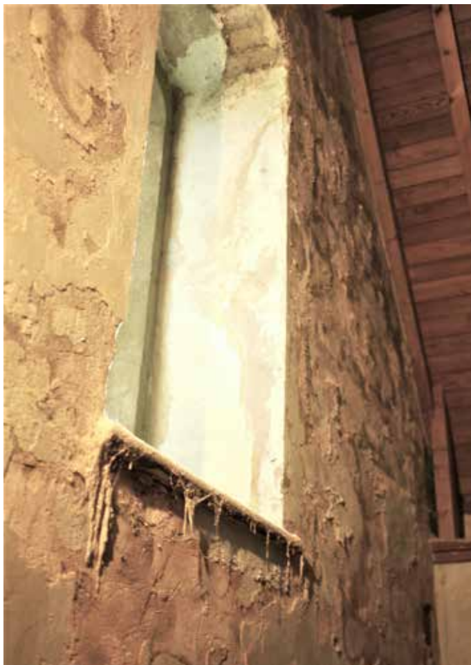
South gable of organ loft in poor condition due to salt damage
