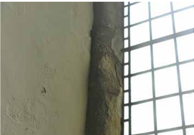
Deterioration of sandstone window reveals and plasterwork
