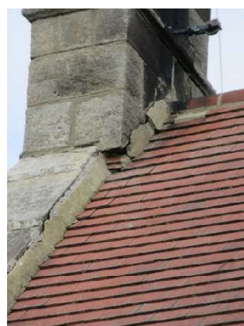
W Gable S side
