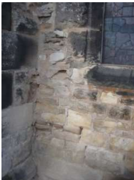
Next to Nave mid SE buttress
