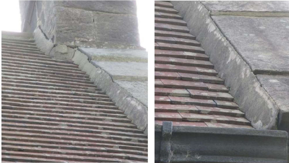
W Gable N side
