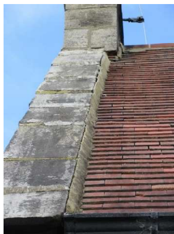
W Gable S side
