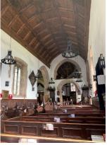
3.2.1.3. The plaster work at high level on both the south and north sides of the Nave is in good condition following lime plaster repairs in 2004. The Church was decorated internally in 2004 and in general is in good condition.
