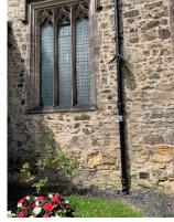
2.2.16.3. There is substantial decay at low level and also inappropriate cement mortar.
