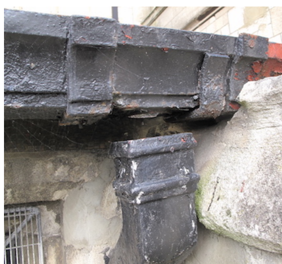
06 South Aisle roof - missing spigot at east end of gutter
