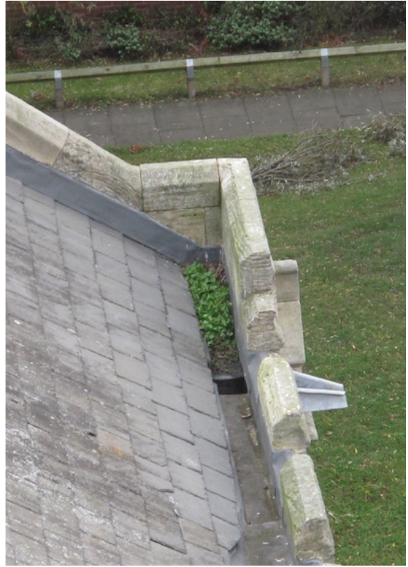
02 Nave roof east end - blocked gutter
