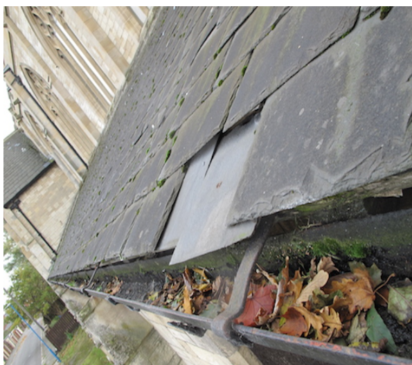
05 South Aisle roof – full gutter and missing slate
