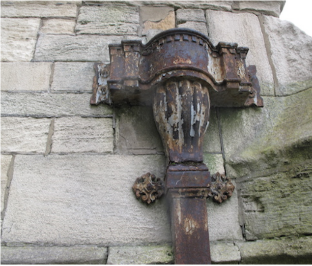
13 North Porch – rusty east gutter rainwater hopper and downpipe
