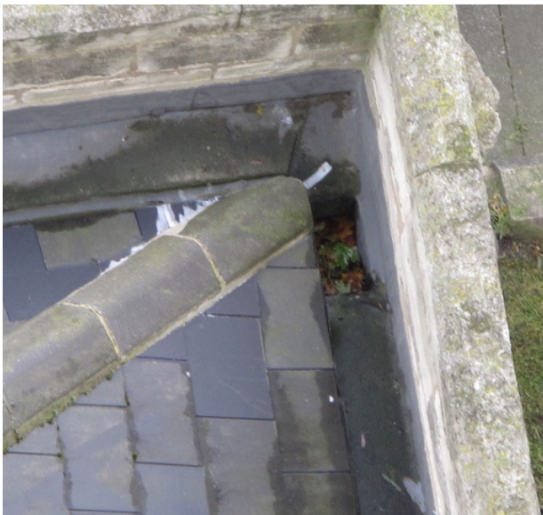
03 North Porch roof - blocked sump outlet at north east corner
