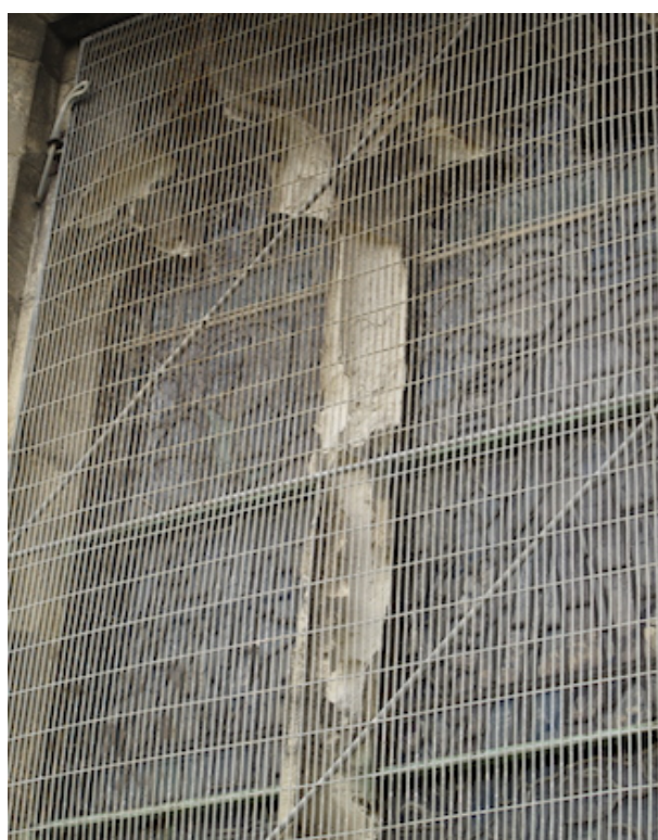
08 Clergy Vestry window – stonework erosion
