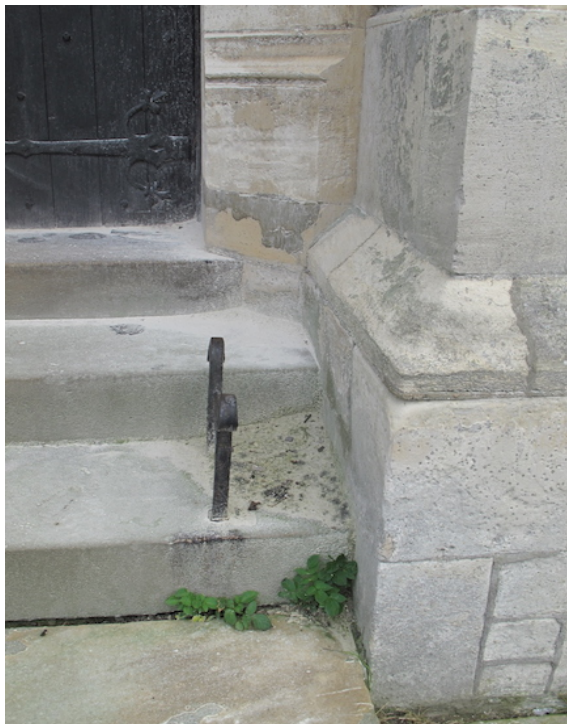
11 North Porch west face doorway – stone dust on steps
