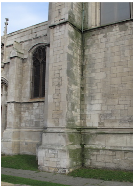
07 West side of Tower – missing lightning conductor tape
