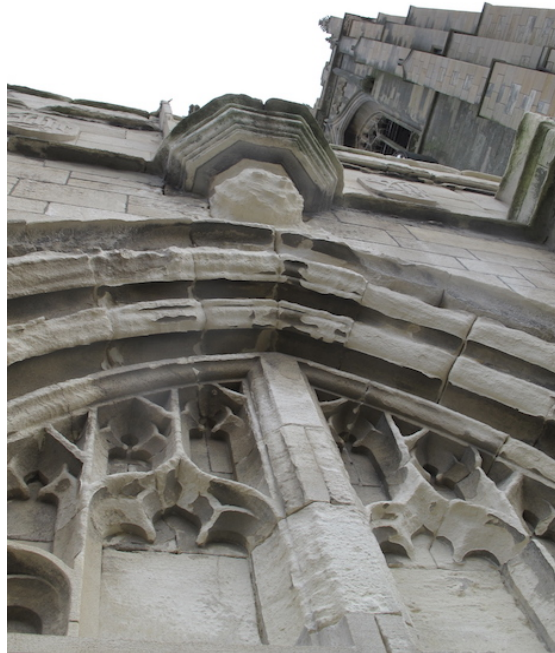
12 North Porch west face – eroding stone features
