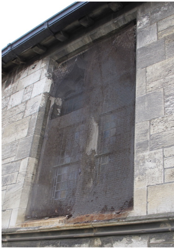
09 North Aisle – rusty and badly fitting window guard
