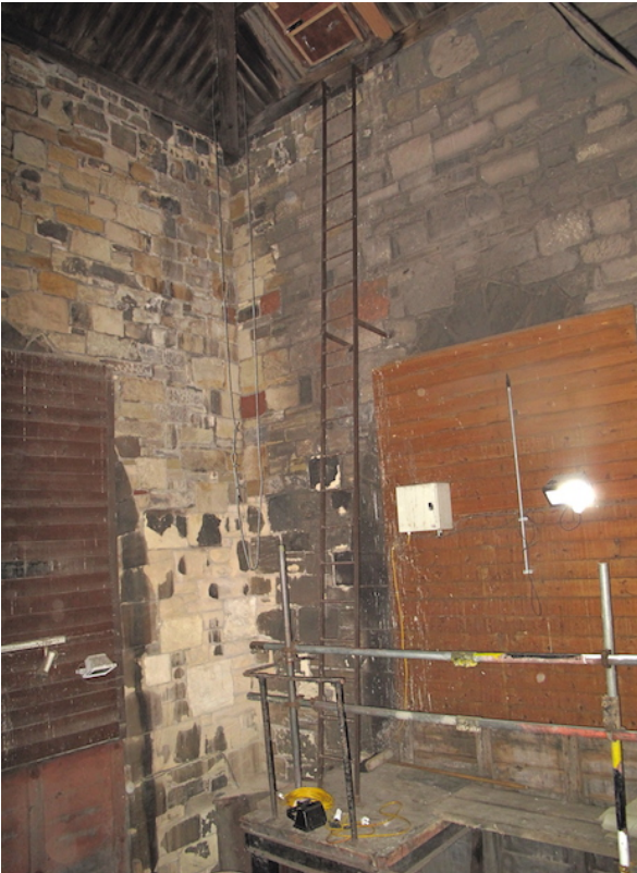
15 Belfry – unguarded ladder up to roof access hatch
