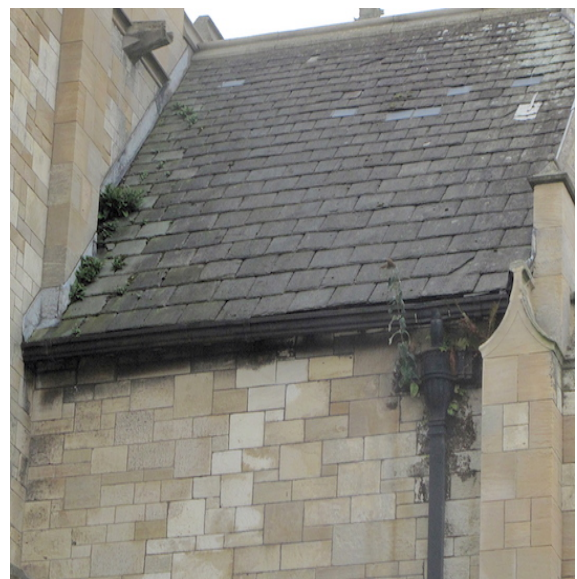
04 Organ chamber roof - east slope - blocked outlet
