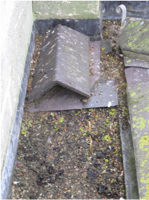
01 Tower Roof gutter south side
