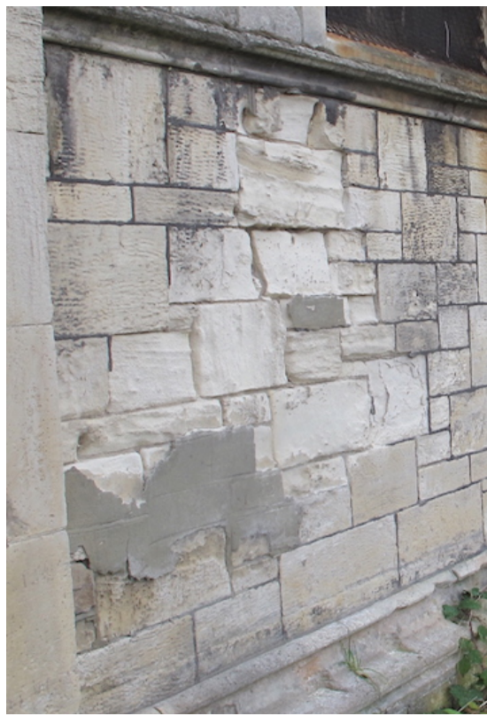
10 North Aisle – badly eroded stone at east end
