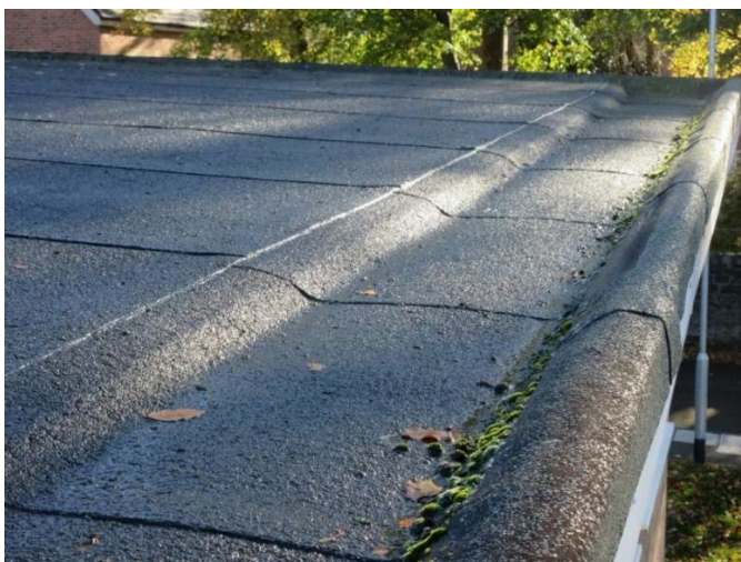
Nave integral gutters
