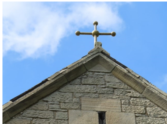
Loss of pointing to Eastern verge
