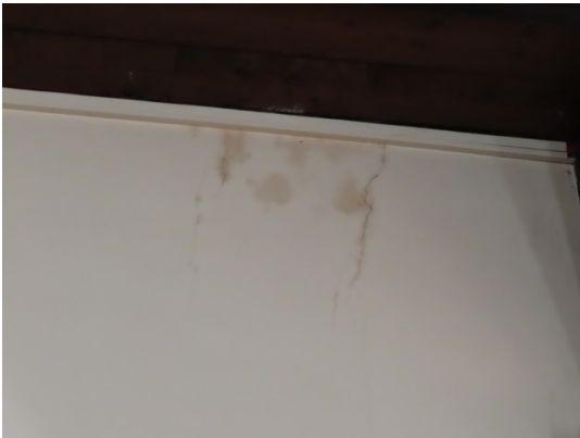
Cracking to stonework to Western window Damp staining over the vestry window
