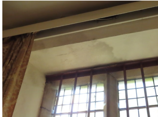
Cracking to stonework to Western window Damp staining over the vestry window
