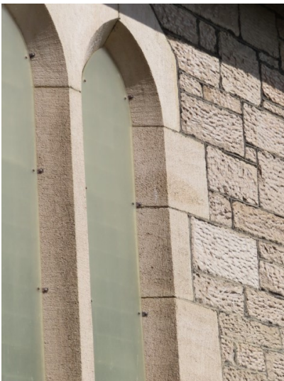
Yellowing protection to window (left) and cobwebs and debris to void between window and outer protection (right and below right)
