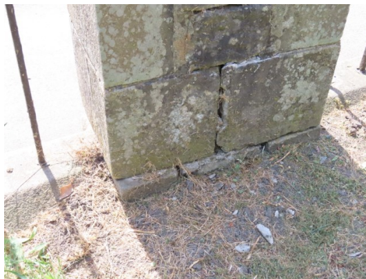
Damaged pier to Eastern side of Southern boundary
