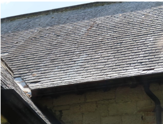
Slipped and missing slates to various roof slopes (above and below)
