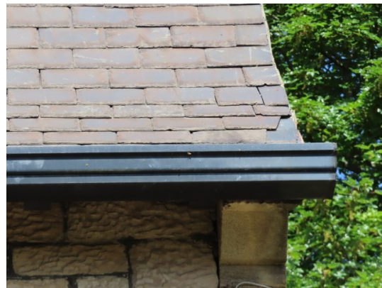
Slipped and missing slates to various roof slopes (above and below)
