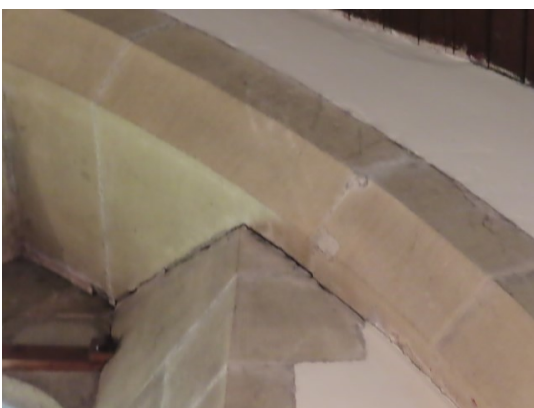
Cracking within window reveal
