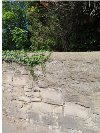
Grass and ivy growth to external face of the Southern boundary
