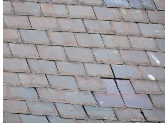
Slipped and missing slates to various roof slopes (above and below)
