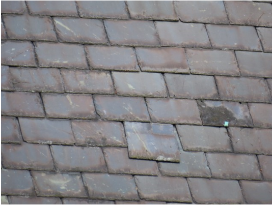
Slipped and missing slates to various roof slopes (above and below)
