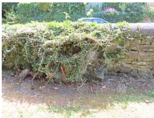
Vegetation growth to internal side of the Southern boundary (above and below)
