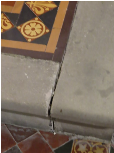
Open joints to altar dais (left) and Chancel step (right)
