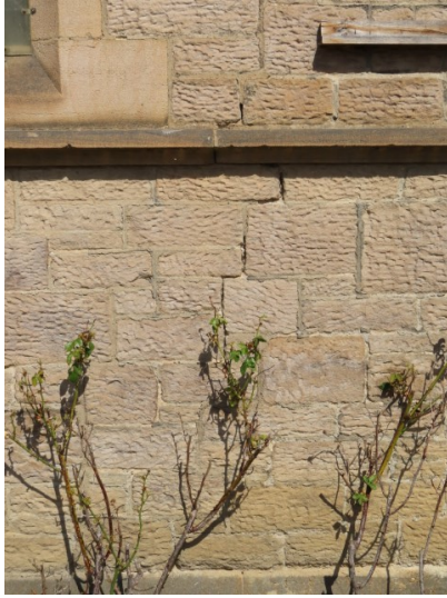
Cracking /open joints to the South Elevation and soil level close to vents
