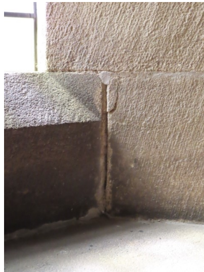
Damp staining on North wall by Vestry
