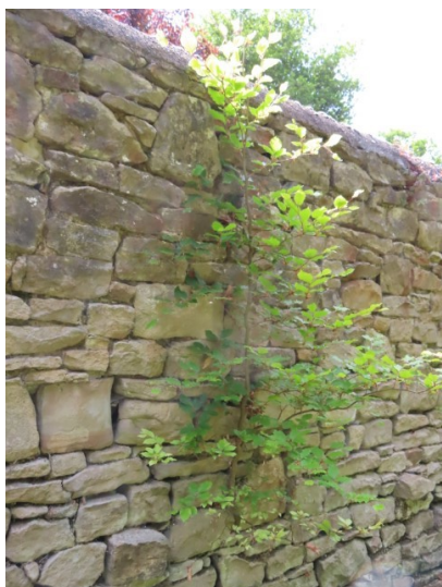
Vegetation growth to internal side of the Southern boundary (above and below)
