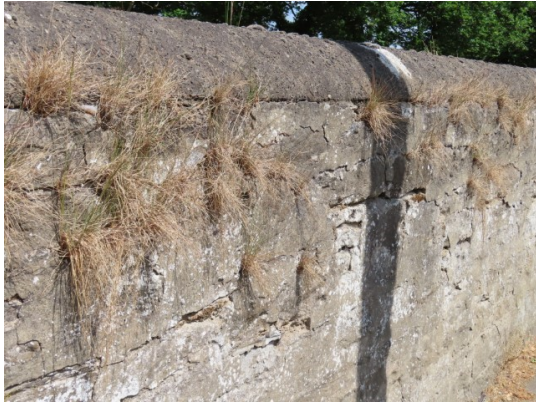
Grass and ivy growth to external face of the Southern boundary
