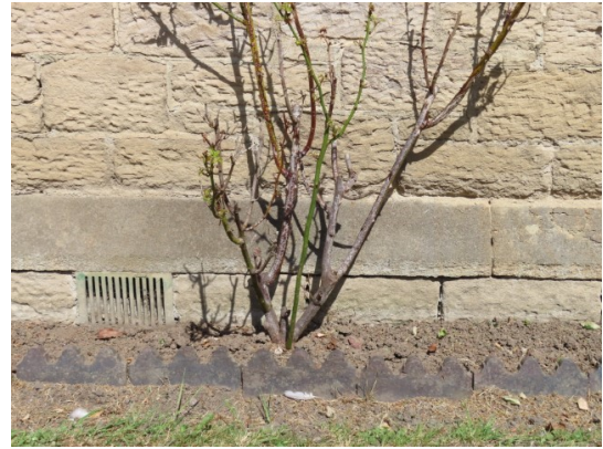
Cracking /open joints to the South Elevation and soil level close to vents
