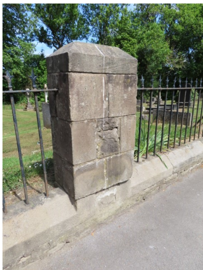
Damaged pier to Eastern side of Southern boundary
