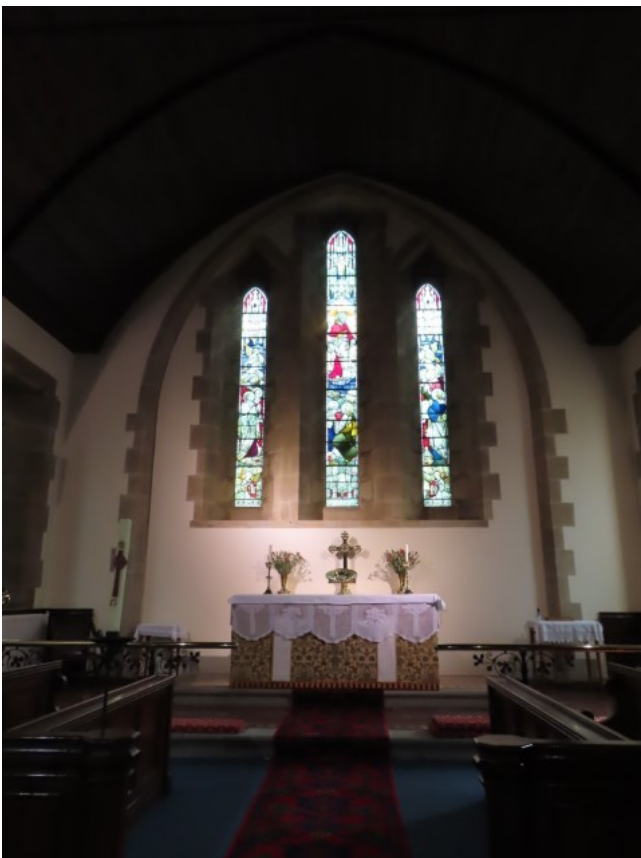
General view of Chancel looking East
