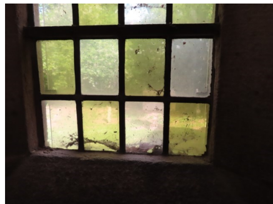
Yellowing protection to window (left) and cobwebs and debris to void between window and outer protection (right and below right)
