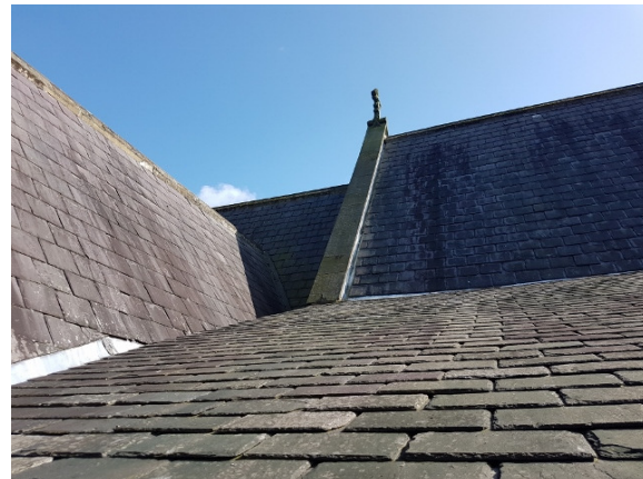
Junction of Organ Chamber, Nave & N. Aisle roofs
