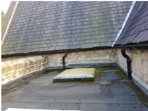
Flat roof over Vestry
