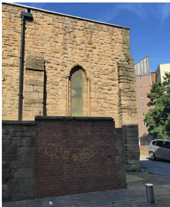
8. Lead drip to S gutter and SE corner without it, leading to water saturation and organic growth
