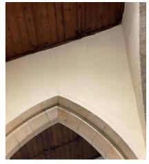
Figure 20- Crack to southern aisle arch
