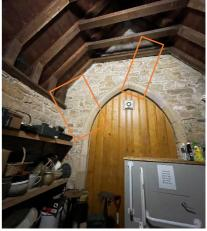
Figure 21- Crack to south porch
