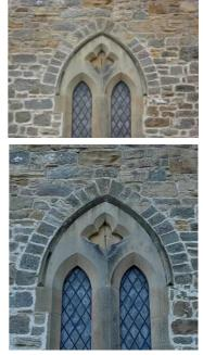
Figure 6 - crack in lancet in 2014 (top) and 2023 (bottom) item 8.3.2
