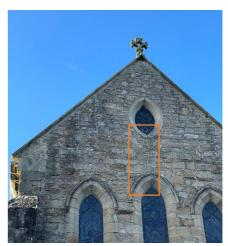
Figure 11 – East lancet cracking
