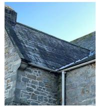
Figure 3- Gutter to west organ loft
