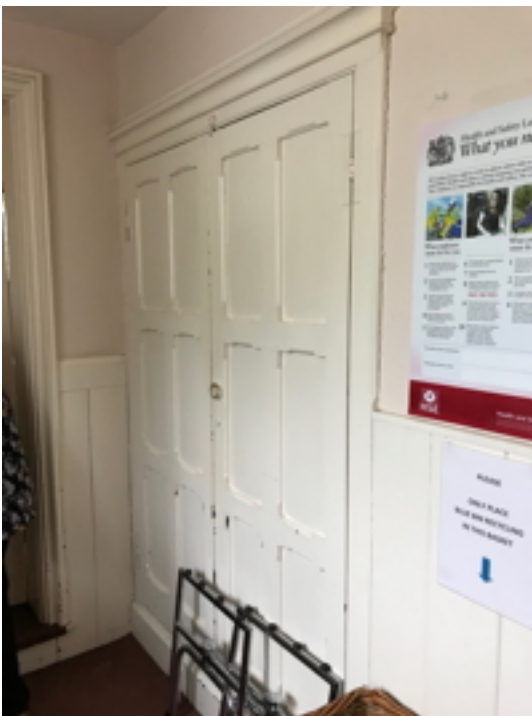
Vestry Corridor South Wall
