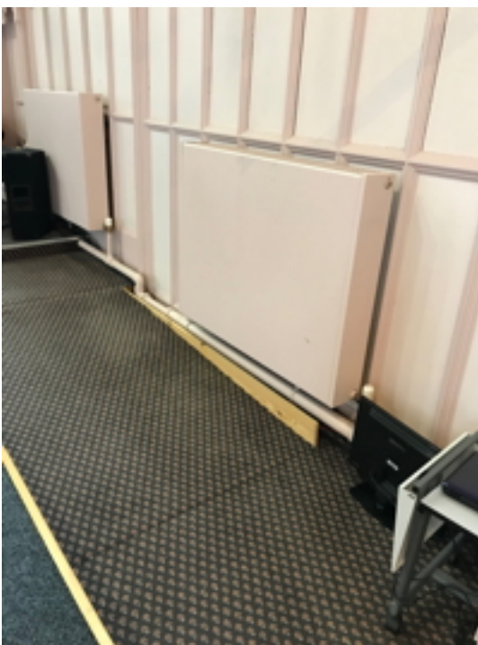
Typical Nave Radiator
