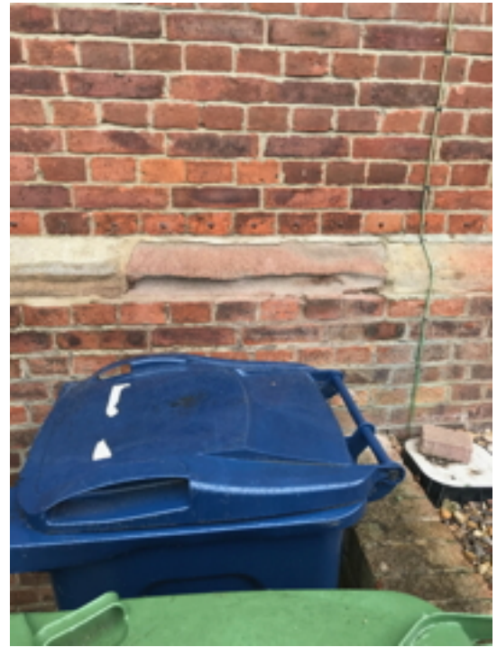
Erosion to Plinth
