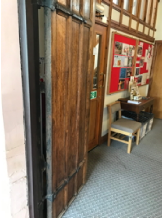
South Porch Doors
