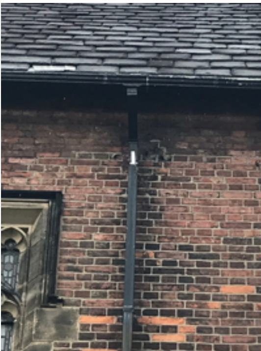
South Elevation East End Rainwater Pipe
