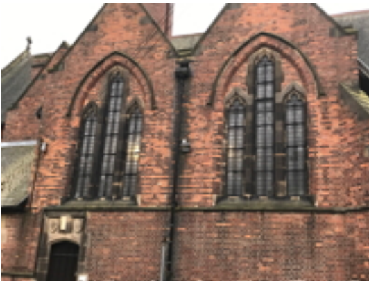
North Aisle Windows
