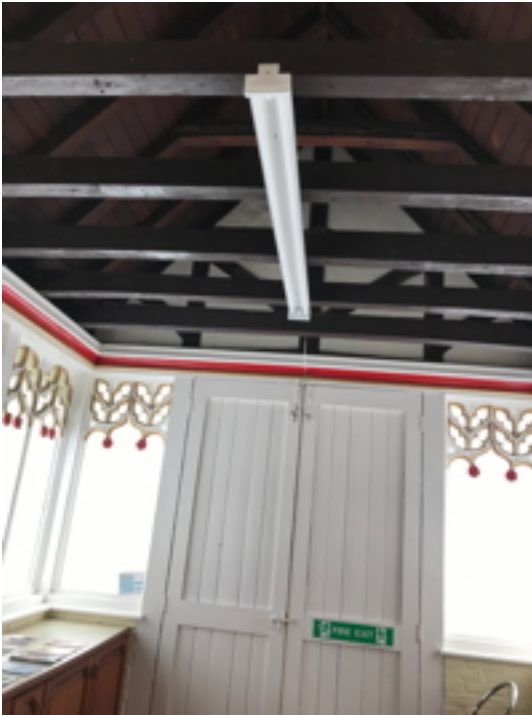
South Porch South Wall
