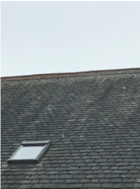
North Elevation Roof
