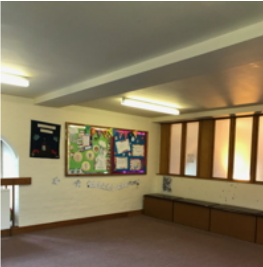
First Floor Meeting Room Looking North East
