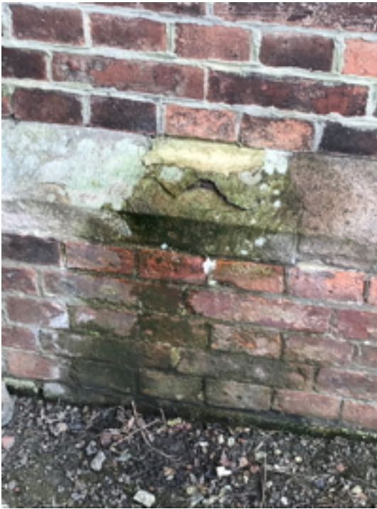
Staining to Plinth
