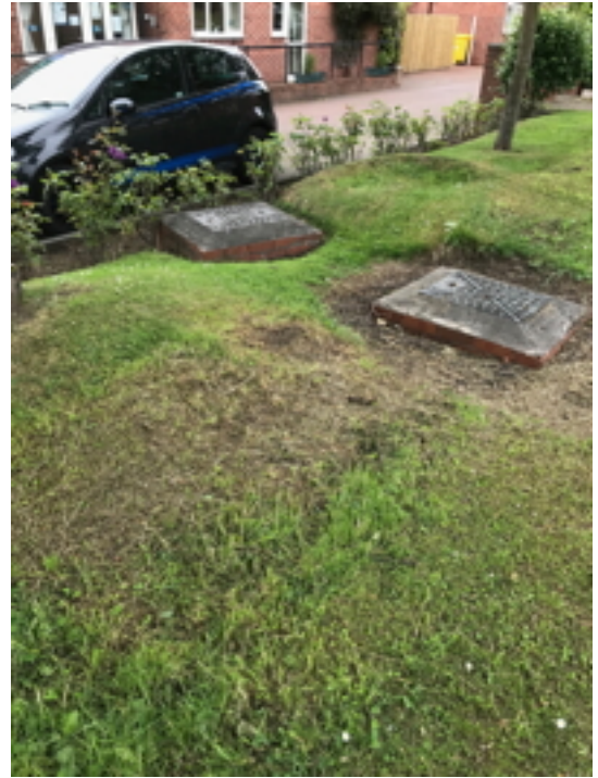
Inspection Chambers West End
