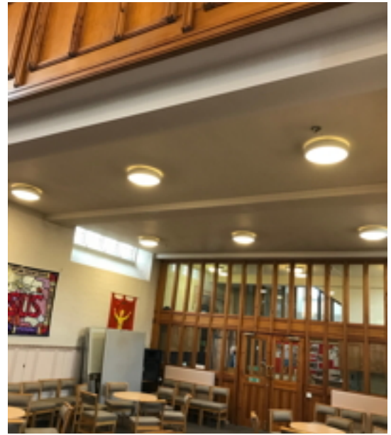
Lower West End Ceiling
