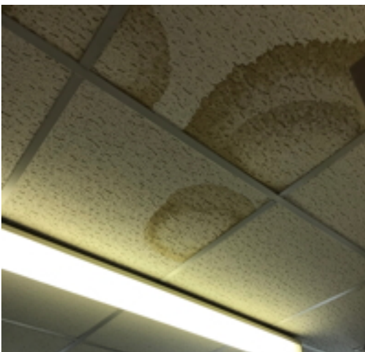
Staining to Vestry Ceiling
