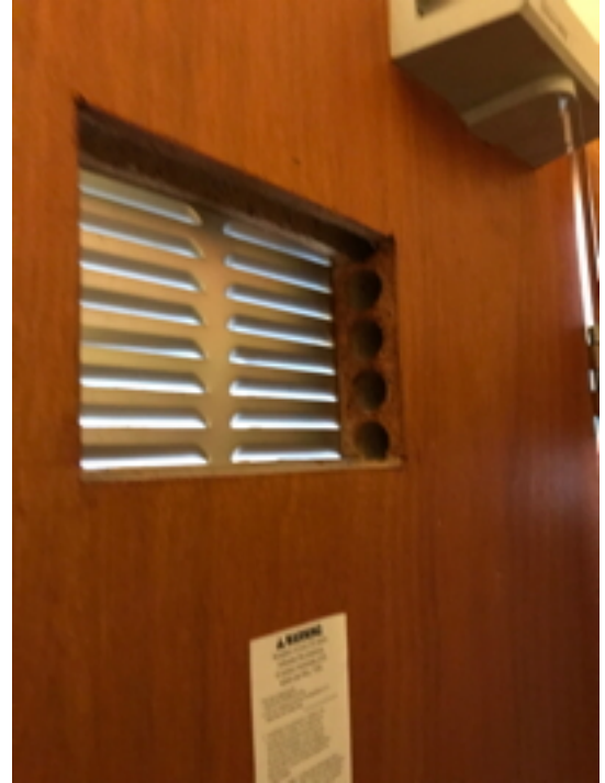
Unsatisfactory Grill to Boiler Room Door
