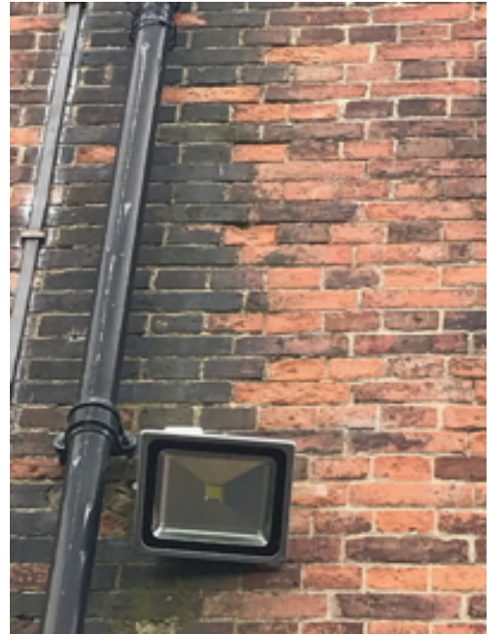
Erosion of brick faces to North Aisle north wall
