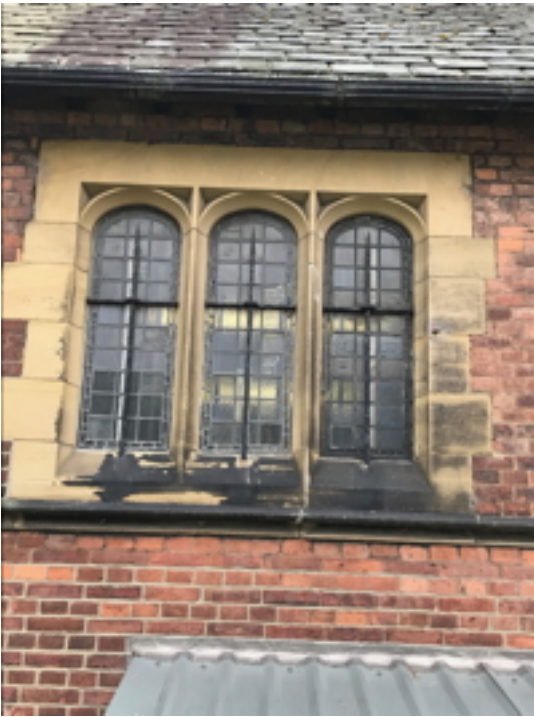
Vestry North Elevation Window
