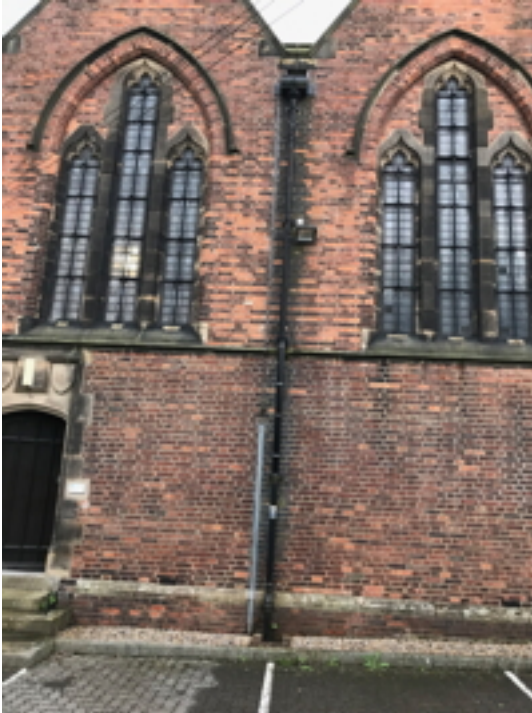
North Aisle Rainwater Pipe
