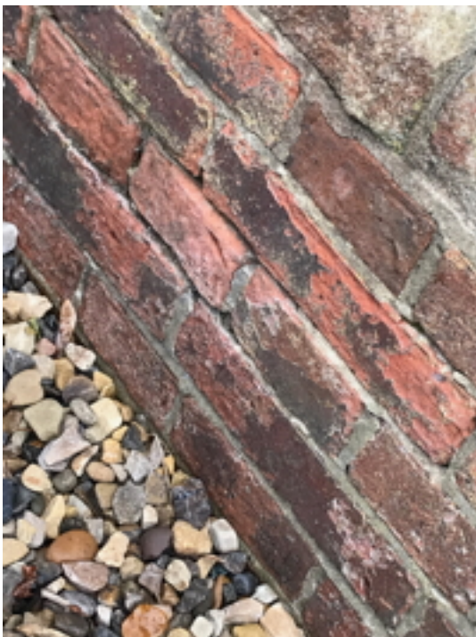
Areas requiring repointing to plinth
