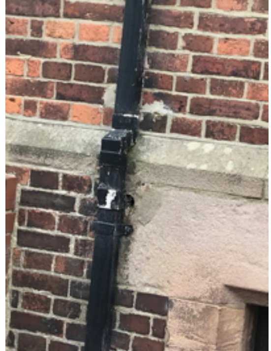
Vestry Rainwater Pipe
