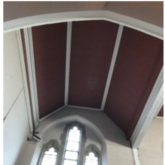
North Aisle Ceiling
