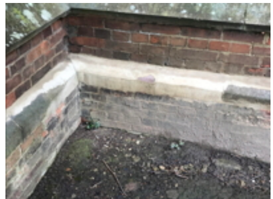
Unsightly plinth repairs
