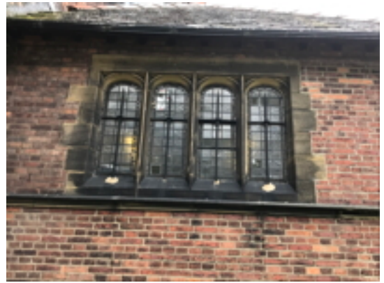
Vestry North Elevation Window
