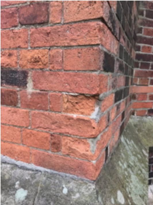
Erosion of brick faces to buttress
