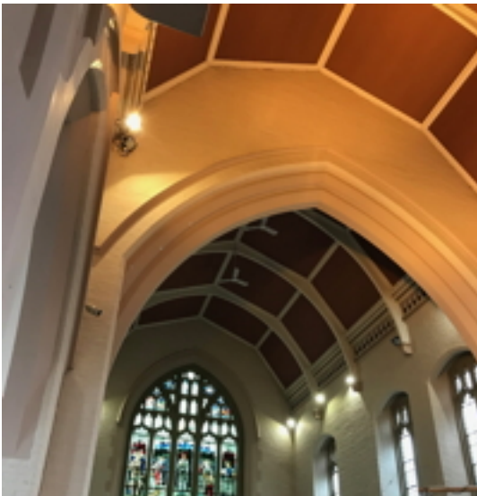
East End Ceiling
