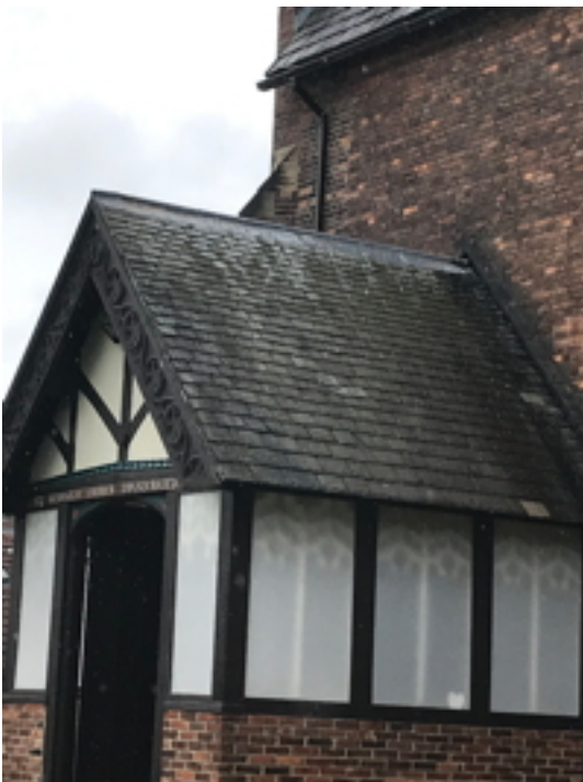
Slipped slate to Porch Roof
