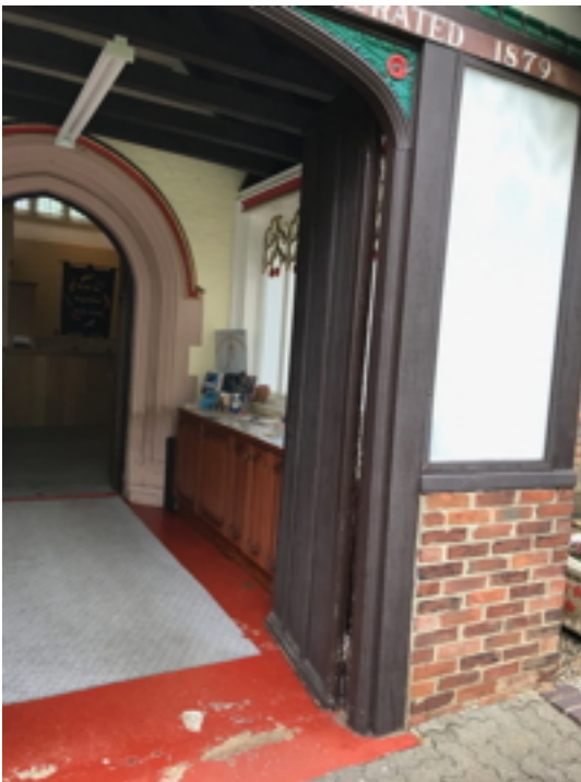
South Porch Doors
