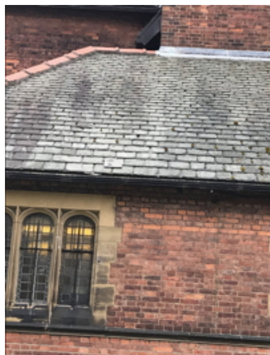
Slipped slate to Vestry Roof
