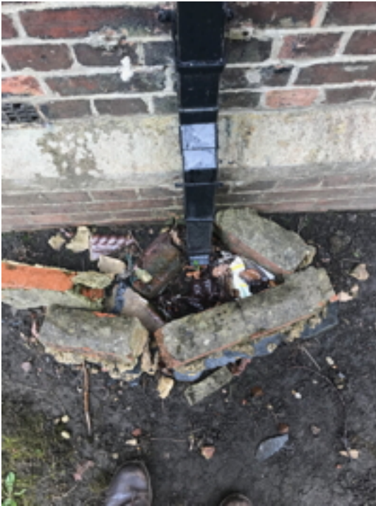
Damaged and Blocked Gully
