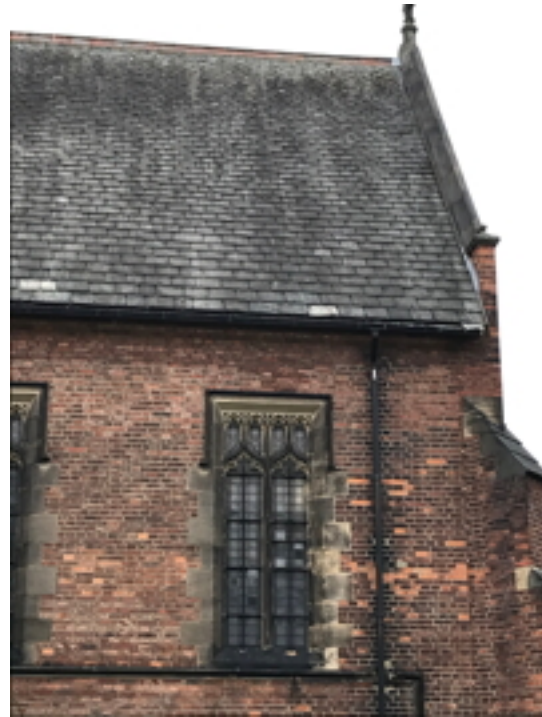
North Elevation West End with
