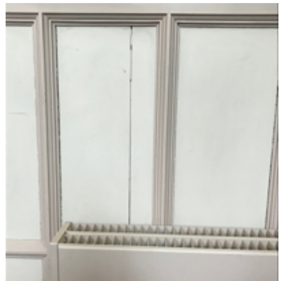
Typical Shrinkage Cracking to Panelling
