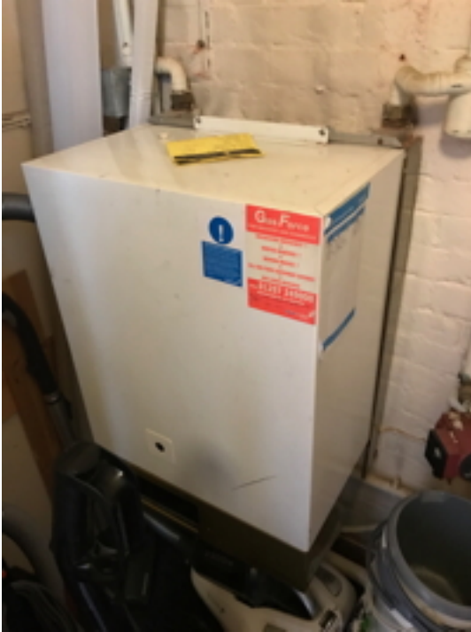
First Floor Boiler Room
