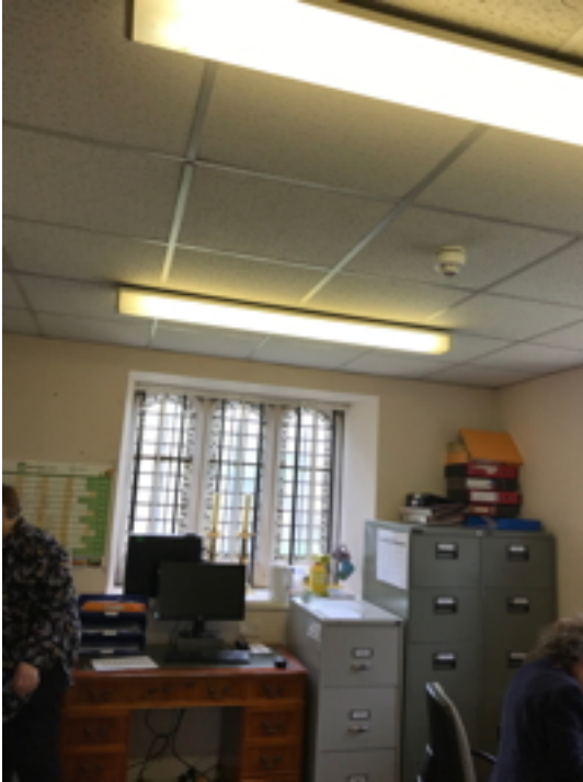
Vestry North Wall
