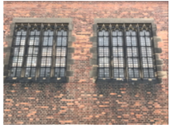
North Wall West End Windows
