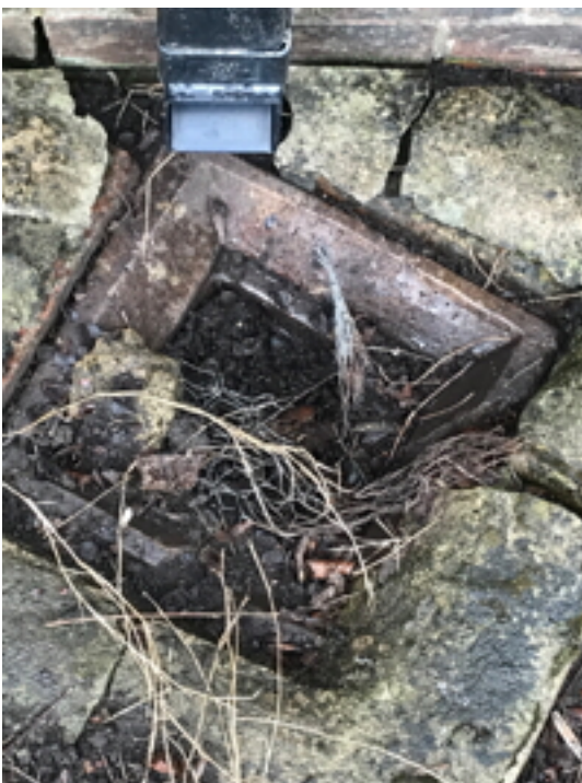
Damaged and Blocked Gully
