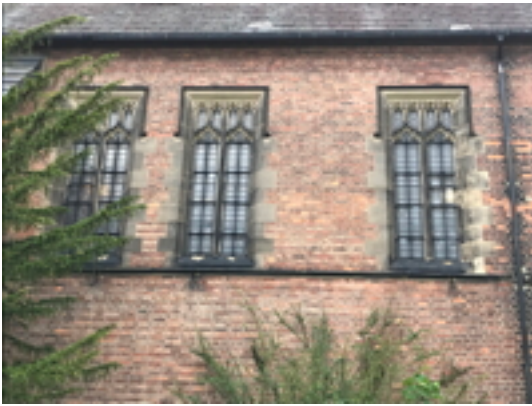
South Elevation East End Windows
