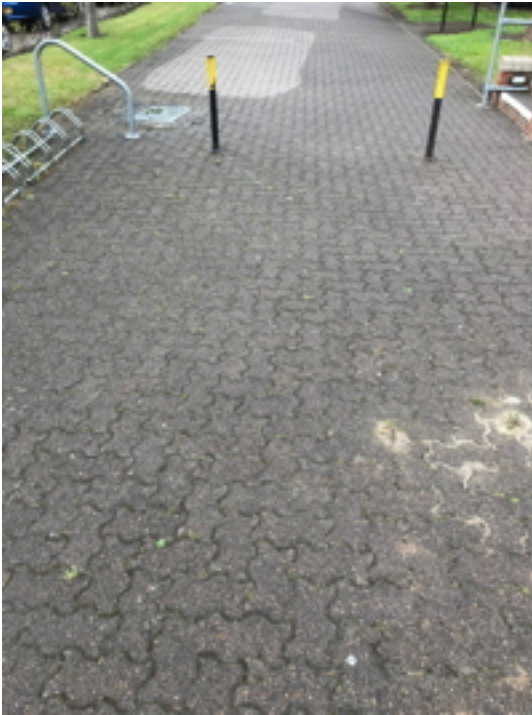
West Elevation Driveway
