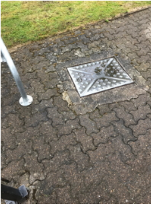
Inspection Chamber West End
