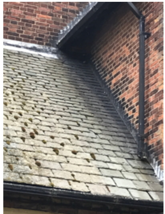
Rainwater Pipe discharging over Vestry Roof
