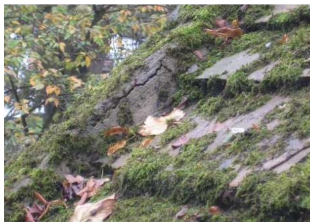
cracked fillet at SE porch (para 24)
