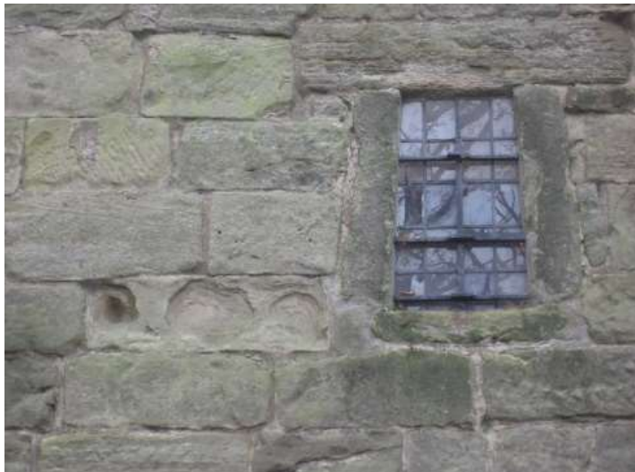
typical N nave
