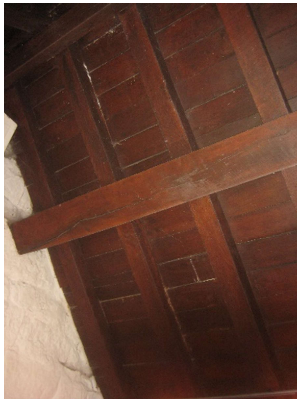
Porch E side
