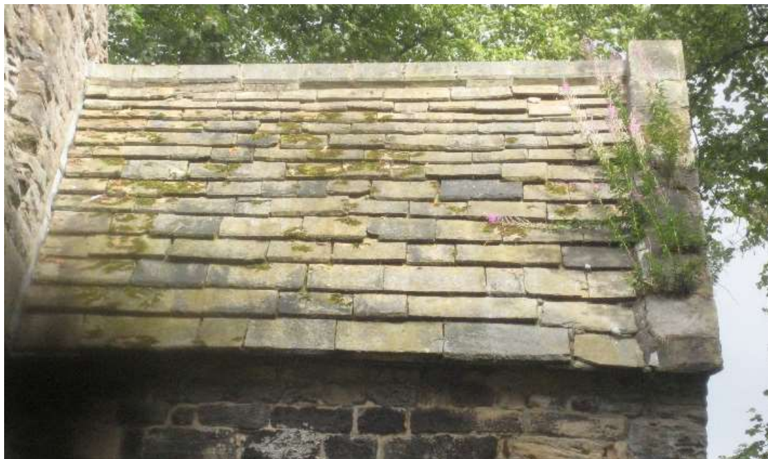
S Chancel, plants in cracked fillets and watertable joints and wedged slate at top right
