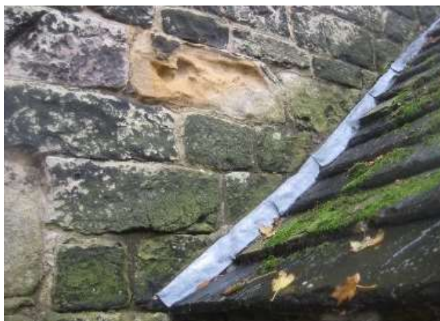
torn cover flashings against nave and decayed nave stone
