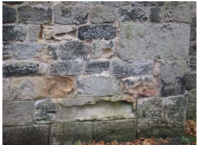
S nave bottom E corner, corresponding to damp inside
