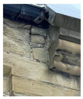
South elevation east end open joints
