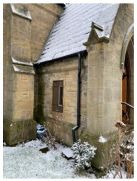
Porch West Elevation gutter misaligned
