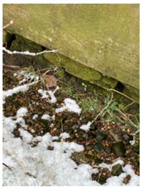
Low level ground erosion with open joints
