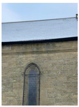
Chancel South Elevation gutter misaligned
