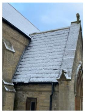
Porch West Roofs with slipped slates at eaves and ridge
