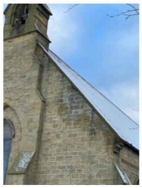
Nave west elevation south side gap in copings and damp stonework below
