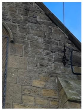
Chancel east elevation north side open joints
