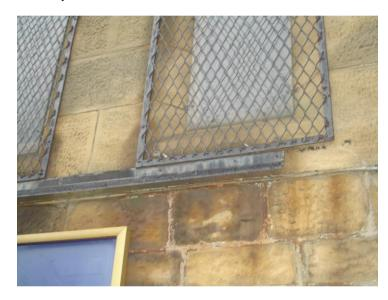
As the polycarbonate provides any necessary protection, it is recommended that consideration be given to removing the grillage to both negate further rust staining and improve the external visual quality of the building.
