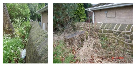
Part of the north-west boundary was appears to be acting as a retention wall to a domestic garage at higher level. The wall is deteriorating at its lower level, and due to the imposed loading from the garage and retained substructure, there is potential for structural failure, with the resultant partial collapse of the supported garage.
