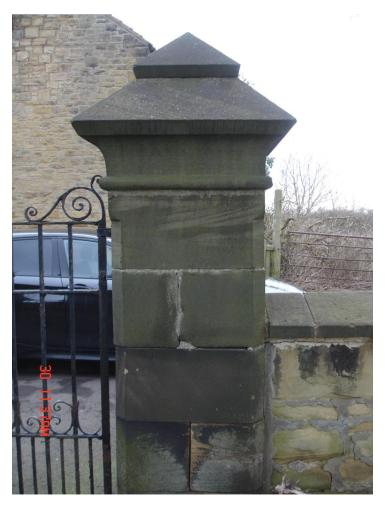
All three sets of original wrought iron gates are in need of urgent maintenance, with serious rust jacking in evidence, which requires careful cleaning, preparation and redecoration if the safe and efficient life of these gates are to be maintained. This applies to both the gates proper and the pillars or posts.
