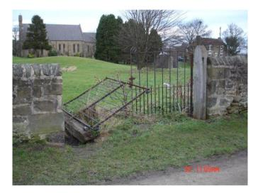
Localised rebuilding, indent repair and repointing to the boundary wall stonework is required.
