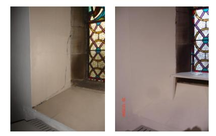
An historic movement crack to the south wall window jamb does not appear to have deteriorated since the previous report, and has been infilled as part of the recent redecoration works as indicated above:
