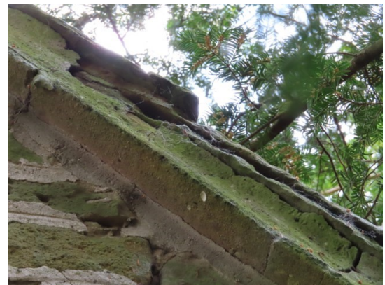
Deteriorating mortar to Western verge
