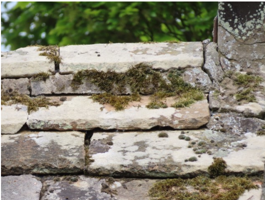
Cracked mortar around Nave cross which appears to be poorly secured
