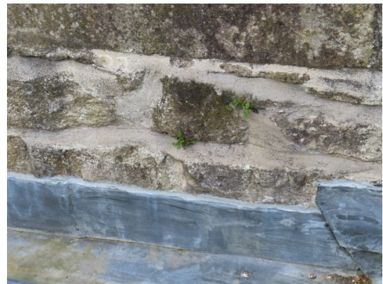
Failed and missing mastic above new Tower roof flashings with vegetation growth to the parapet (top right)
