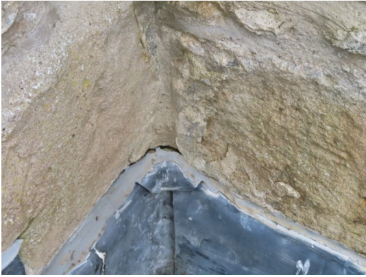
Failed and missing mastic above new Tower roof flashings
