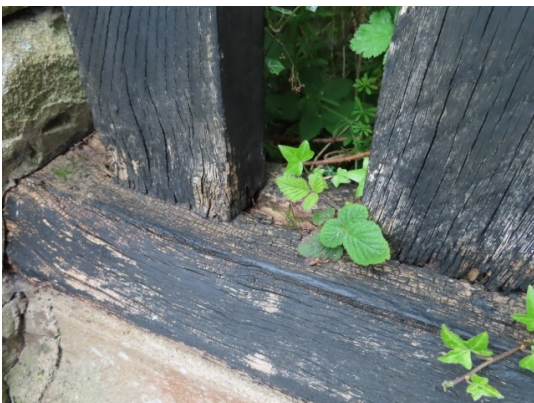
Rotten timber to Lych gate and cracking to stone plinth
