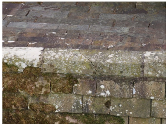
Cracked Nave ridge tile
