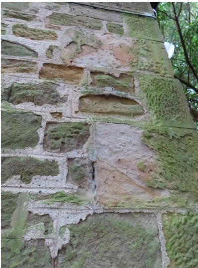
Weathered stone and failing mortar to the West elevation of the Nave (above and below)
