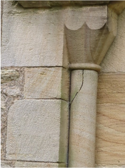
Cracked Pilaster to Chancel
