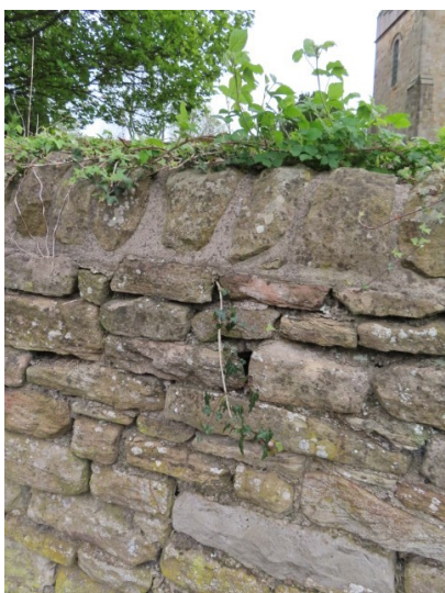
Ivy growth, loss of pointing and bowing around trees to boundary walls
