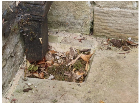
Debris filling Southern gully
