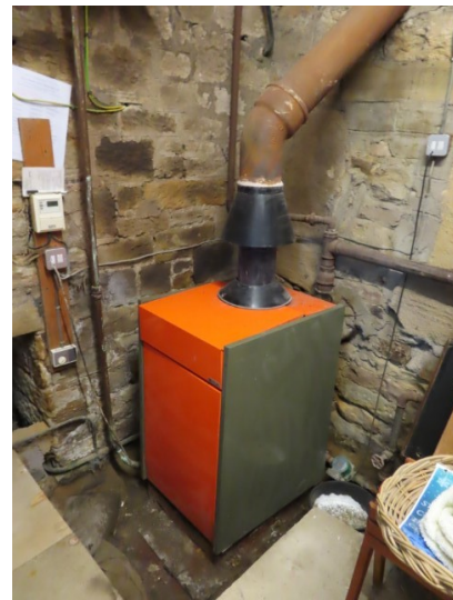
Rusty flue to boiler
