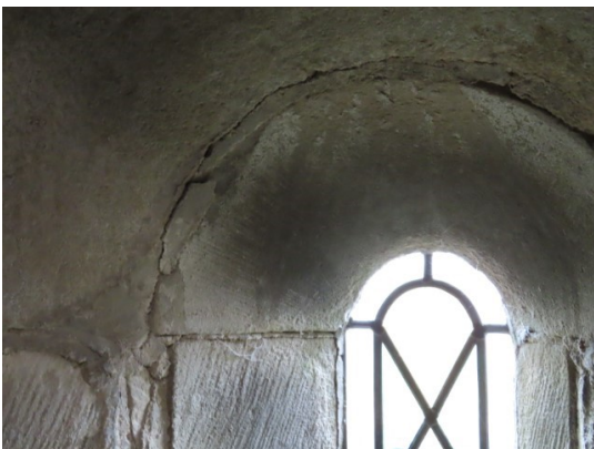
Cracking around nave window
