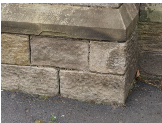
Deterioration of tower plinth stonework (North)
