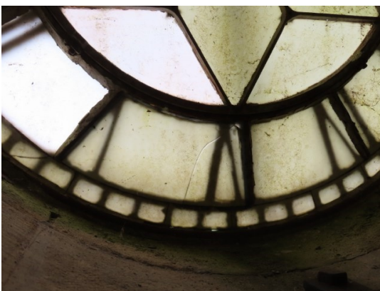
Cracked glazing and daylight visible to clock faces
