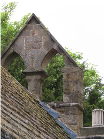
Open joints to Bellcote
