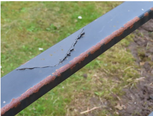
Failing paint to railing to main path
