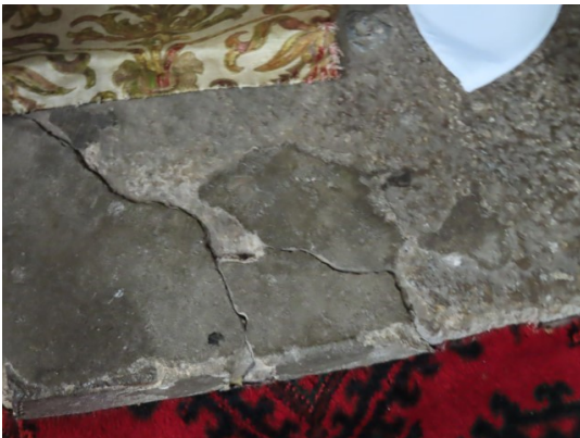
Failure to edge of altar dais
