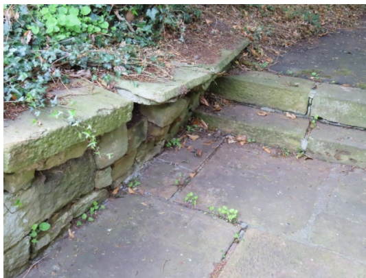
Bowing wall to the South of the Church
