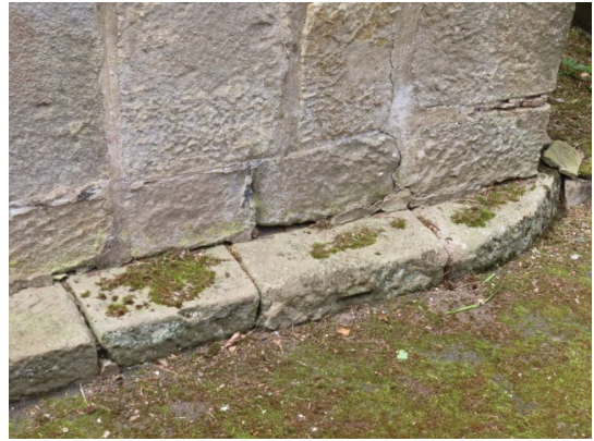
Open joints to the base of the Chancel wall
