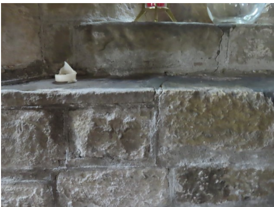
Cracking and hard mortar repairs to various Chancel Windows
