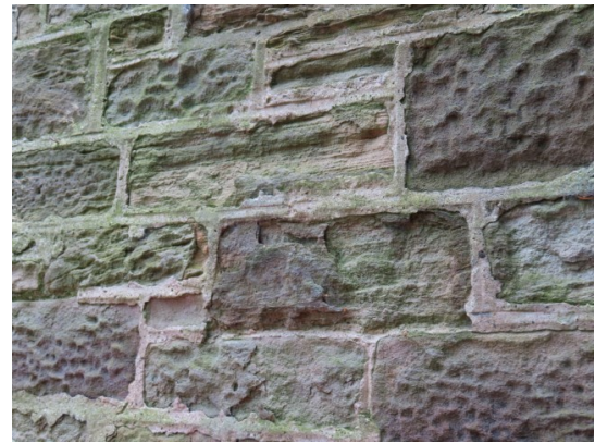
Weathered stone and failing mortar to the West elevation of the Nave (above and below)
