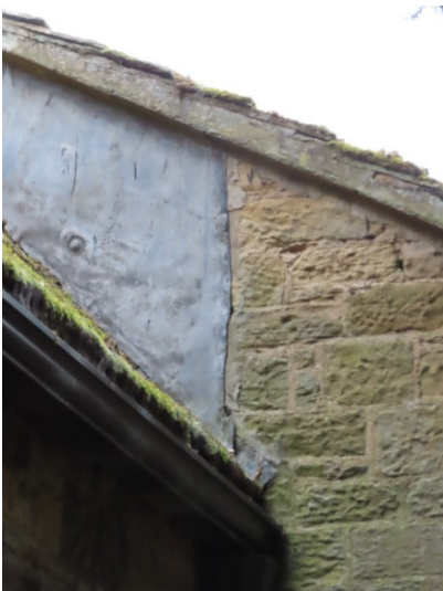
Mortar to edge of lead panels is failing in places
