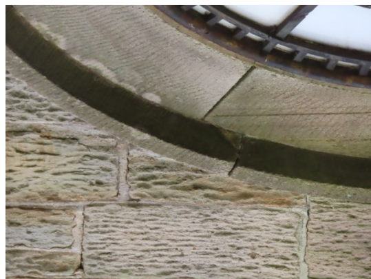
Deterioration of tower plinth stonework (North)
