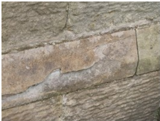
Deterioration of tower plinth stonework (North)
