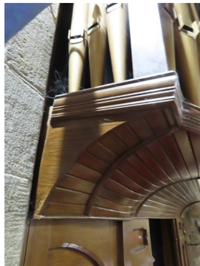
Organ frontal pulling away from the wall
