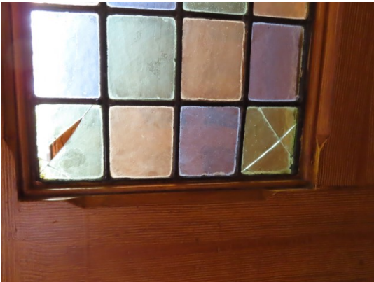
Cracked and missing glass to main internal doors of tower
