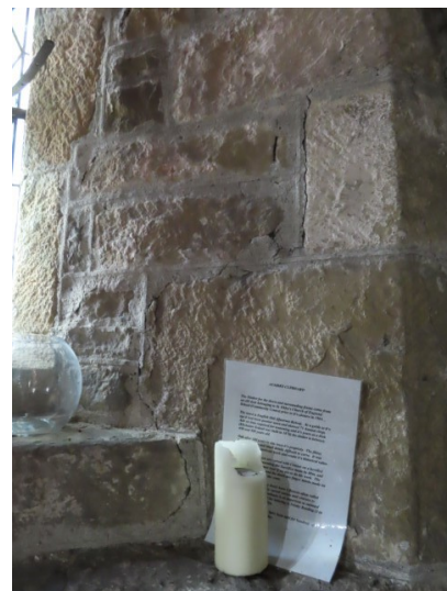
Cracking and hard mortar repairs to various Chancel Windows
