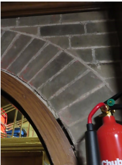
Cracking of mortar around door to organ chamber
