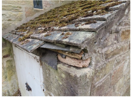
Damaged section of roof to boiler room lean to
