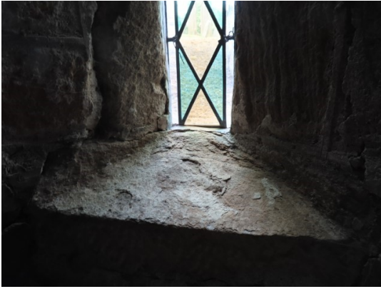
Cracking and hard mortar repairs to various Chancel Windows (above and below left)
