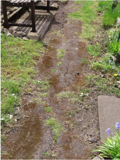
Cracked and raised path to main Garden of Remembrance bench. The Garden is generally rather overgrown
