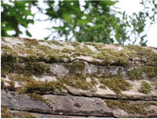
Moss growth and cracked mortar to bedding of ridge
