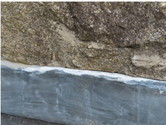
Failed and missing mastic above new Tower roof flashings with vegetation growth to the parapet (top right)
