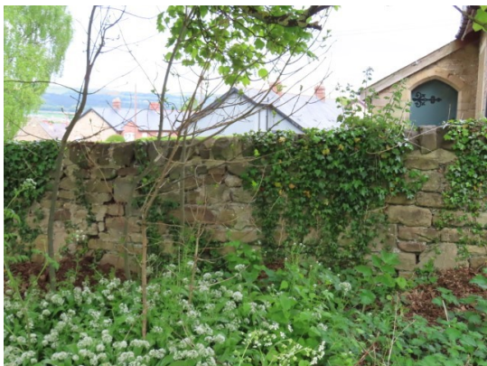
Ivy growth and cracking to the boundary wall
