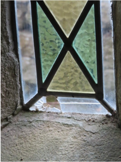
Damage to South Choir Vestry window
