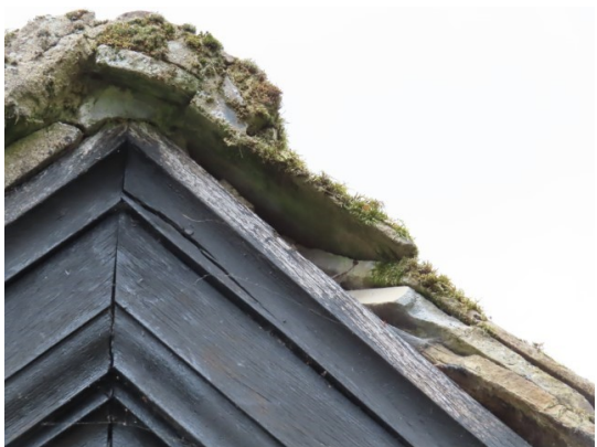
Failing mortar to Lych gate verge
