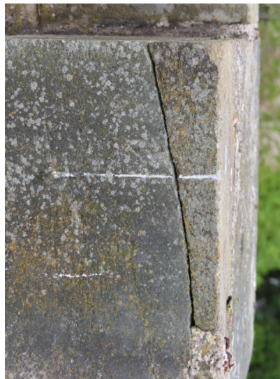
Crack to parapet stonework
