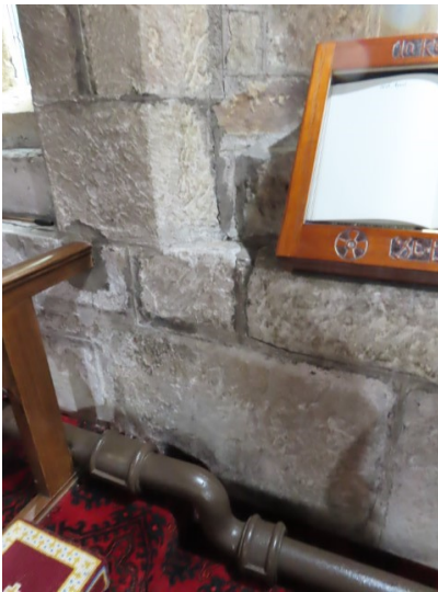
Cracking and hard mortar repairs to various Chancel Windows (above and below left)
