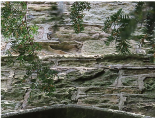
Weathered stone and failing mortar to the West elevation of the Nave (above and below)
