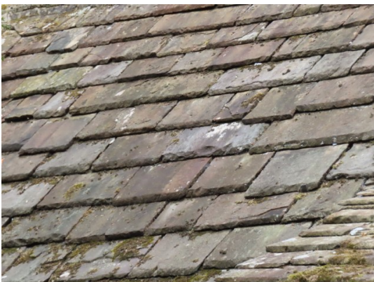
Slipped and damaged slates to the Southern roof slopes
