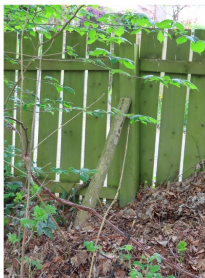
Propped fence post to Eastern side of the churchyard
