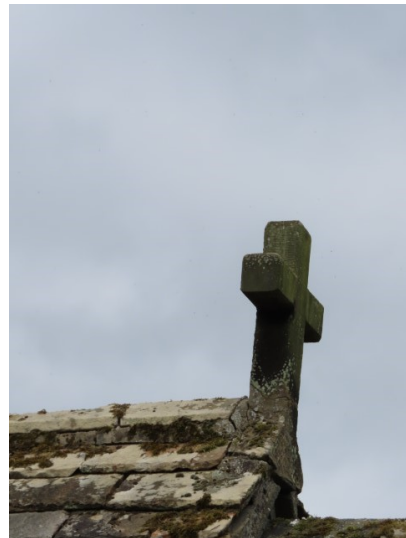
Cracked mortar around Nave cross which appears to be poorly secured
