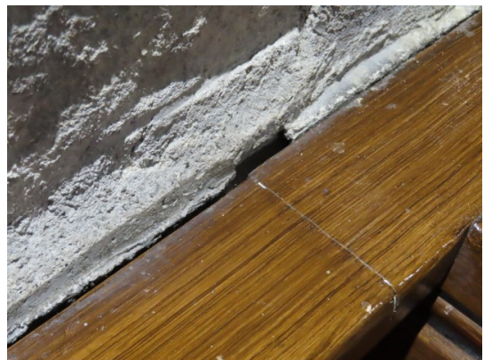
Fill behind pew edging is failing
