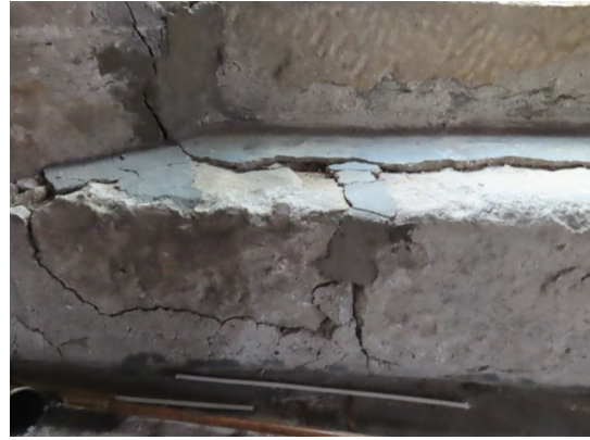
Cracking and hard mortar repairs to various Chancel Windows (above and below left)
