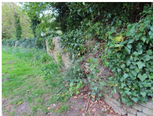
Ivy growth, loss of pointing and bowing around trees to boundary walls
