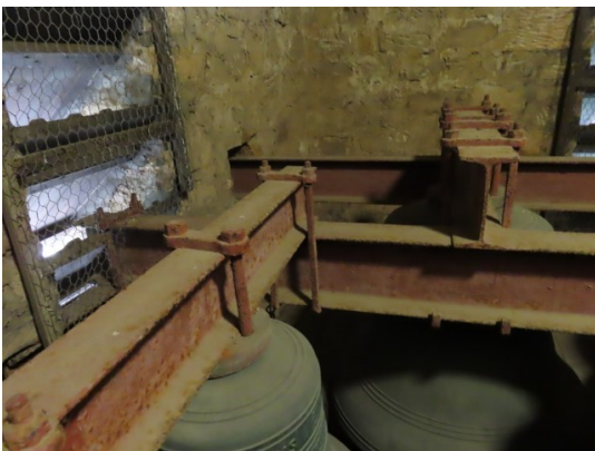
Rusting headstock and beams supporting the bells
