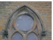
Central rose window, hoodmould looks ok, some wear on the northern side of the inner reveal. The radiating trefoil tracery looks ok. The inner ring has a chip out of it at the one o'clock position and I wonder if the tracery might be a little poor, there has been some shouldering in cement in the past so it has seen some repair. It is probably the dowel joint that has rusted and broke the inner circle.
