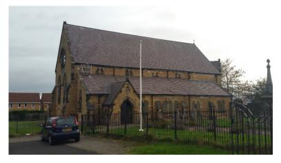
**South side** – Angled terracotta ridges bedded ok, some chipped slates one probably losing its fixing, there has been some repairs in none-matching towards the eastern end. W abutment is mortar flaunching to watertable not much upstand on the
