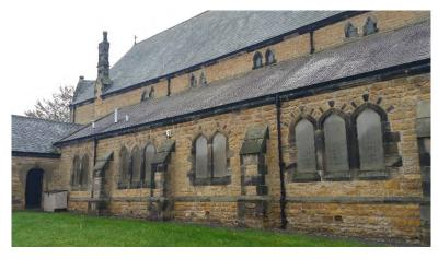
It is the same design as the S aisle except they have two triple windows here and the masonry ashlar surrounds are fine. The polycarbonate is looking rather grey. The eastern most window seems to be in an aluminium frame possibly to provide a ventilator which can't open because there is polycarbonate stopping it.
