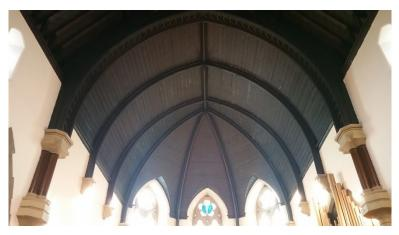
False ceiling of curved members down to corbels and all of these are ok, between the two is a chancel arch formed of boxed truss
